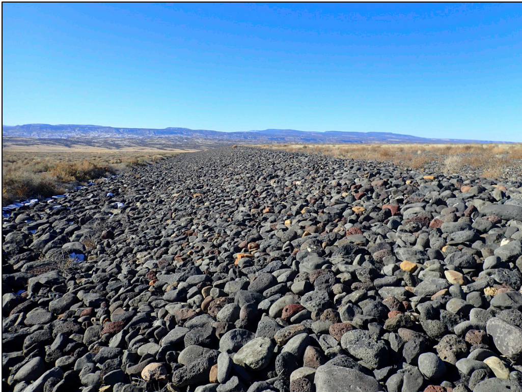
PL-8. Disposal Cell, South Side Slope
