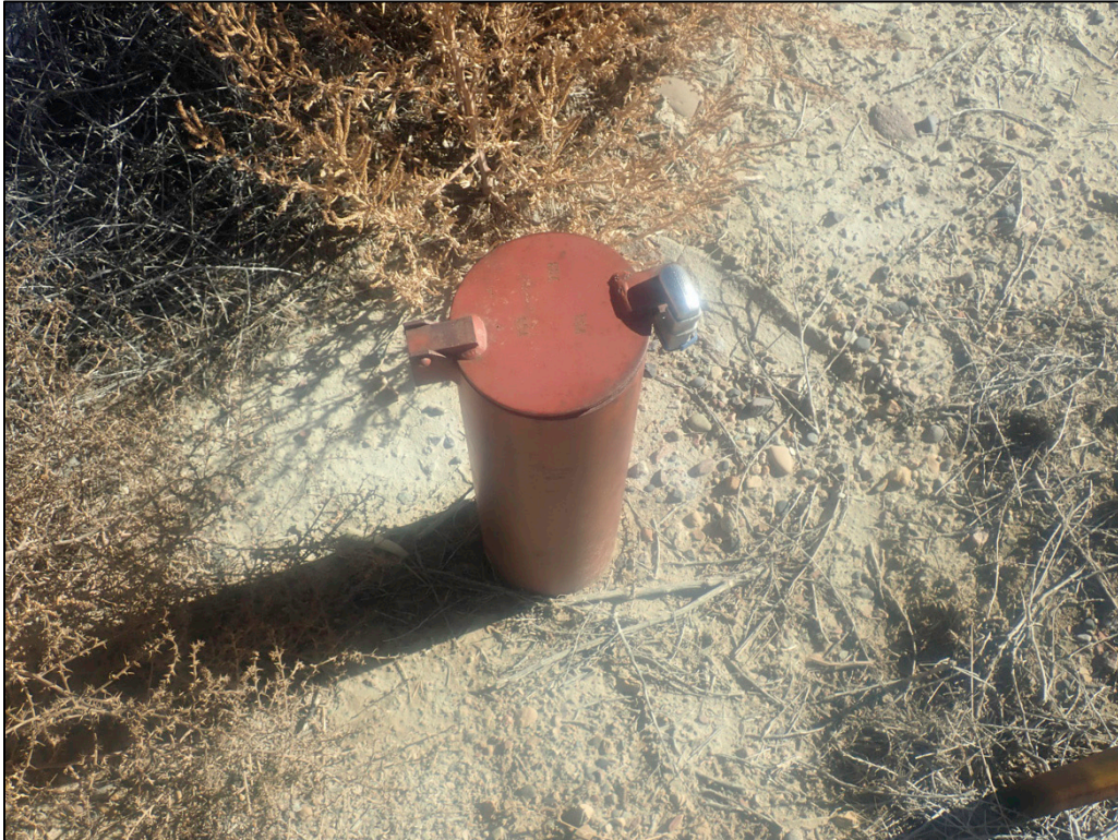
PL-7. Monitoring Well 0733
