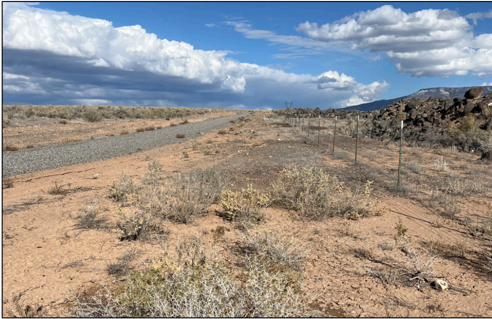
PL-1. Perimeter Fence
