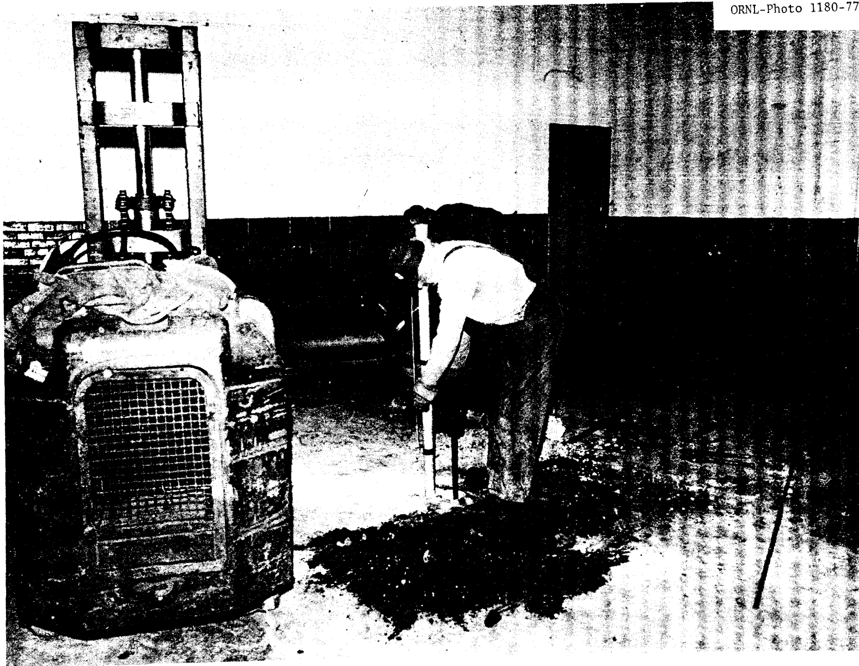
Fig. I-J. View southwest to northeast in old storage area in Building C, showing workmen at a core drilling site.
