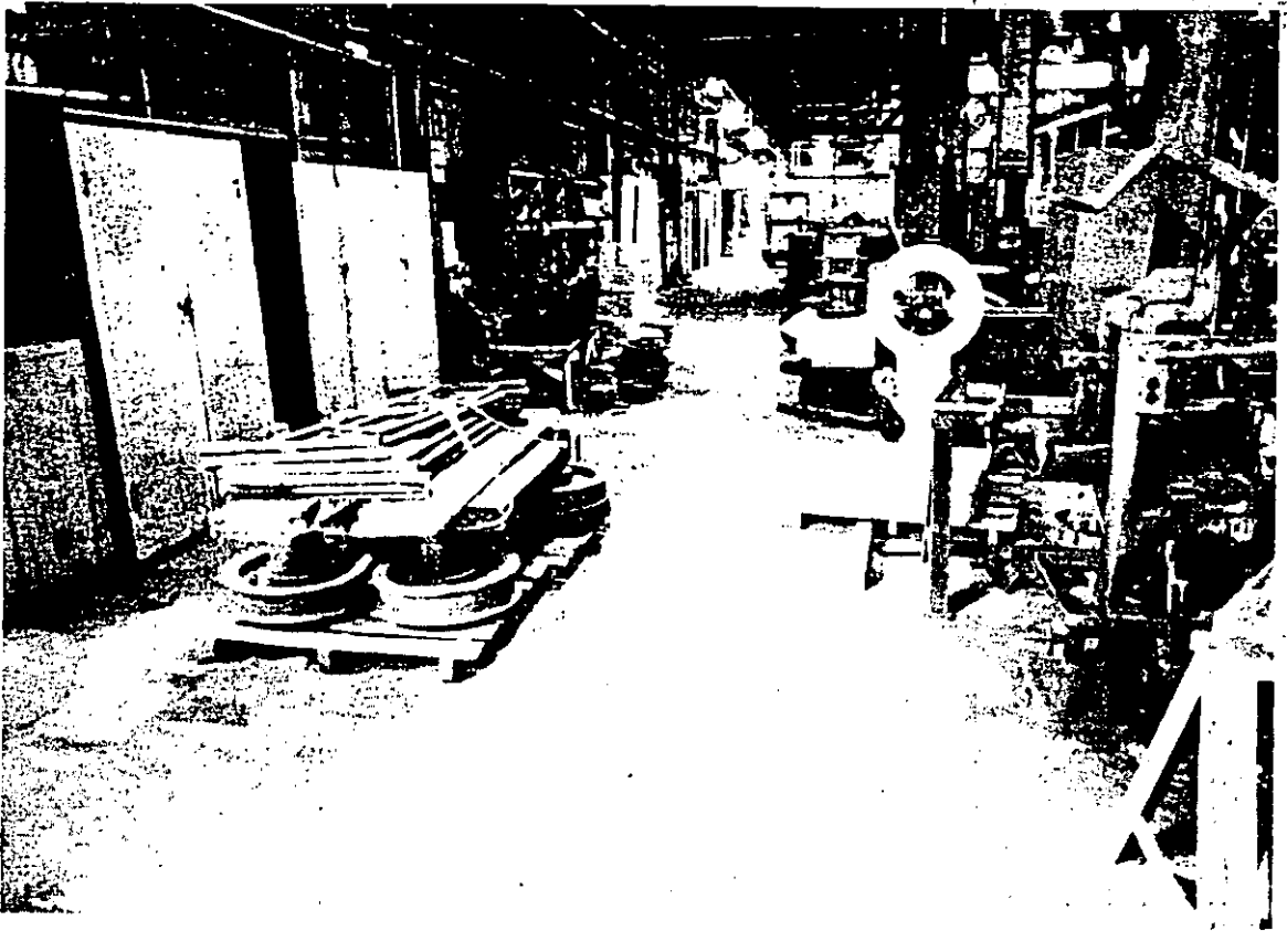
Fig. 9. Eastward view in building D of the rolling mill and storage area at Jessop Steel Company, 500 Green Street, Washington, Pennsylvania (JSP001).
