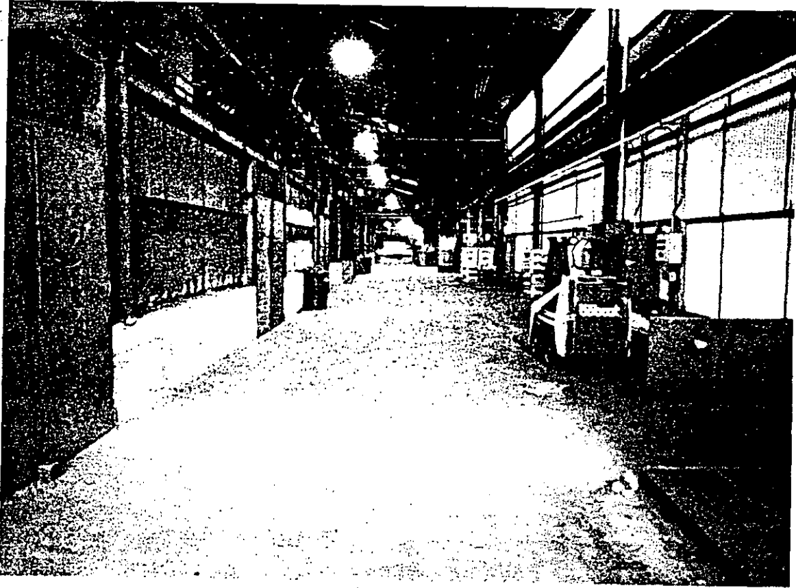
Fig. 10. Eastward view in building D of the SWARF bins at Jessop Steel Company, 500 Green Street, Washington, Pennsylvania (JSP001).
