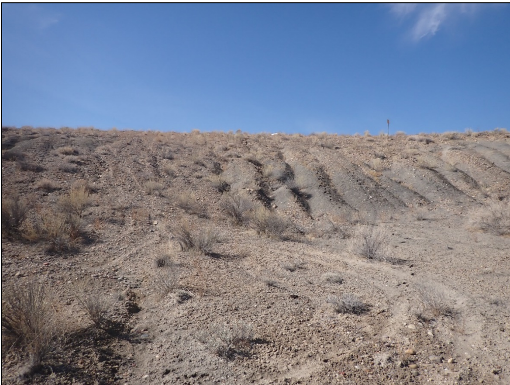
PL-12. Soil Erosion by Boundary Monument BM-7 (Offsite)
