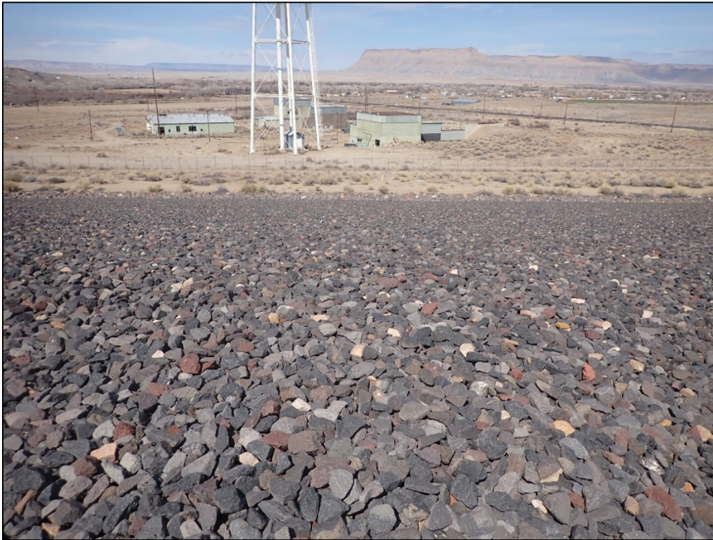
PL-9. Disposal Cell Northwest Side Slope
