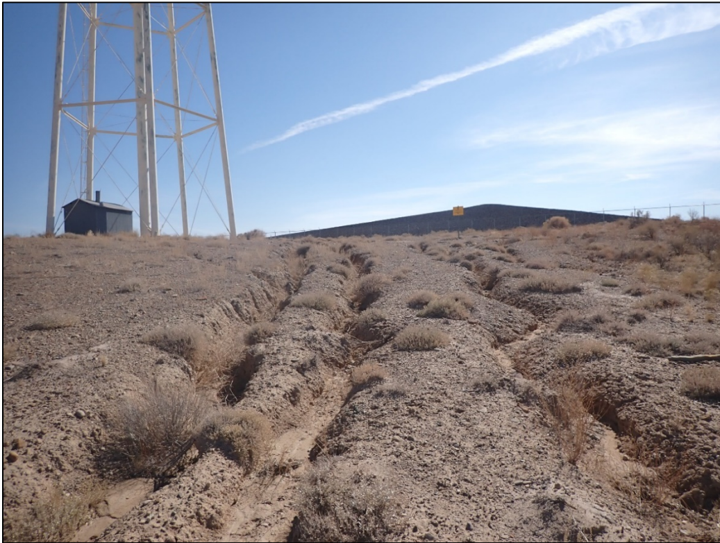
PL-15. Soil Erosion (Offsite)
