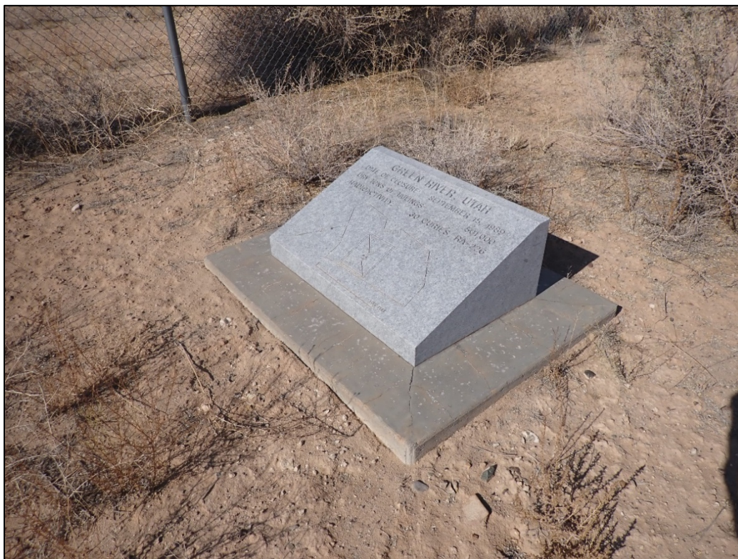
PL-4. Minor Cracks in the Base of Site Marker SMK-1
