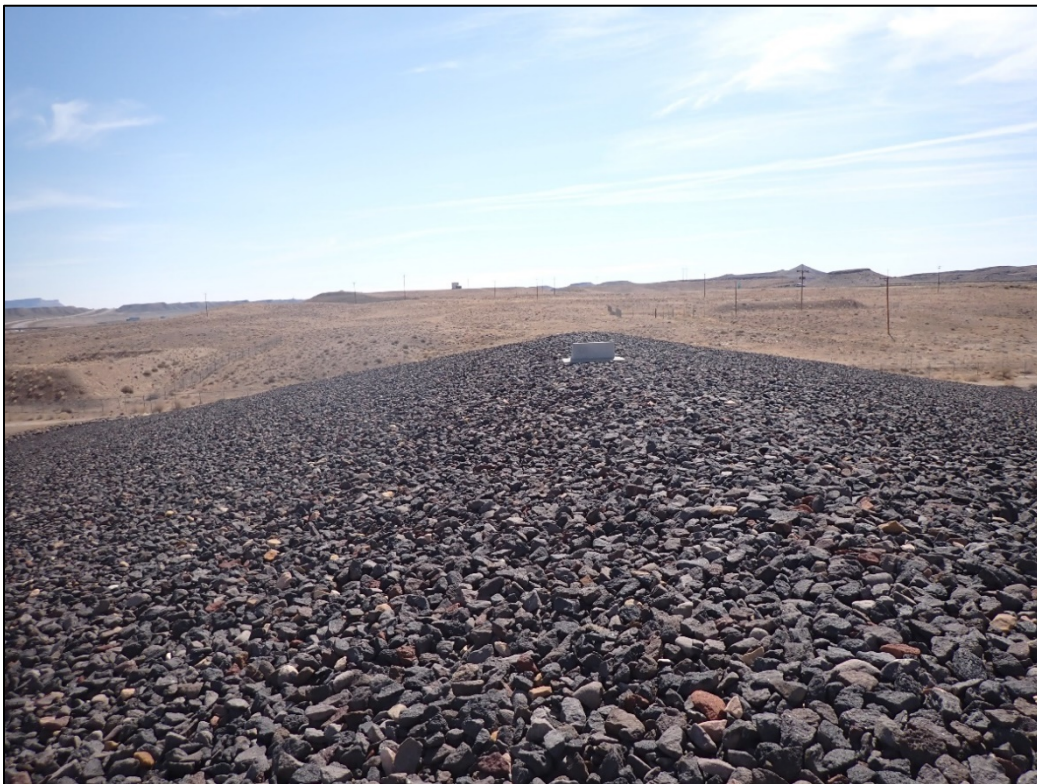
PL-8. Site Marker SMK-2 on Disposal Cell Top Slope
