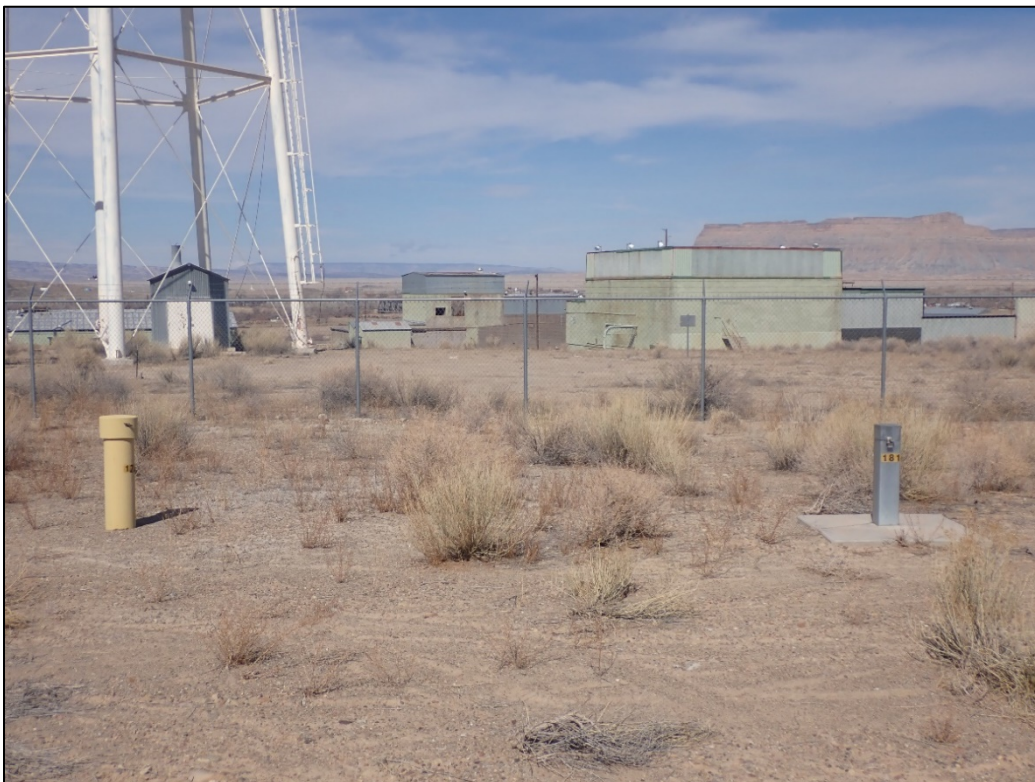
PL-14. Monitoring Wells 0172 and 0181 (Onsite) and Abandoned Mill Buildings (Offsite)
