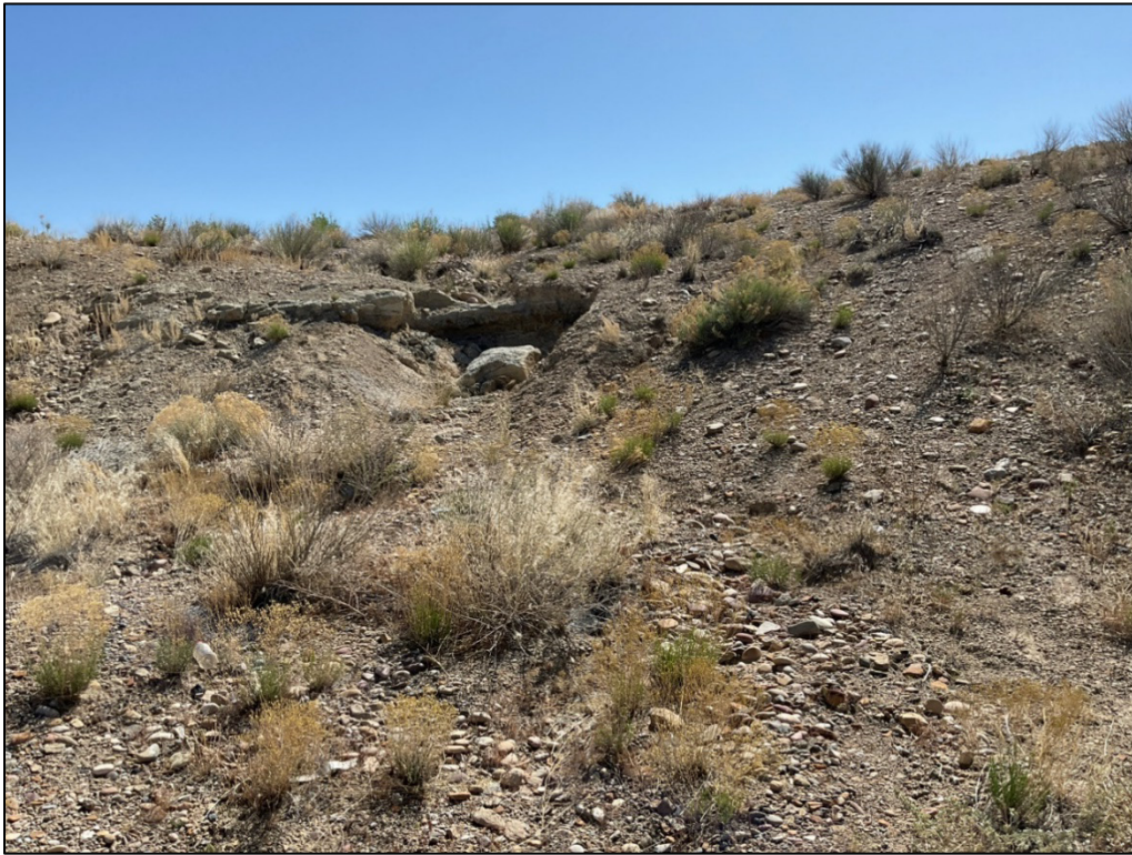
PL-7. Erosion near Perimeter Sign P7 and the Water Tower
