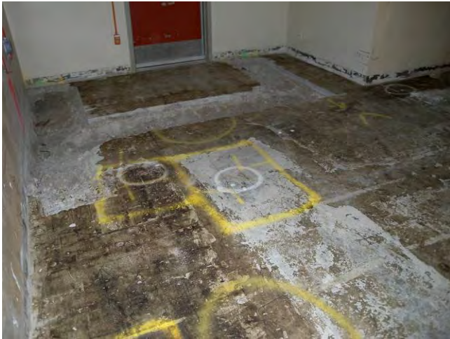
T Bldg. Room 61 View E
