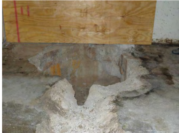
T Bldg. Room 16 View D
