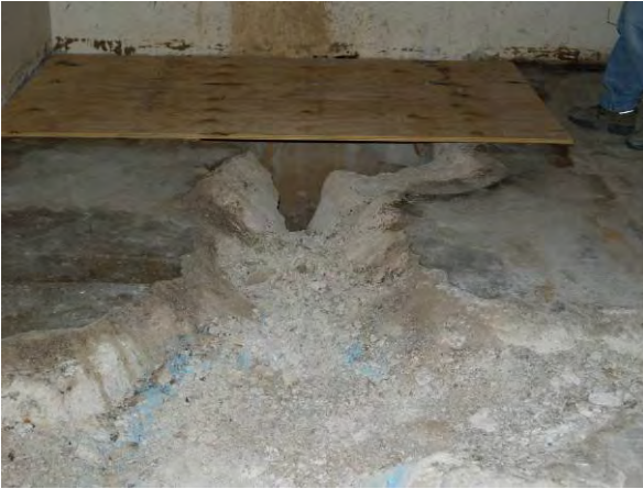
T Bldg. Room 16 View C
