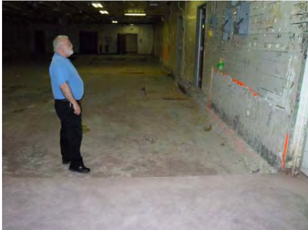
T Bldg. Rooms 39-44, 48-50 View B
