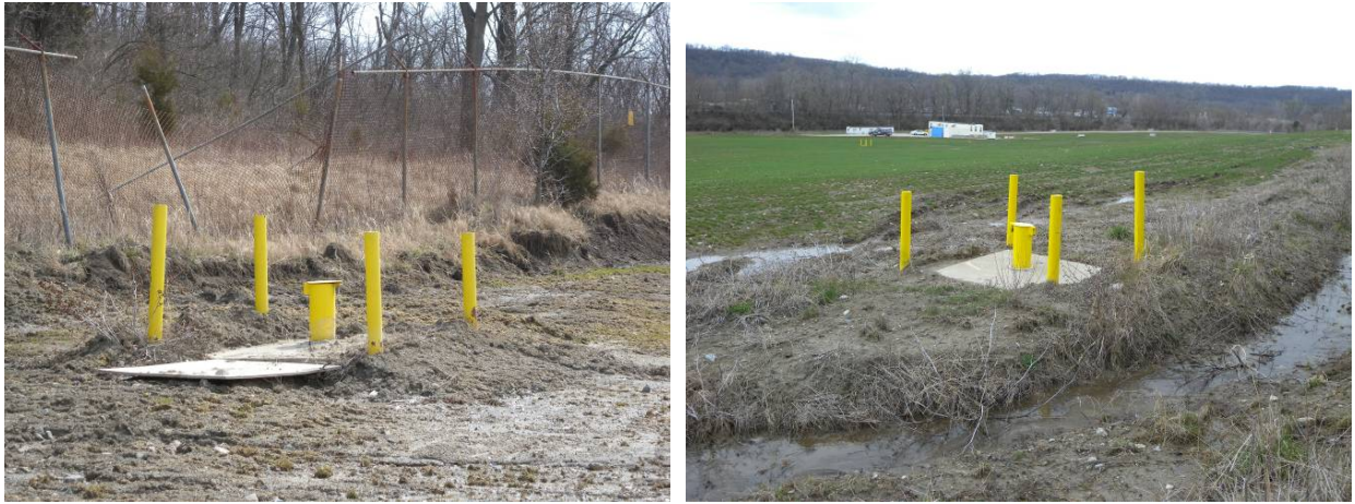
Figure 16. Well 0353 in 2009, with drainage problems, and in 2011, with water diverted away from well
