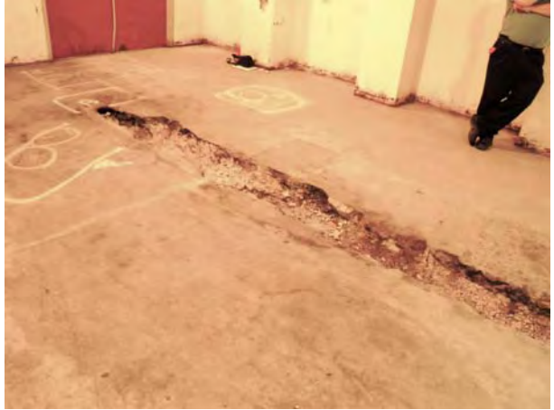
T Bldg. Room 16 View F
