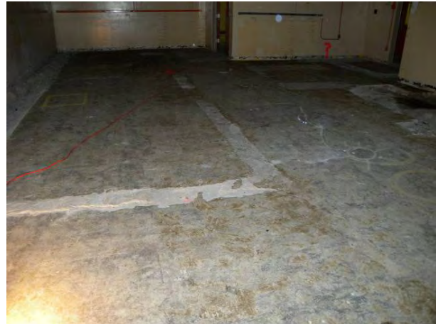
T Bldg. Room 61 View B
