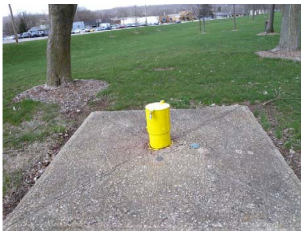
Figure 13. Well 0124 offsite condition during 2011 IC assessment
