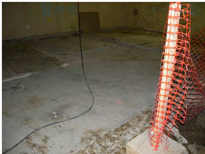
T Bldg. Room 63 View J
