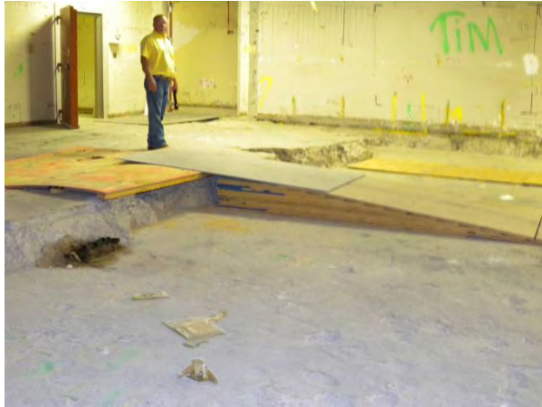
T Bldg. Rooms 39-44, 48-50 View E
