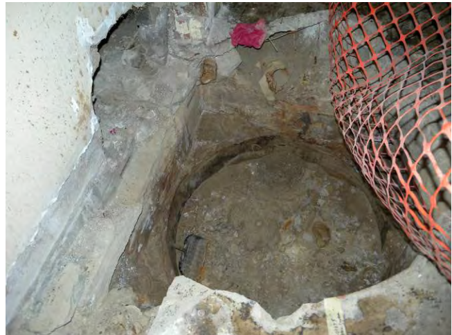
T Bldg. Room 63 View H
