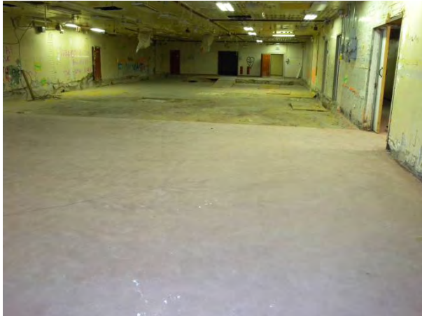
T Bldg. Rooms 39-44, 48-50 View A
