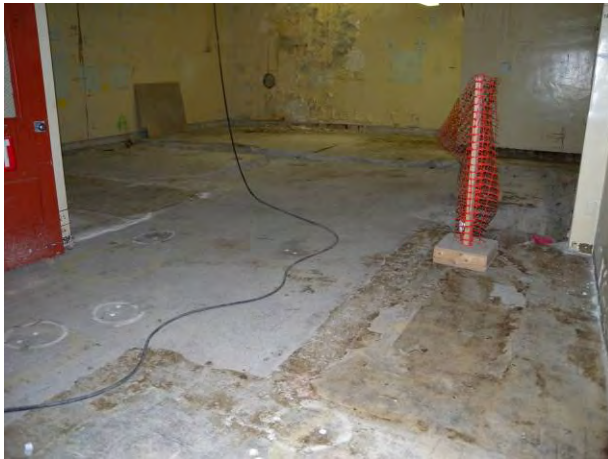
T Bldg. Room 63 View A
