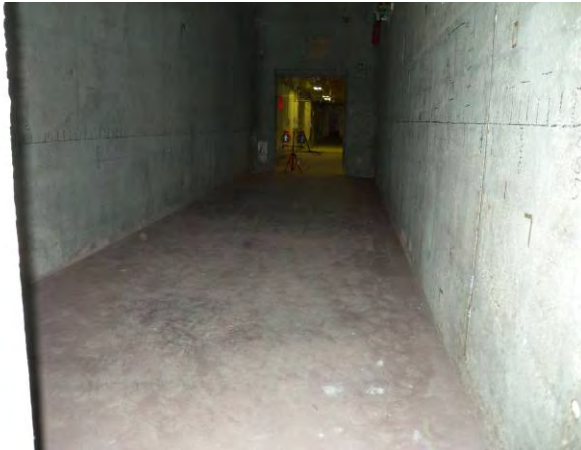
T Bldg. Room 59 View E
