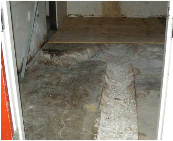
T Bldg. Room 16 View A
