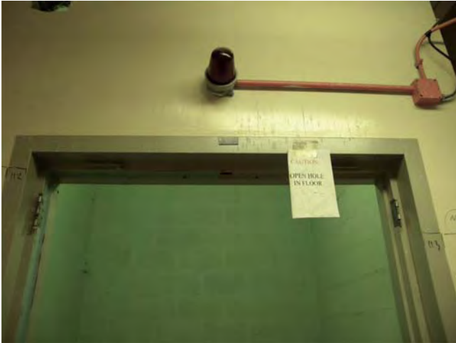
T Bldg. Room 62 View K
