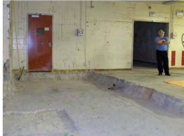
T Bldg. Rooms 39-44, 48-50 View F
