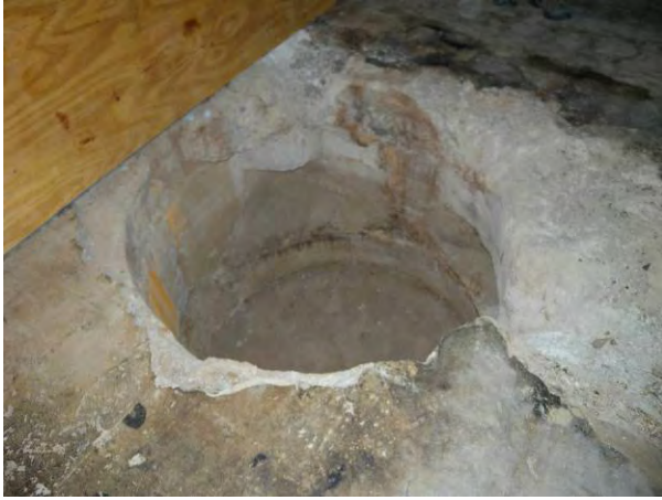
T Bldg. Room 16 View E
