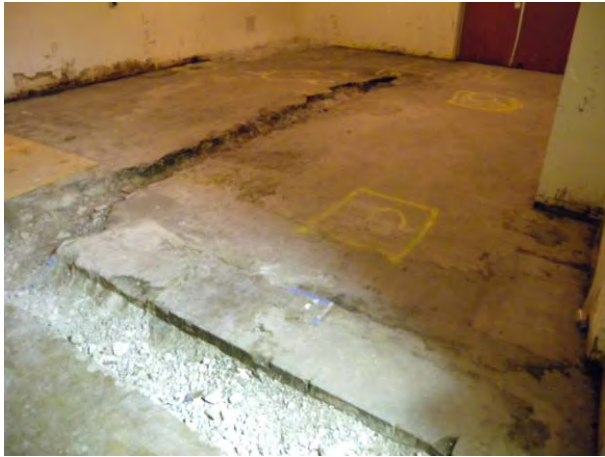
T Bldg. Room 16 View B
