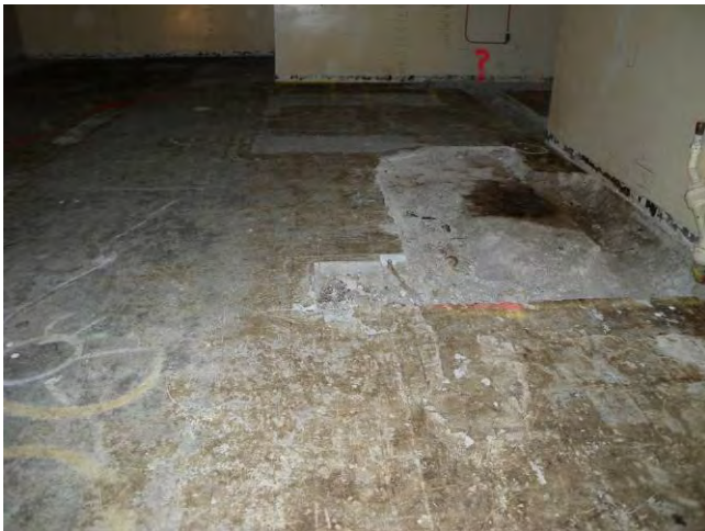
T Bldg. Room 61 View G
