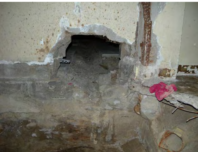
T Bldg. Room 63 View I
