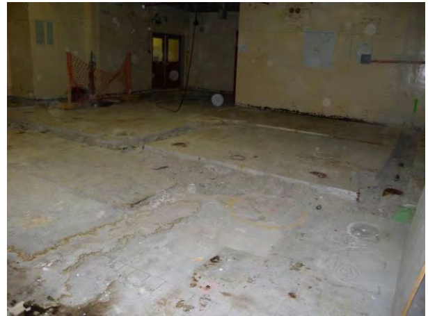
T Bldg. Room 63 View D
