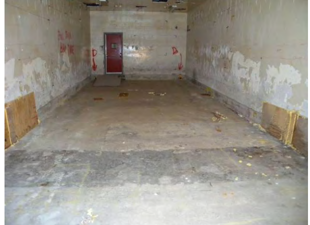
T Bldg. Room 58 View D
