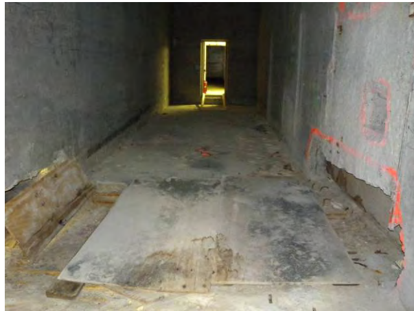
T Bldg. Room 57 View B
