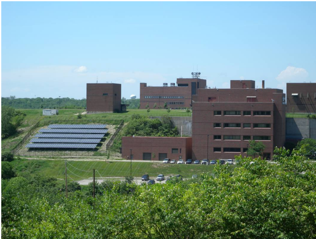
Figure 8. Solar array west of COS Building
