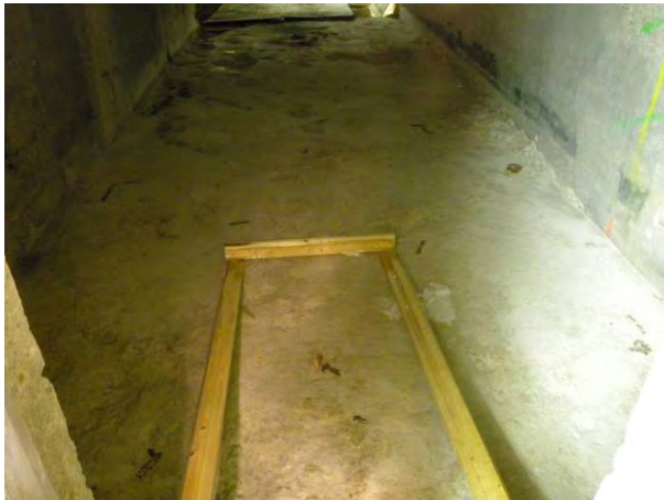
T Bldg. Room 57 View A
