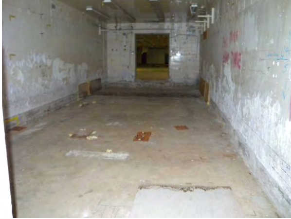
T Bldg. Room 58 View C
