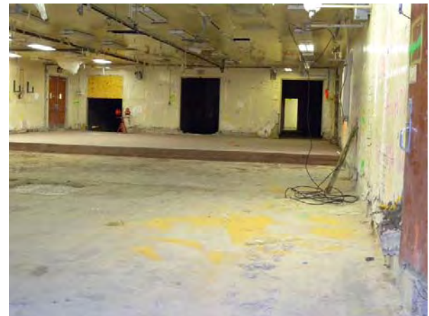
T Bldg. Rooms 39-44, 48-50 View J
