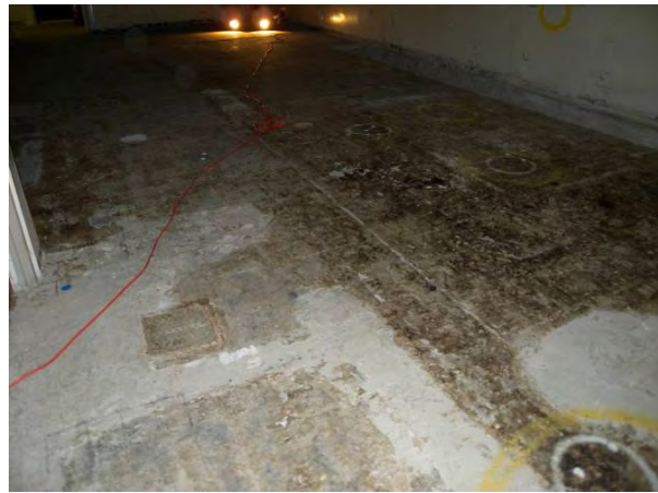
T Bldg. Room 61 View D
