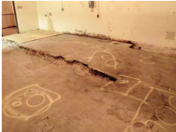
T Bldg. Room 16 View I
