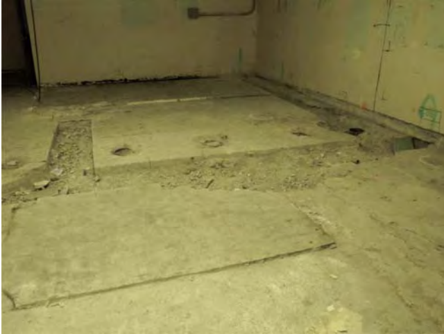
T Bldg. Room 63 View E
