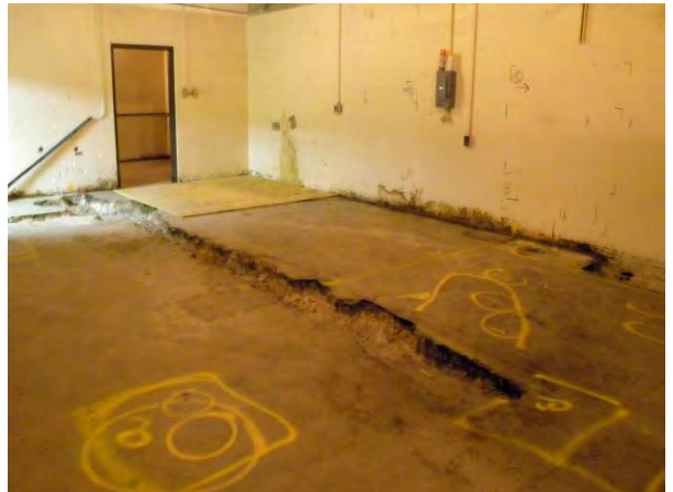
T Bldg. Room 16 View J
