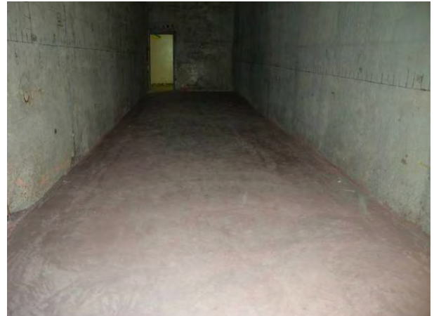
T Bldg. Room 59 View F
