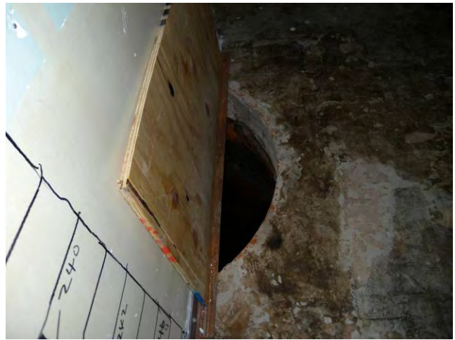
T Bldg. Room 61 View H
