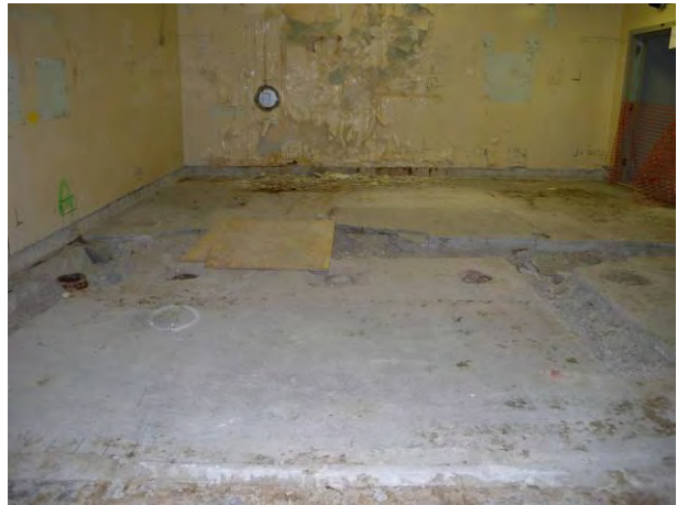
T Bldg. Room 63 View B
