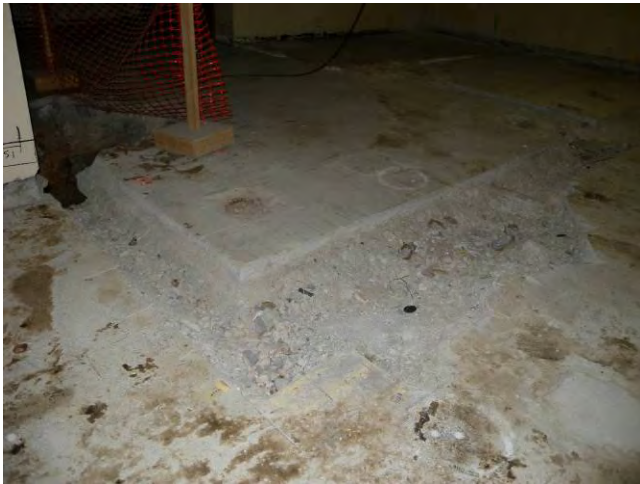
T Bldg. Room 63 View G
