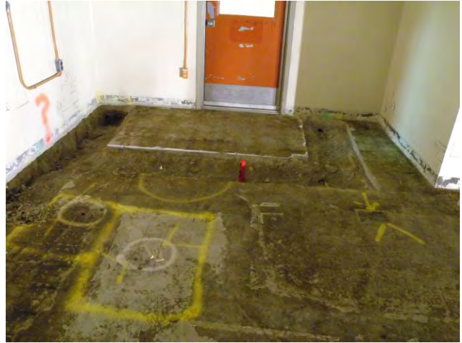
T Bldg. Room 61 View F
