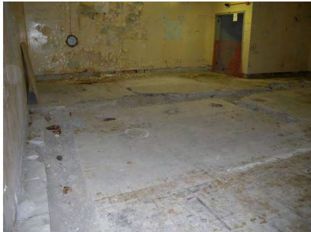
T Bldg. Room 63 View C
