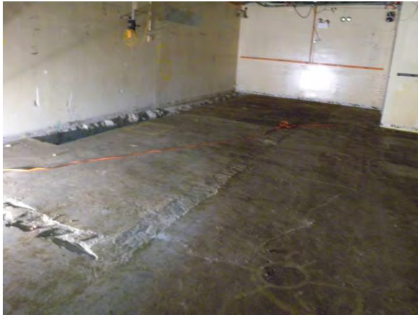
T Bldg. Room 61 View A
