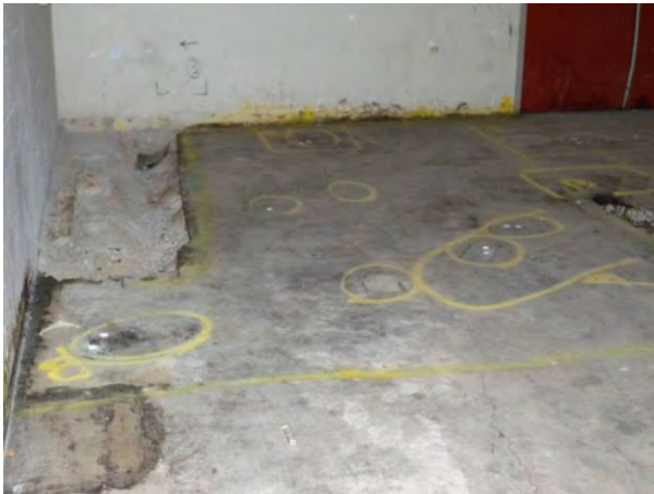
T Bldg. Room 16 View G
