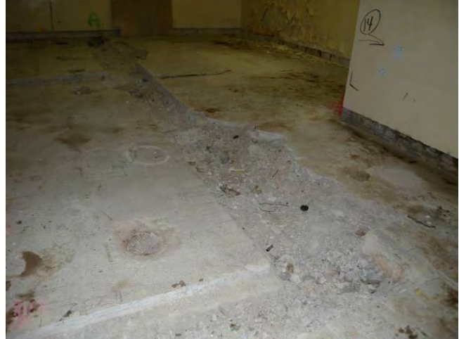
T Bldg. Room 63 View F
