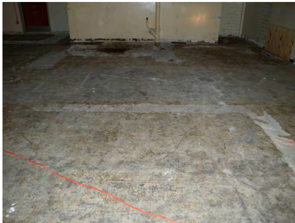
T Bldg. Room 61 View C
