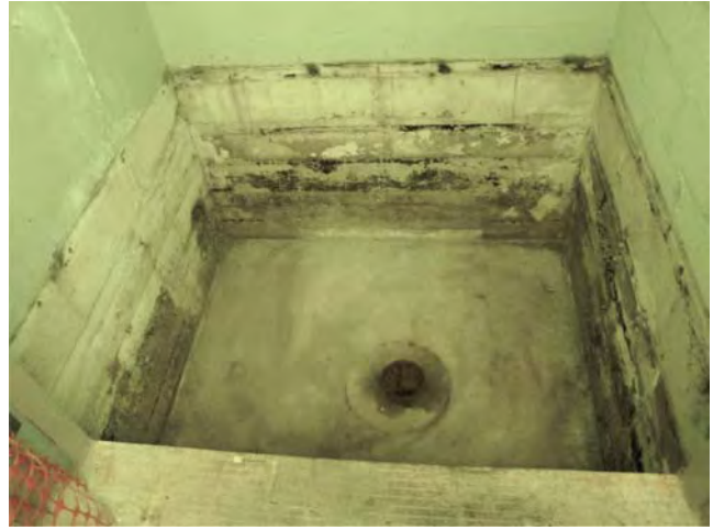
T Bldg. Room 62 View L
