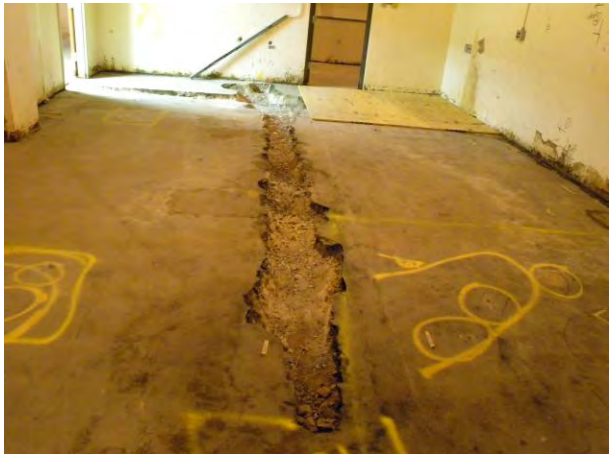
T Bldg. Room 16 View H
