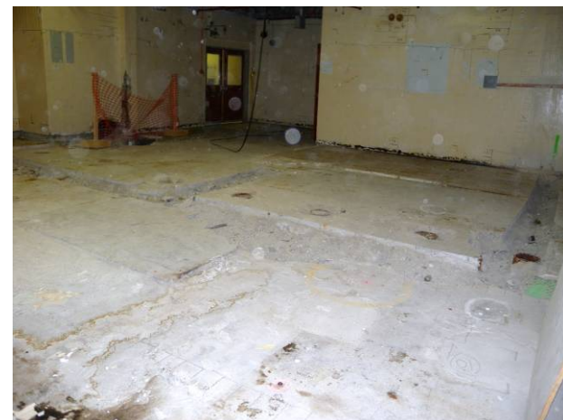
Figure C-23. T Bldg. Room 63 View D
