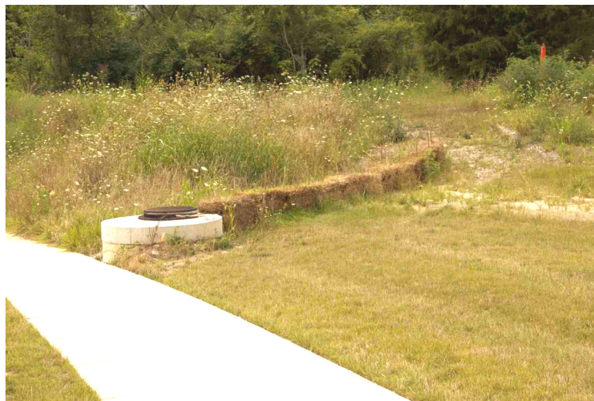
Figure 13. Erosion-Control Barrier North of OU-1 West of Vanguard Blvd.
