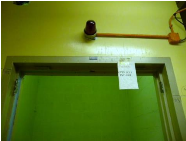
Figure C-30. T Bldg. Room 62 View K
