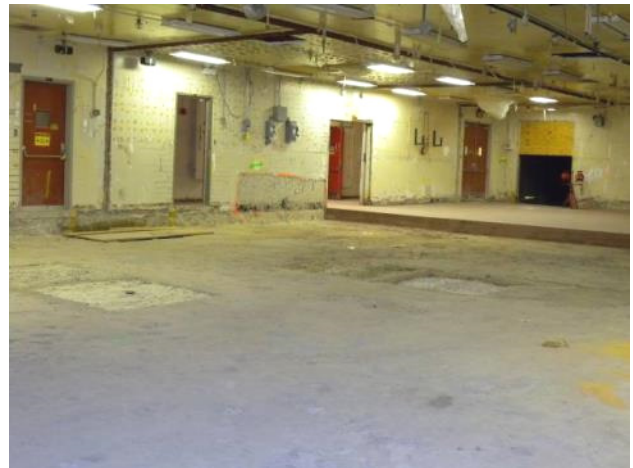
Figure C-45. T Bldg. Rooms 39-44 and 48-50 View H
