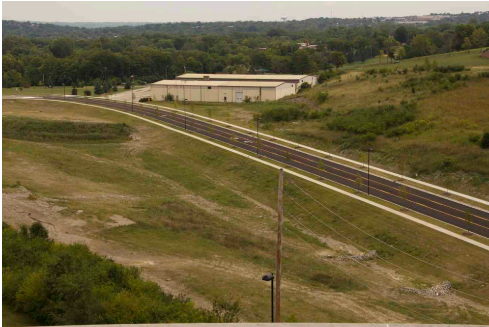
Figure 10. Vanguard Blvd. Looking Northeast Toward Building 61
