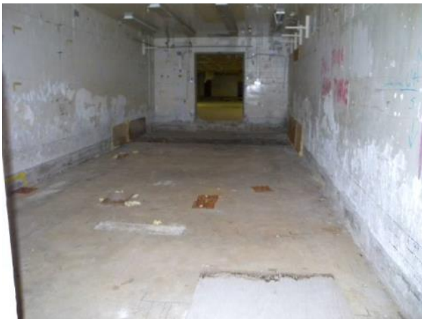
Figure C-34. T Bldg. Room 58 View C
