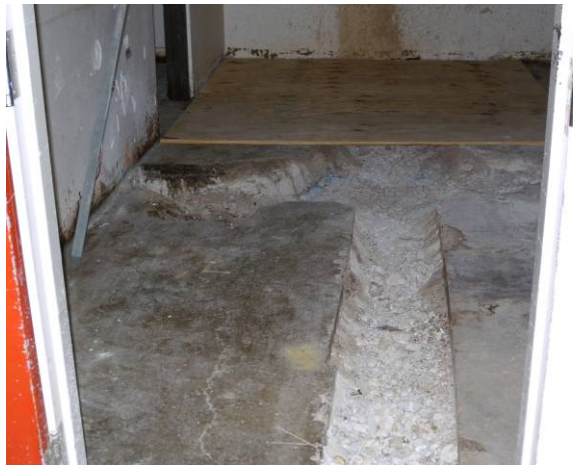
Figure C-2. T Bldg. Room 16 View A
