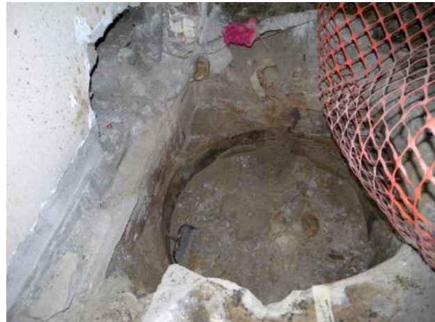
Figure C-27. T Bldg. Room 63 View H
