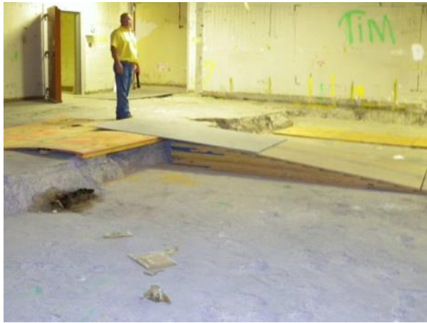
Figure C-42. T Bldg. Rooms 39-44 and 48-50 View E
