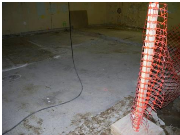
Figure C-29. T Bldg. Room 63 View J
