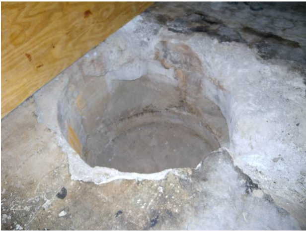
Figure C-6. T Bldg. Room 16 View E
