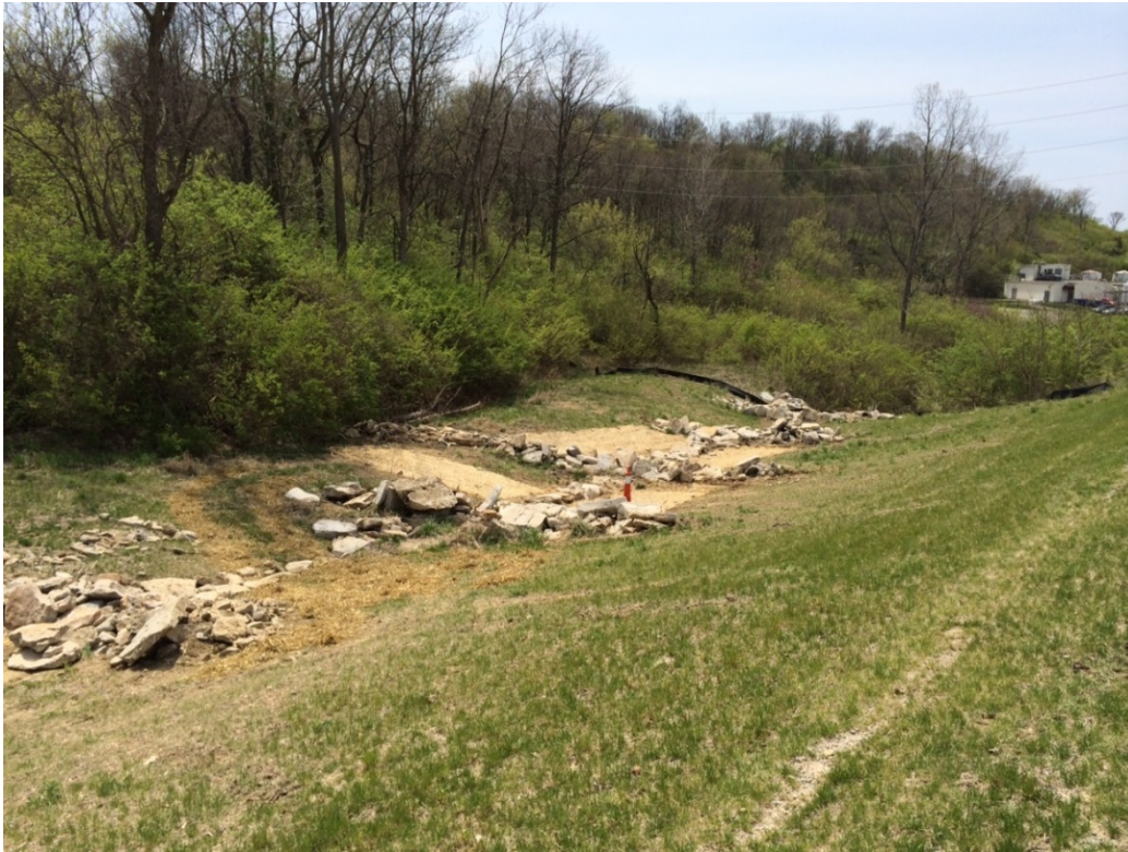
Figure 14. Erosion Controls East of Vanguard Blvd. Installed in April 2014
