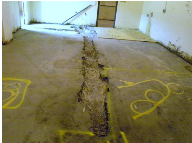
Figure C-9. T Bldg. Room 16 View H
