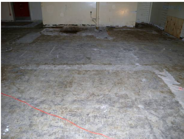
Figure C-14. T Bldg. Room 61 View C
