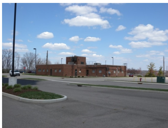
Figure 5. Guard House (GH) Building
