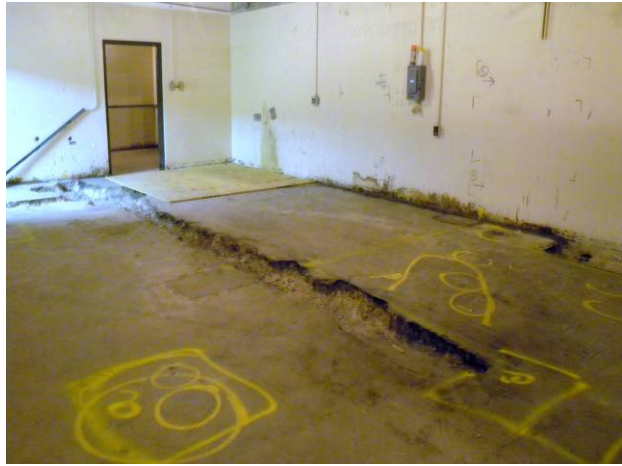
Figure C-11. T Bldg. Room 16 View J
