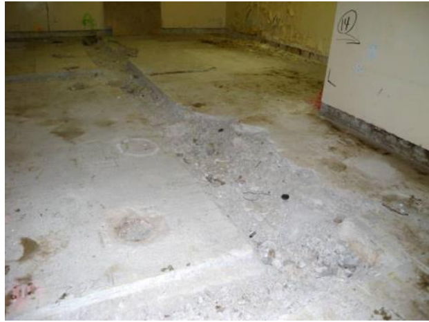
Figure C-25. T Bldg. Room 63 View F
