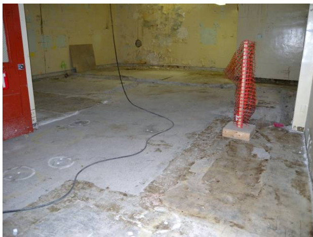
Figure C-20. T Bldg. Room 63 View A
