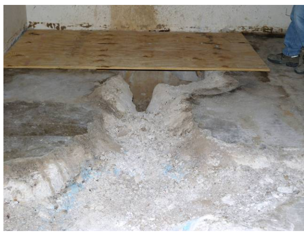
Figure C-4. T Bldg. Room 16 View C
