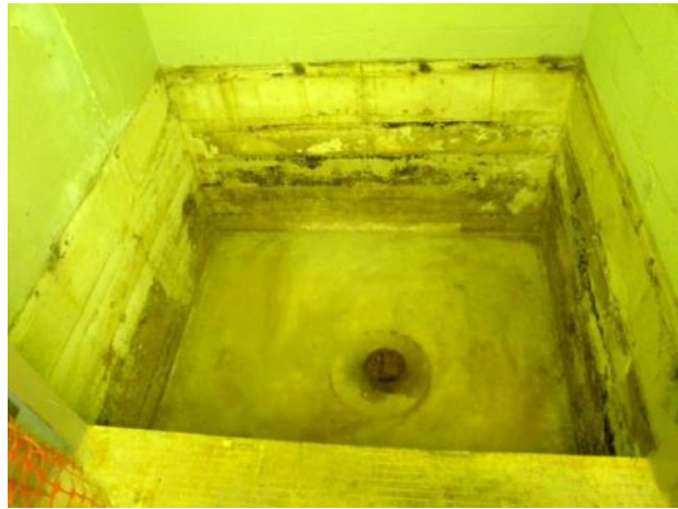
Figure C-31. T Bldg. Room 62 View L
