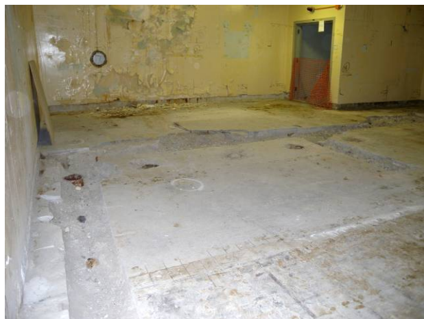
Figure C-22. T Bldg. Room 63 View C
