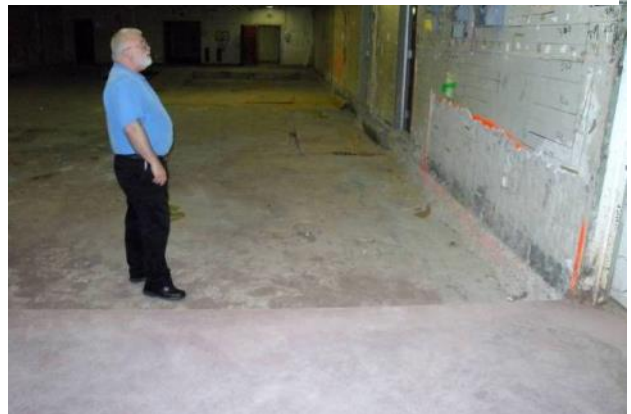
Figure C-39. T Bldg. Rooms 39–44 and 48–50 View B
