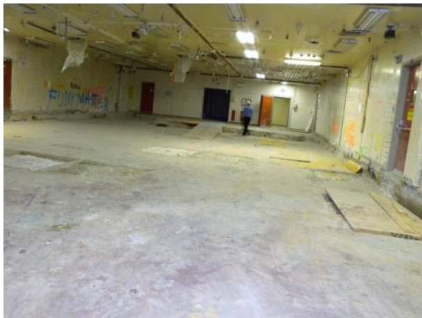
Figure C-40. T Bldg. Rooms 39–44 and 48–50 View C
