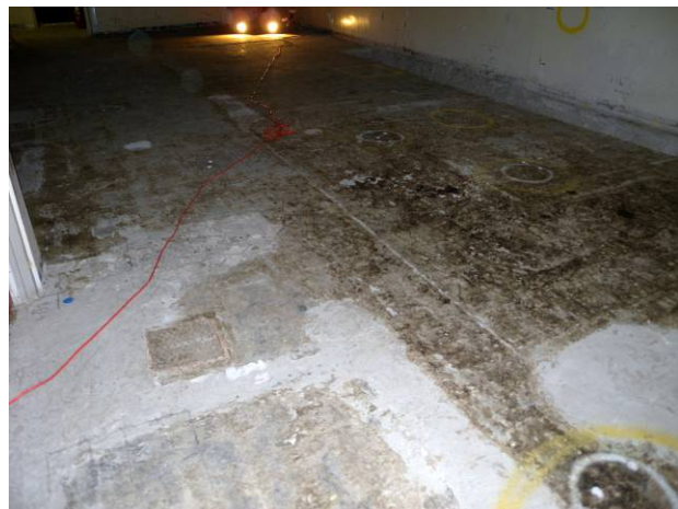
Figure C-15. T Bldg. Room 61 View D
