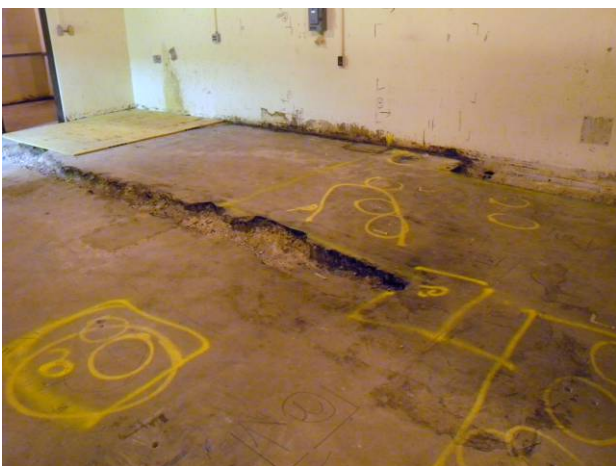
Figure C-10. T Bldg. Room 16 View I
