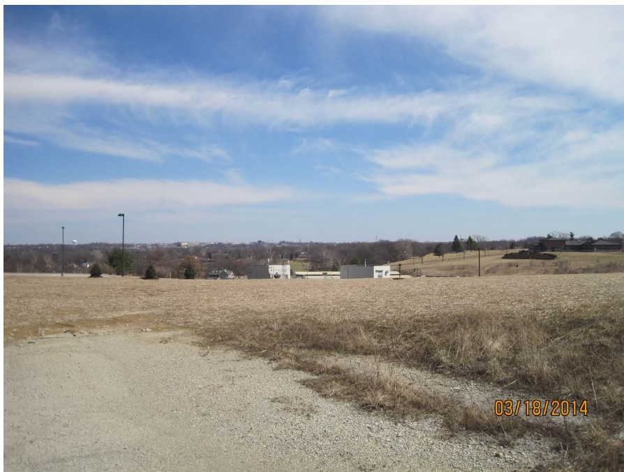
Figure 17. Area After Building 28 Demolition. The Top of Building 45 is Visible in the Center
