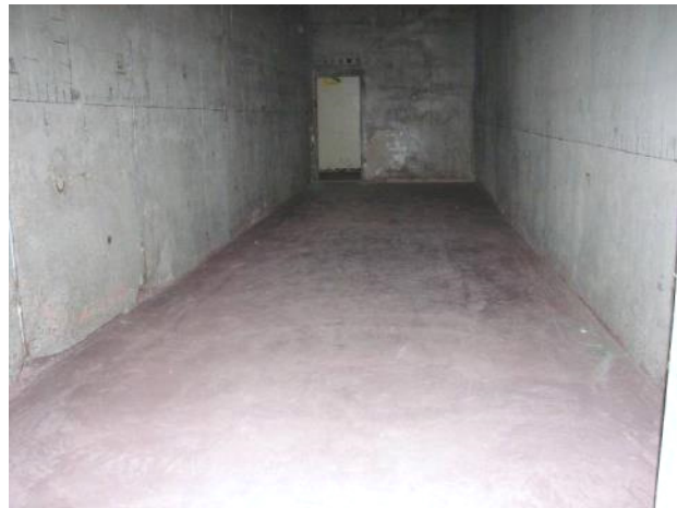
Figure C-37. T Bldg. Room 59 View F
