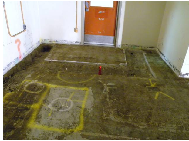
Figure C-17. T Bldg. Room 61 View F
