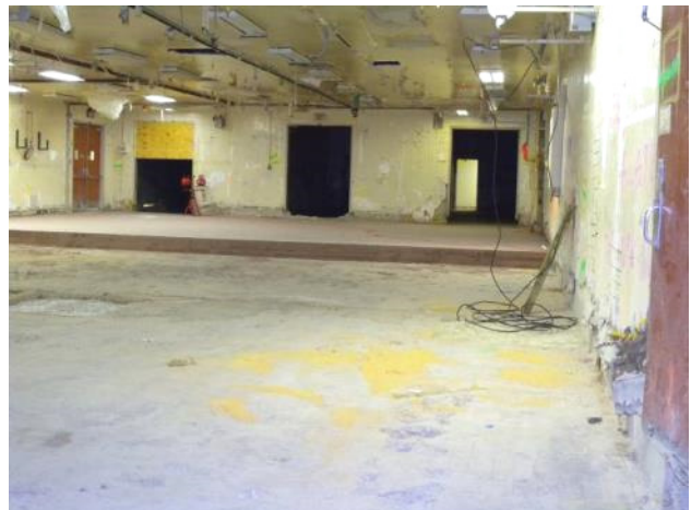
Figure C-47. T Bldg. Rooms 39-44 and 48-50 View J
