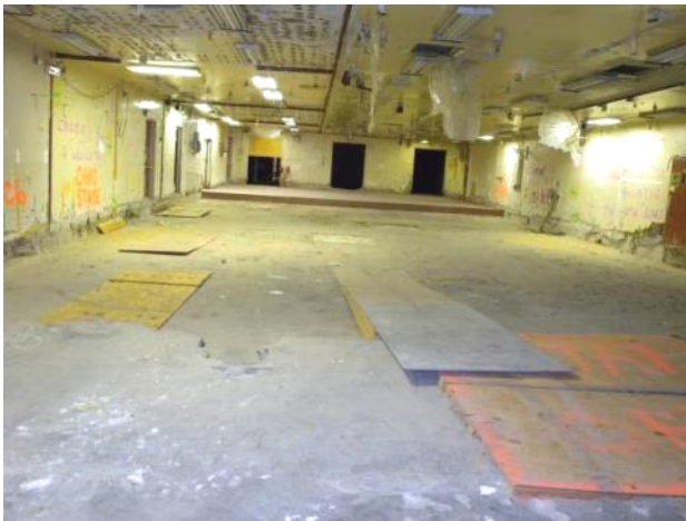
Figure C-44. T Bldg. Rooms 39-44 and 48-50 View G
