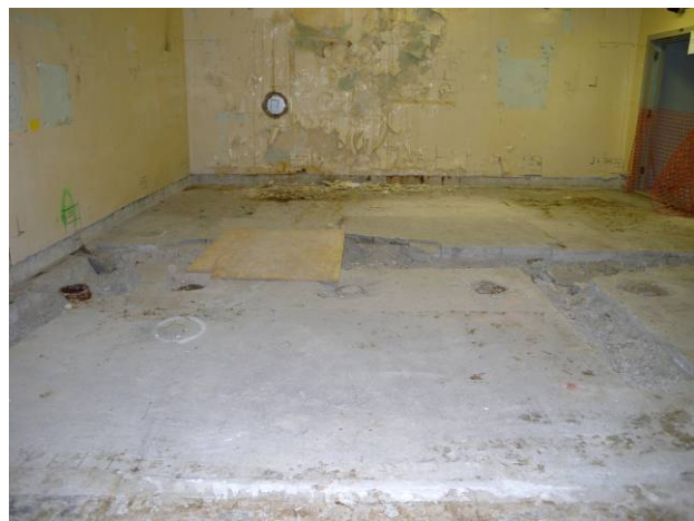
Figure C-21. T Bldg. Room 63 View B
