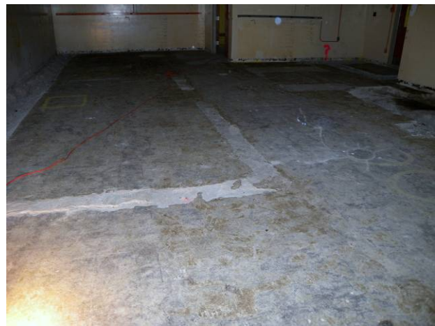
Figure C-13. T Bldg. Room 61 View B
