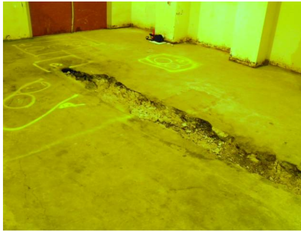
Figure C-7. T Bldg. Room 16 View F
