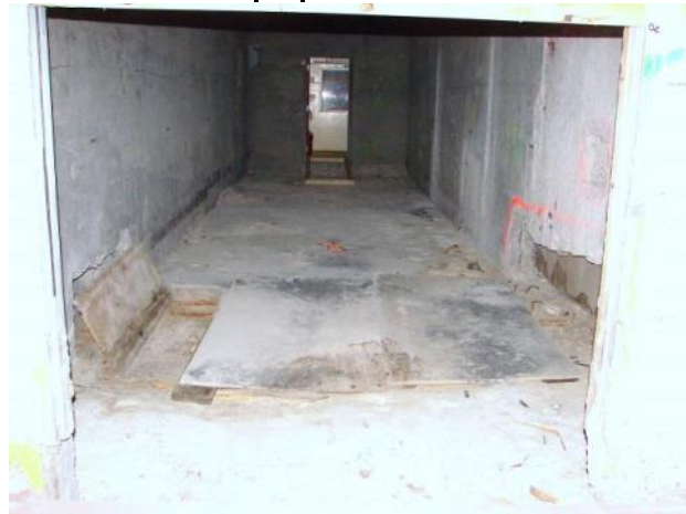
Figure C-33. T Bldg. Room 57 View B
