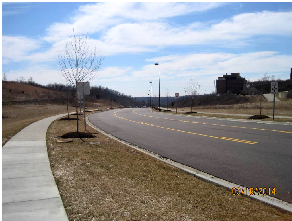
Figure 9. Vanguard Blvd. Looking Southwest Toward Central Office Support Building
