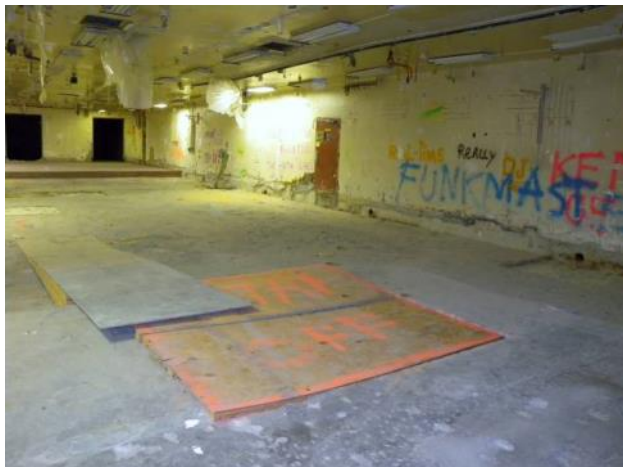
Figure C-46. T Bldg. Rooms 39-44 and 48-50 View I
