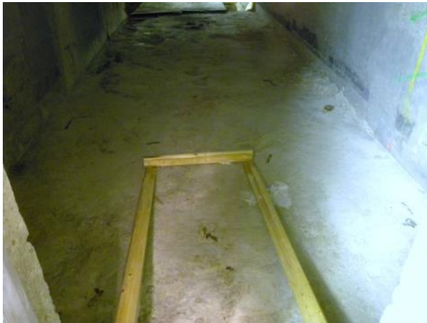
Figure C-32. T Bldg. Room 57 View A
