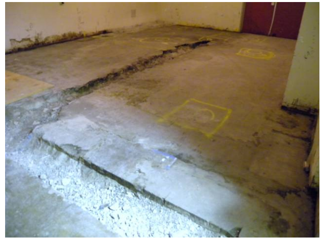
Figure C-3. T Bldg. Room 16 View B
