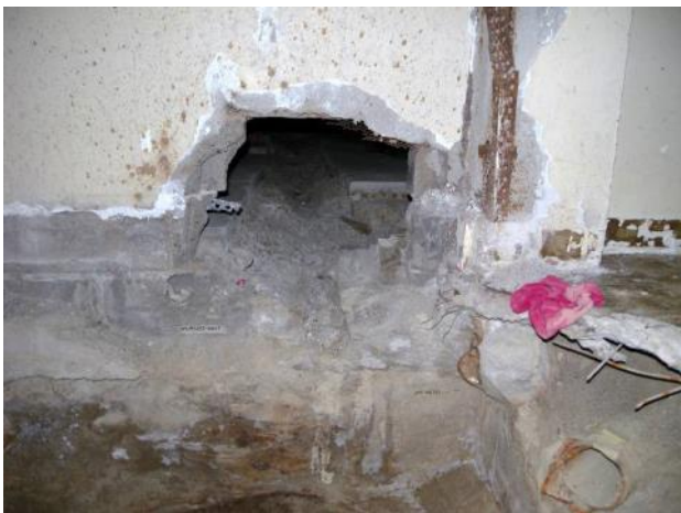
Figure C-28. T Bldg. Room 63 View I
