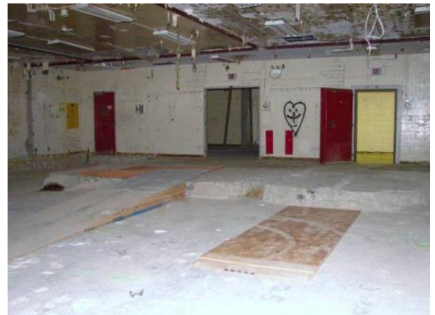
Figure C-41. T Bldg. Rooms 39–44 and 48–50 View D
