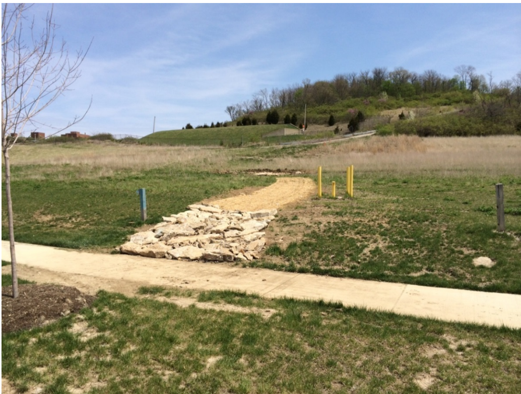
Figure 15. Erosion Controls in OU-1 Area Installed in April 2014
