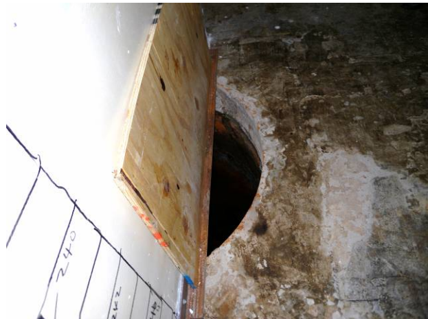
Figure C-19. T Bldg. Room 61 View H
