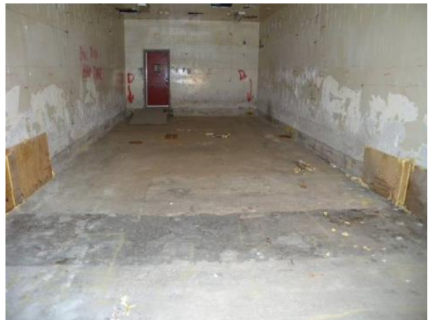
Figure C-35. T Bldg. Room 58 View D
