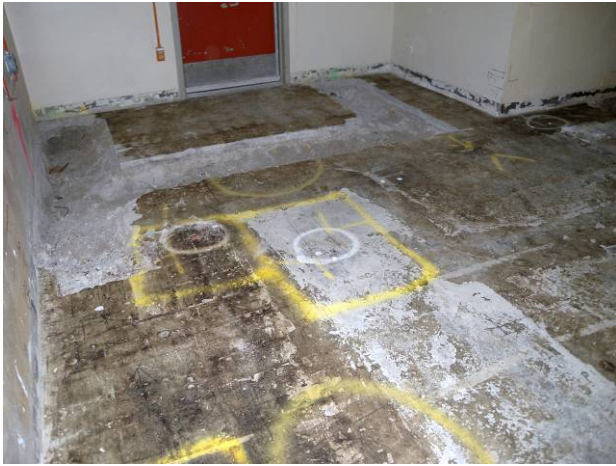
Figure C-16. T Bldg. Room 61 View E
