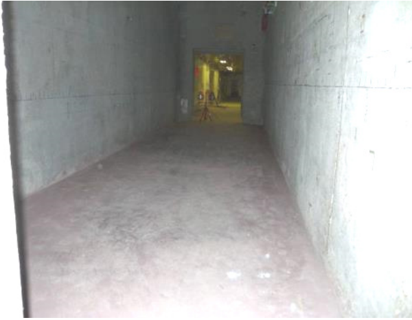
Figure C-36. T Bldg. Room 59 View E
