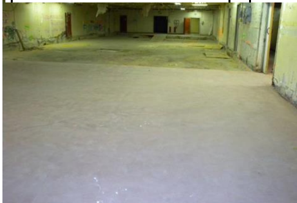
Figure C-38. T Bldg. Rooms 39–44 and 48–50 View A
