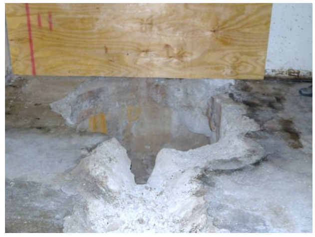
Figure C-5. T Bldg. Room 16 View D
