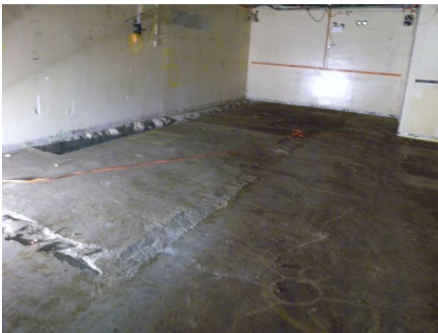
Figure C-12. T Bldg. Room 61 View A
