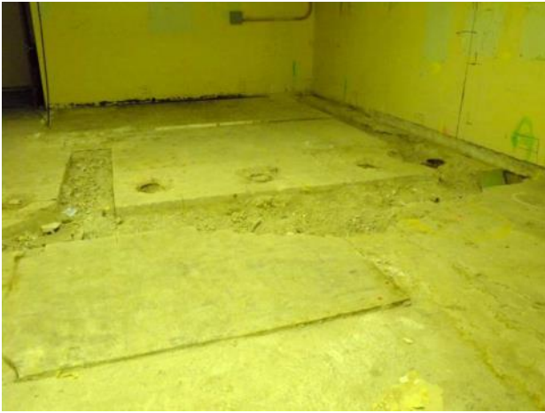
Figure C-24. T Bldg. Room 63 View E
