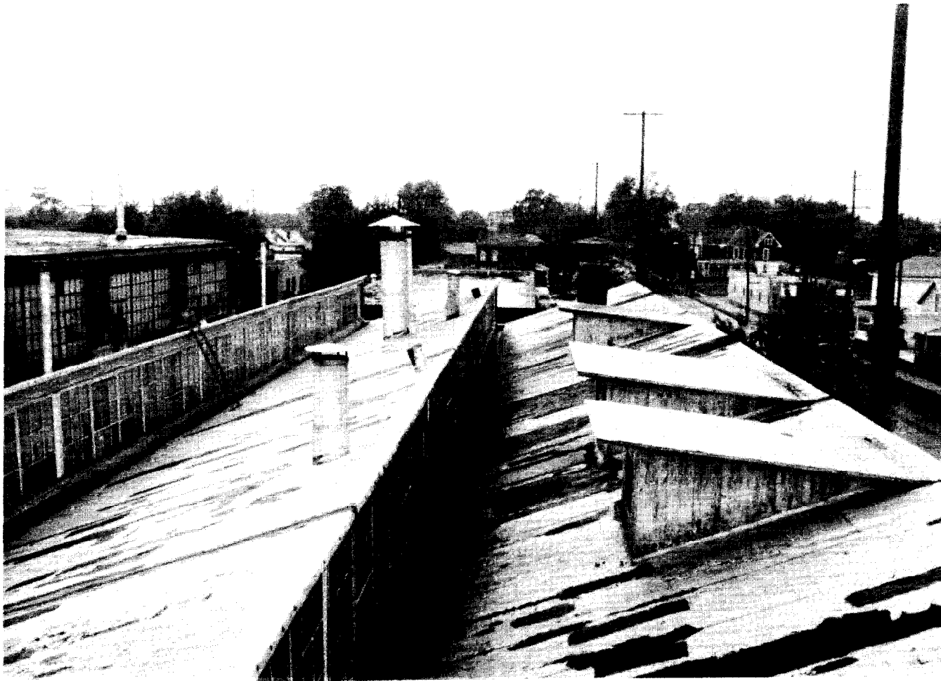
Fig. 6. Sawtooth roof over the area where the MED processing took place, looking west, B&T Metals, Columbus Ohio (CO001).
