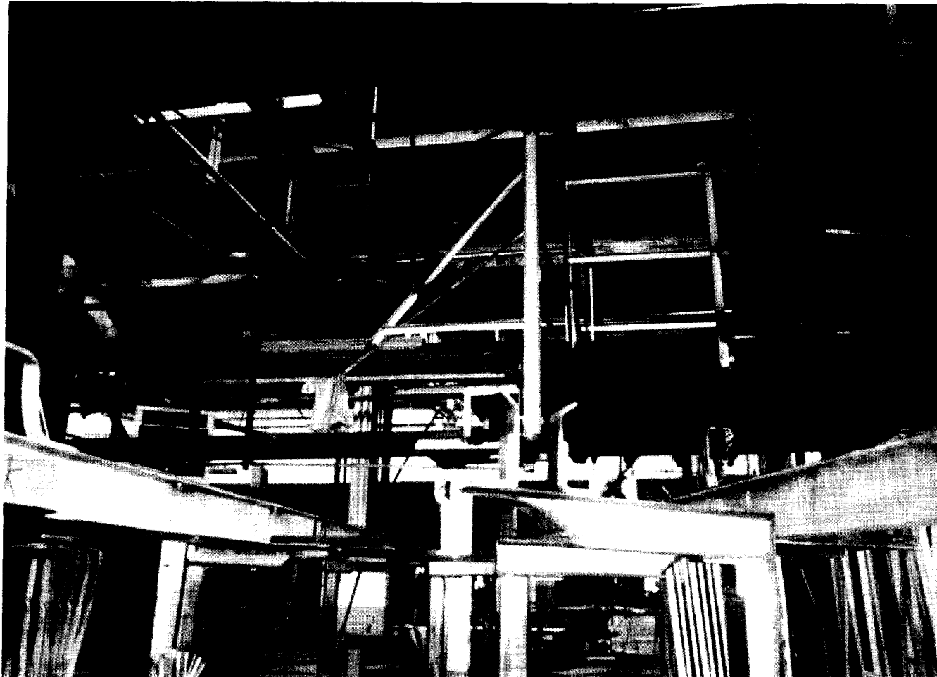
Fig. 5. Support beams inside the main office building, B&T Metals, Columbus, Ohio (CO001).
