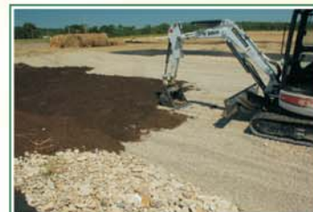
A three-inch mulch layer is applied to the subsurface flow wetland.
