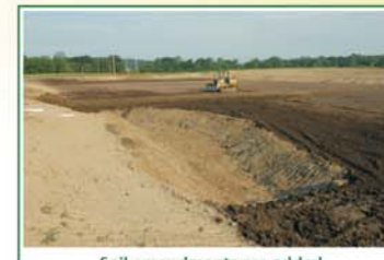
Soil amendments are added to the surface flow wetland basin.
