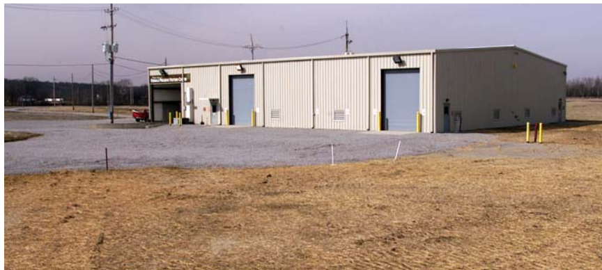
Fig. 2. Former Onsite Warehouse
