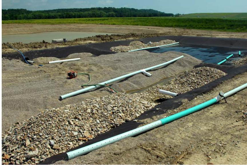
Fig. 3. Installation of Subsurface Wetland Piping and Substrate
