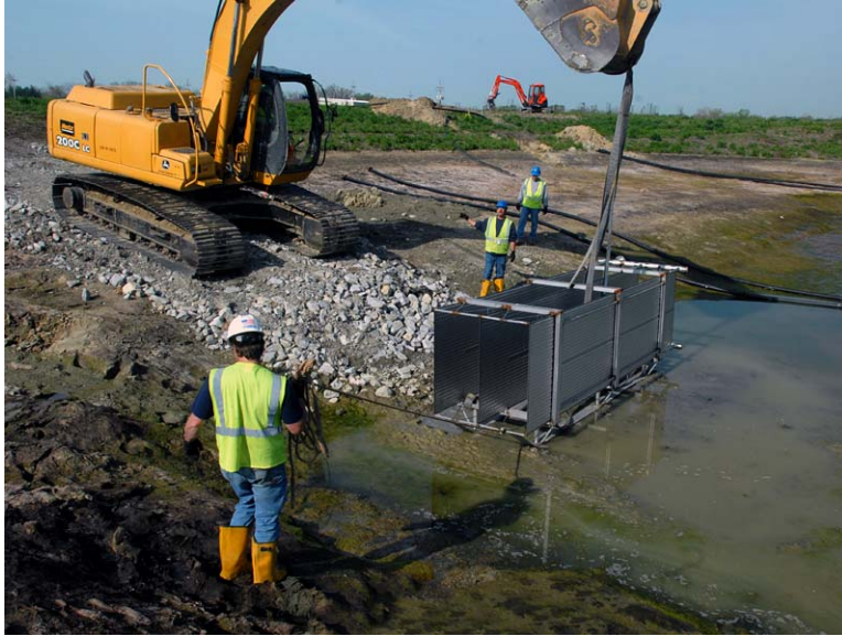
Fig. 4. Ground Source Heat Pump Installation
