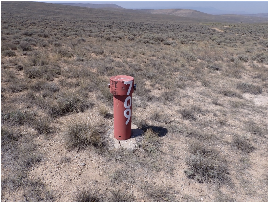
PL-4. Cracked Base of Well 0709
