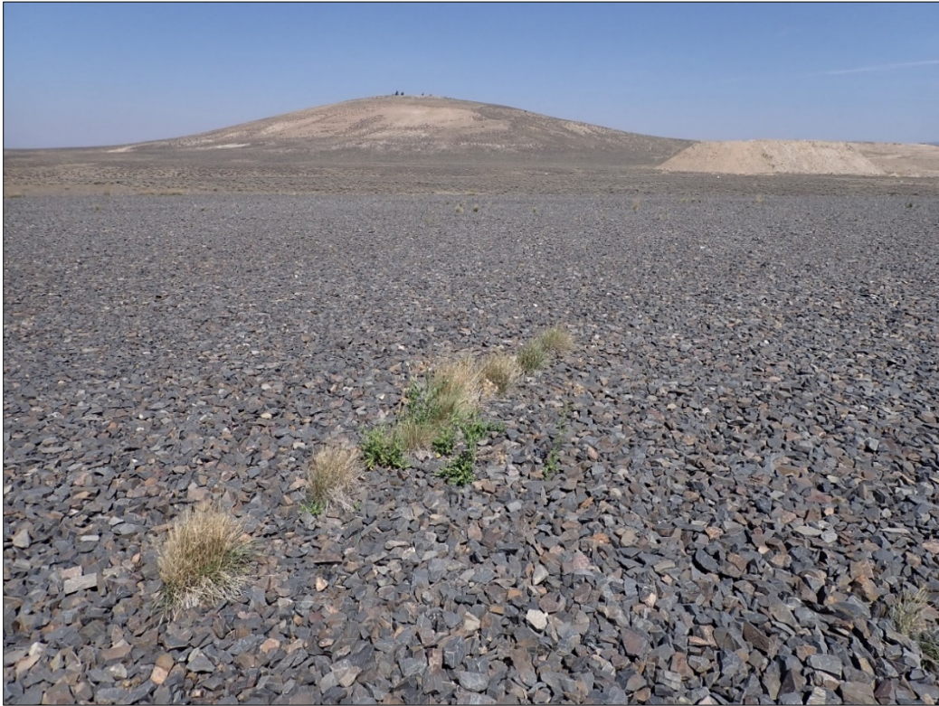
PL-5. Vegetation on Disposal Cell Top Slope
