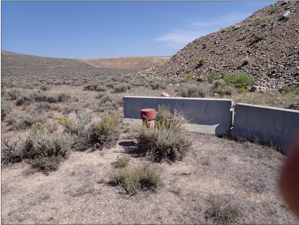
PL-3. Well 0716 Overgrown with Vegetation and Nearby Spoil Pile
