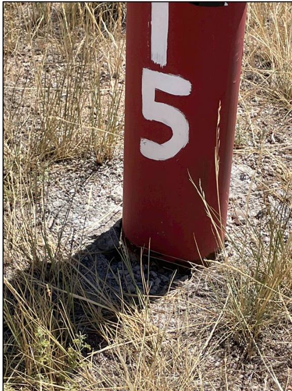
PL-5. Monitoring Well 0715 with Concrete Spalling at Base
