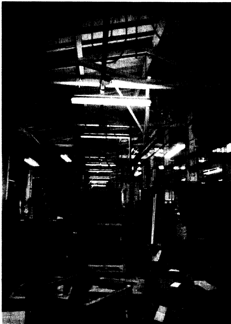
Fig. 4. Interior view of the building at Diebold Safe Company, 1550 Grand Boulevard, Hamilton, Ohio (HO001), showing the cross braces.
