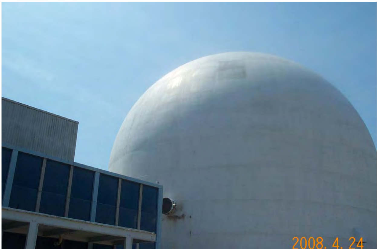
PIQ 4/2008. PL-2. Containment Dome.
