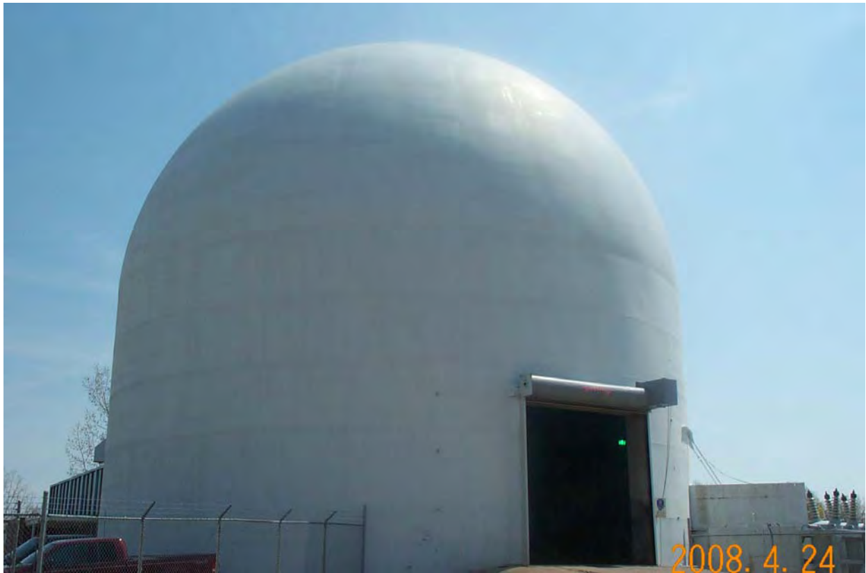
PIQ 4/2008. PL-1. Containment Dome.
