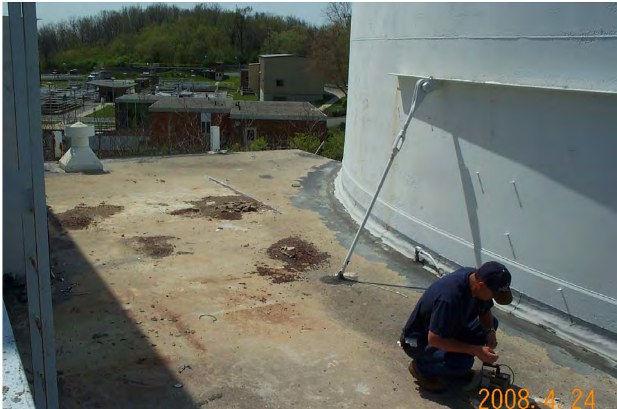
PIQ 4/2008. PL-3. Flat Roof, 111-foot level, HVAC Equipment Removed.
