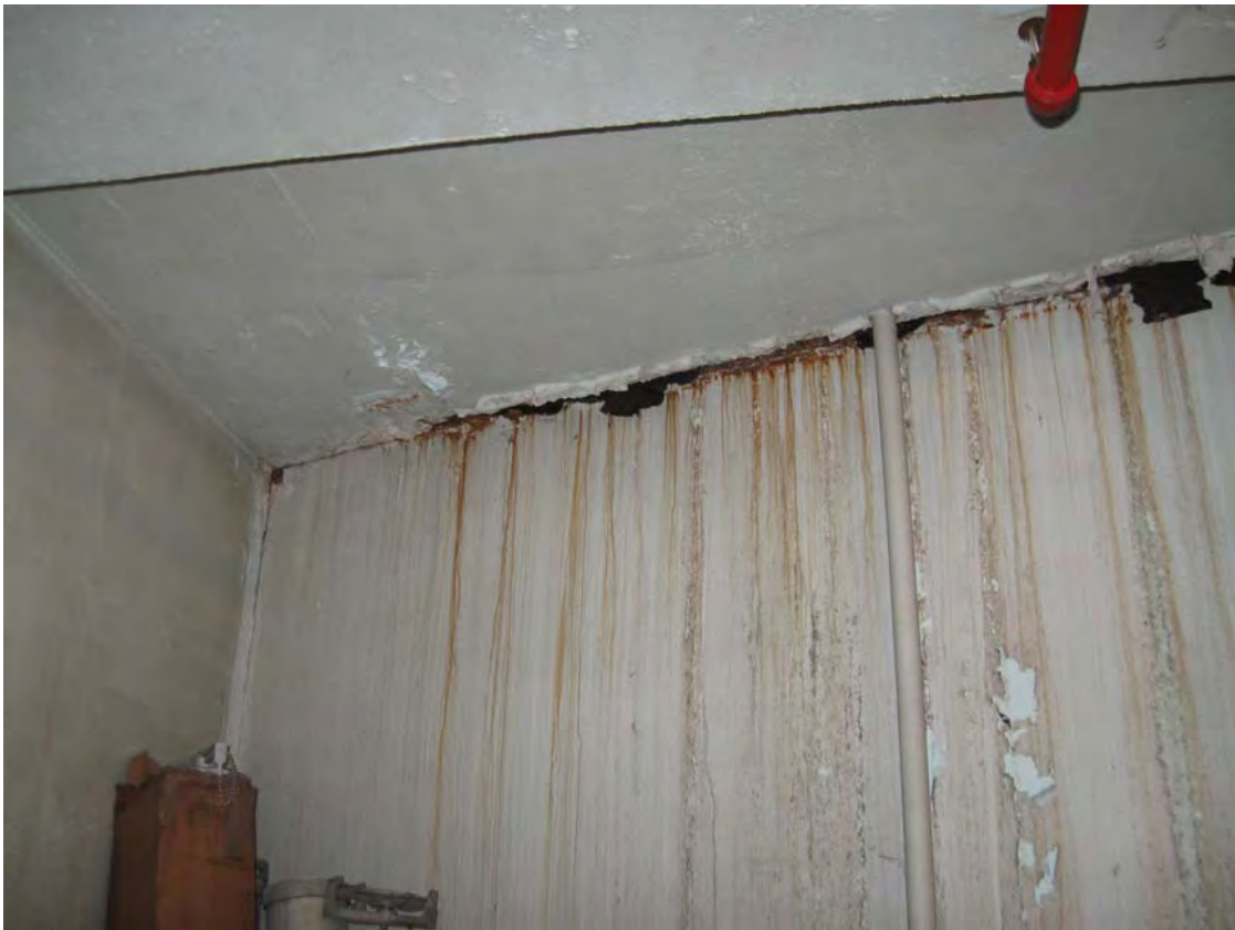
PIQ 4/2009. PL-7. Water corrosion along seam of wall in Room B-1: 79-foot level.
