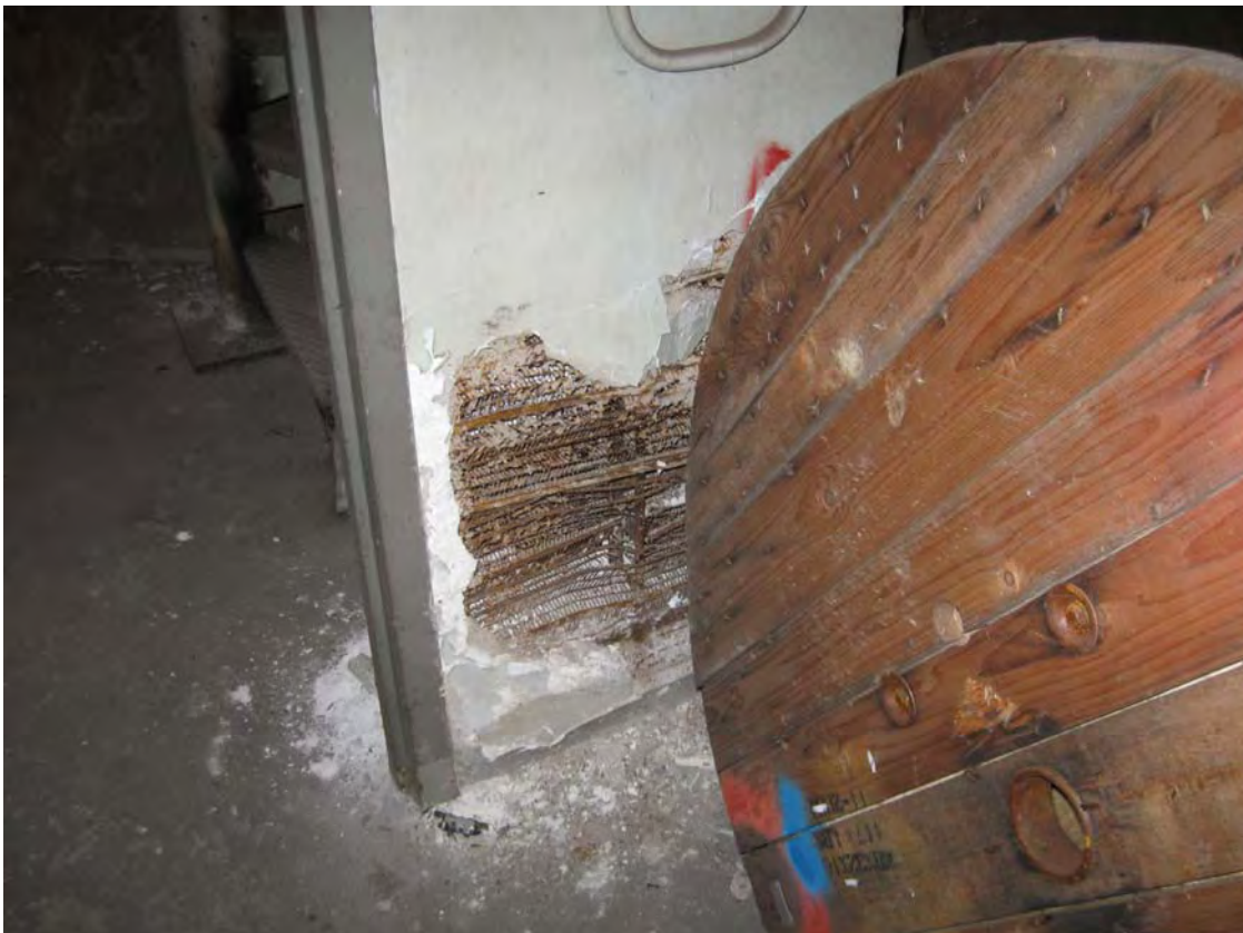
PIQ 4/2009. PL-6. Damage to Walls by Cable Spools: 56 foot level.
