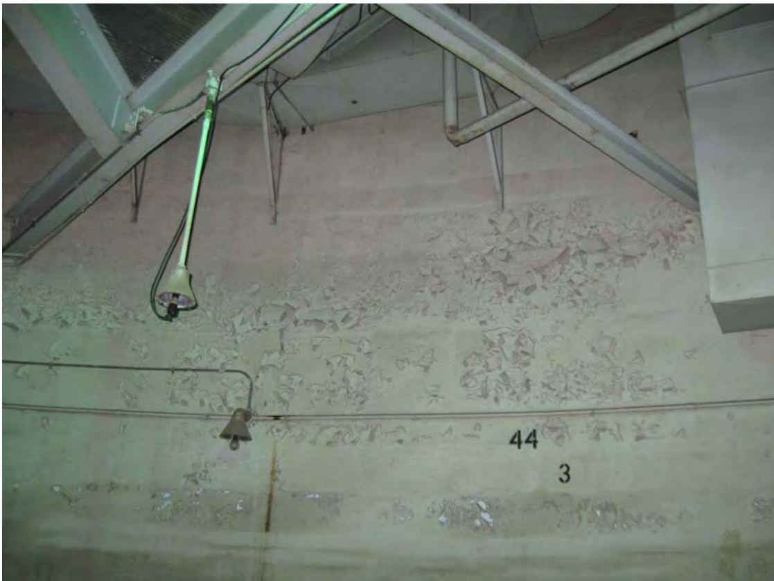
PIQ 4/2009. PL-4. Peeling Paint on interior wall: 56 foot level.
