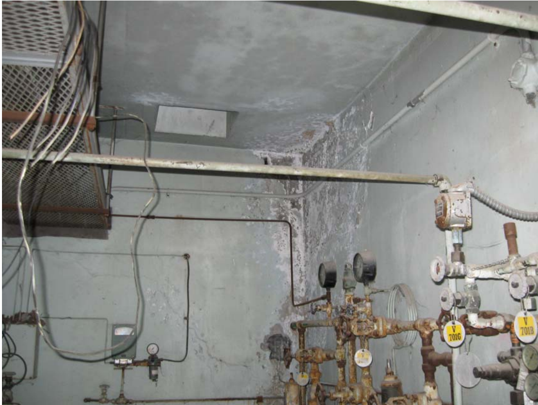
PIQ 4/2010. PL-11. Water appears to be leaking down the back corner of Room 125.
