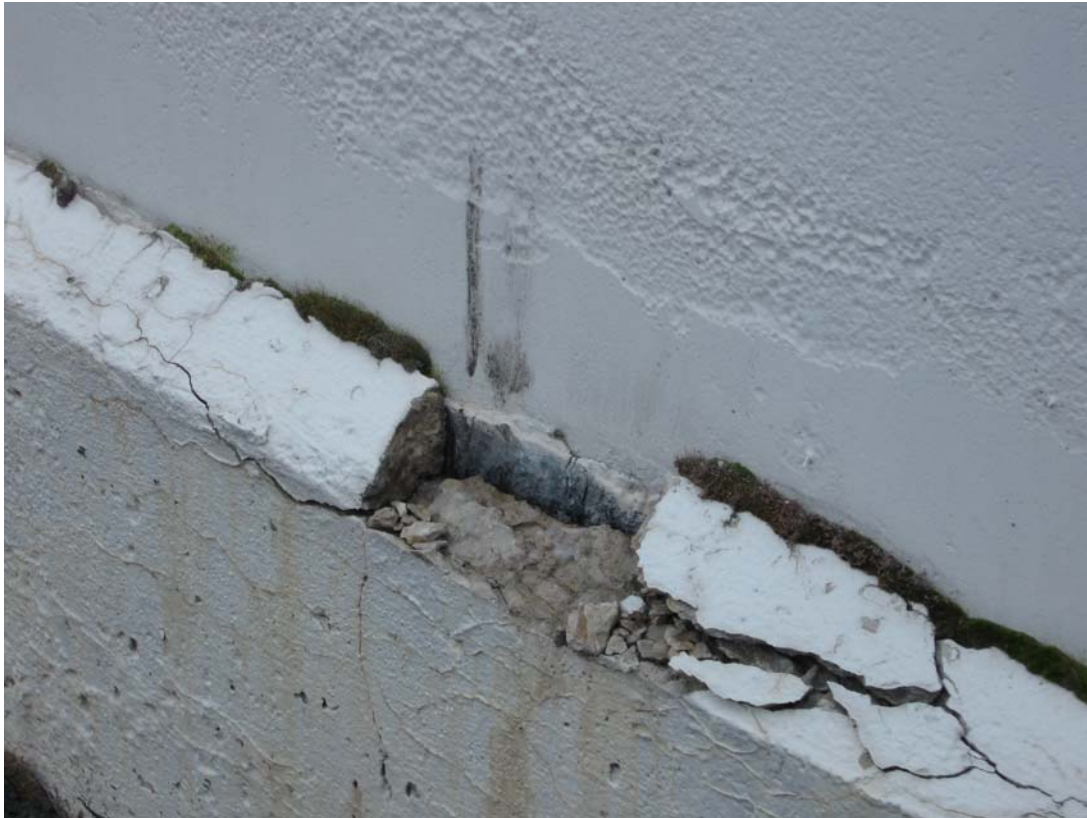
PIQ 4/2010. PL-17. Damaged concrete around base of containment dome. Top seam needs to be cleaned out and weatherproofed to keep water from causing further damage.
