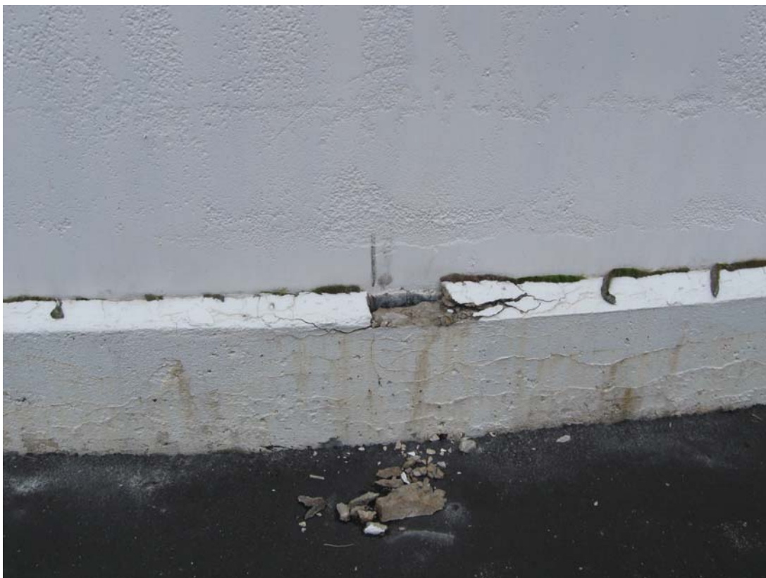
PIQ 4/2010. PL-16. Concrete damage around the base of containment building. Water is seeping into small crack at base of building and impacting concrete.
