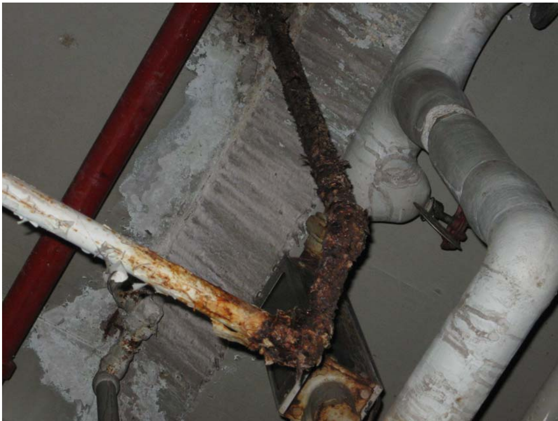
PIQ 4/2010. PL-8. Pipe in ceiling of Room B-5 of auxiliary building. Water was slowly dripping down the outside surface of the pipe during the inspection.
