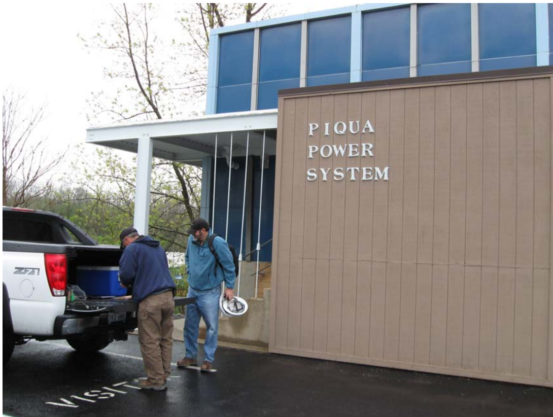
PIQ 4/2010. PL-1. Entrance to the Piqua auxiliary building.
