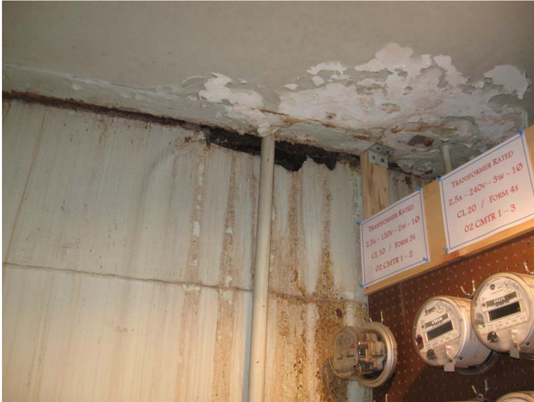
PIQ 4/2010. PL-7. Water and rust stains on seam of ceiling in OAP room of auxiliary building: 79-foot level.
