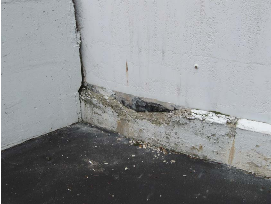
PIQ 4/2010. PL-15. Concrete damage around base of containment building. Water is seeping into small crack at base of building and impacting concrete.
