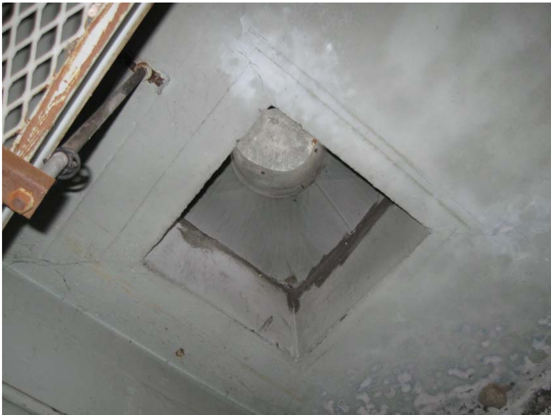
PIQ 4/2010. PL-12. Water noticeable around air vent in ceiling of Room 125: 100-foot level.
