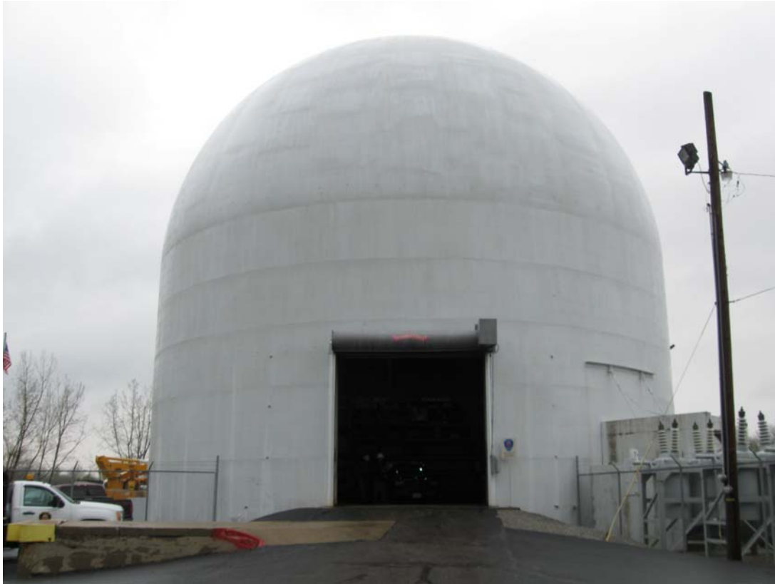
PIQ 4/2010. PL-3. Exterior of the Piqua containment building.
