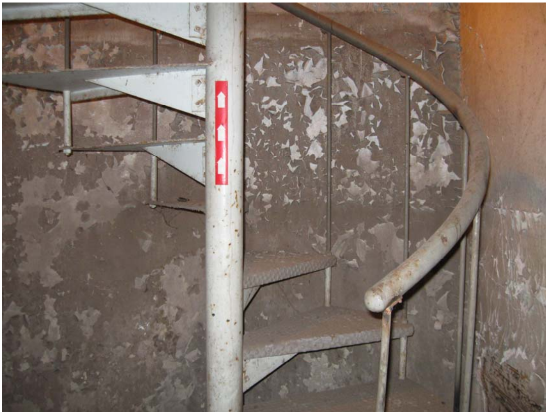
PIQ 4/2010. PL-4. Base of spiral staircase: 56-foot level.
