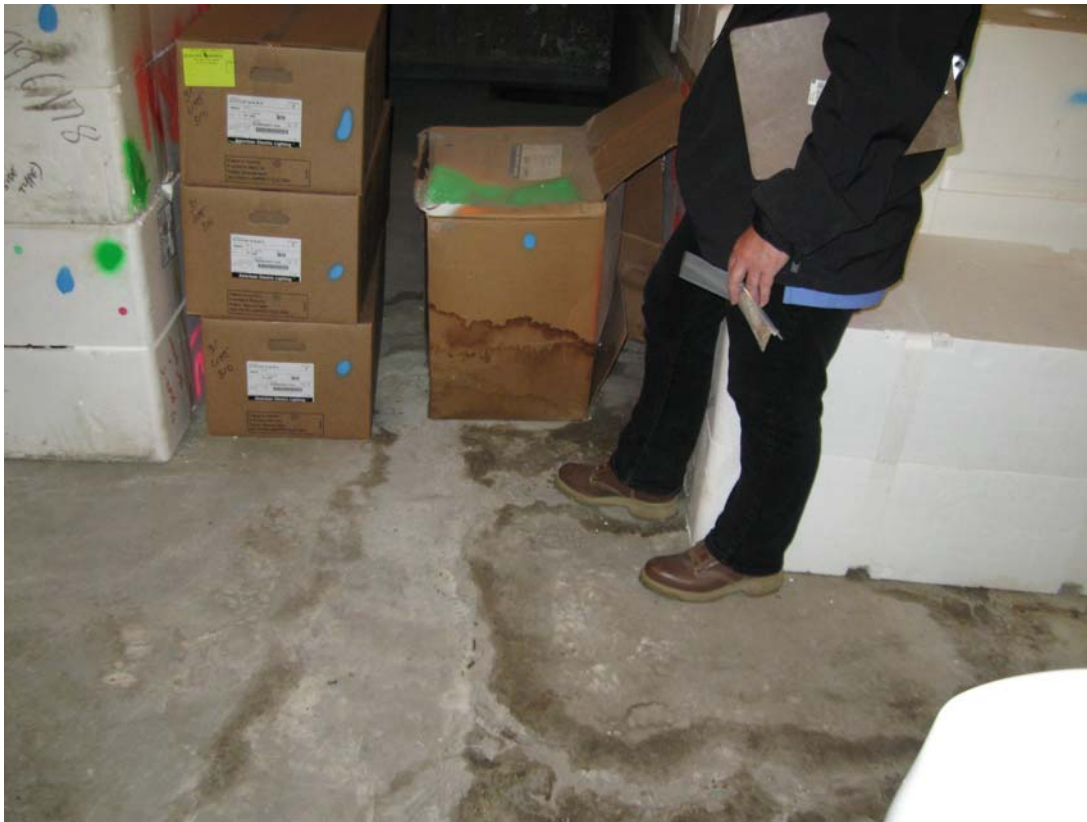
PIQ 4/2010. PL-9. Water stains on the floor of Room B-5 of auxiliary building: 79-foot level. Water staining on boxes in background.
