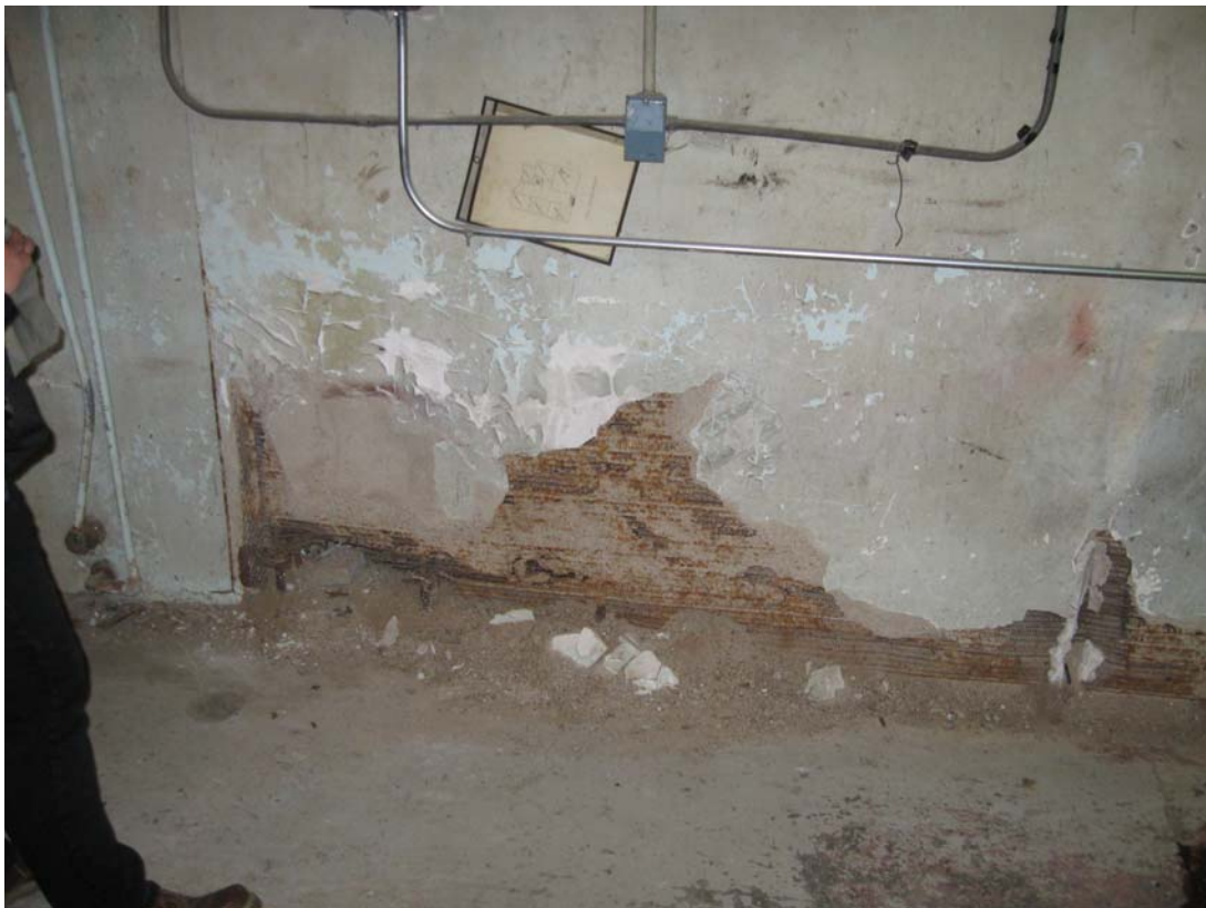
PIQ 4/2010. PL-6. Damage to base of interior wall in Room B-4 of auxiliary building: 79-foot level.
