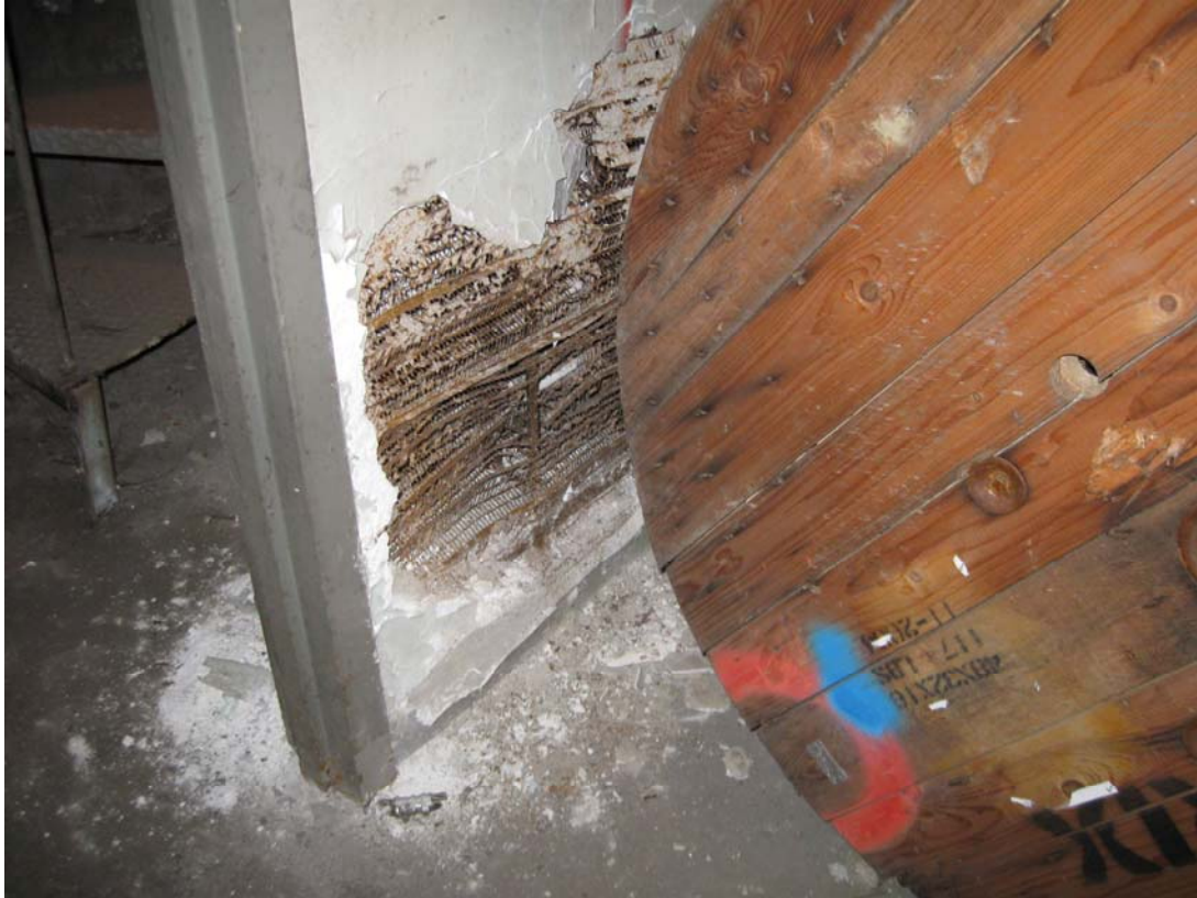
PIQ 4/2010. PL-5. Damage to walls by cable spools: 56-foot level.
