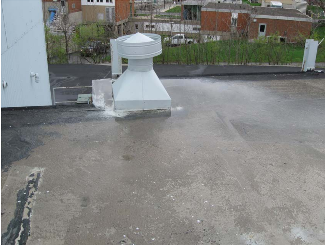
PIQ 4/2010. PL-13. Roof above Room 125. Water collected in corner. Corner of roof not draining properly.
