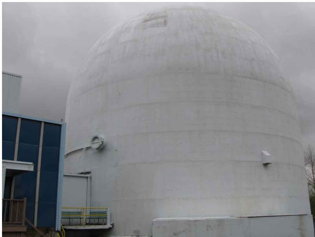
PIQ 4/2010. PL-2. Exterior of the Piqua containment building.
