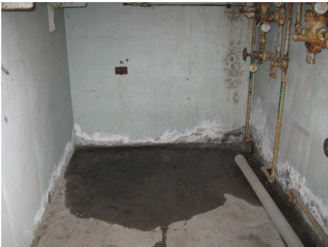
PIQ 4/2010. PL-10. Water present on floor of Room 125, off the outside loading dock: 100-foot level.
