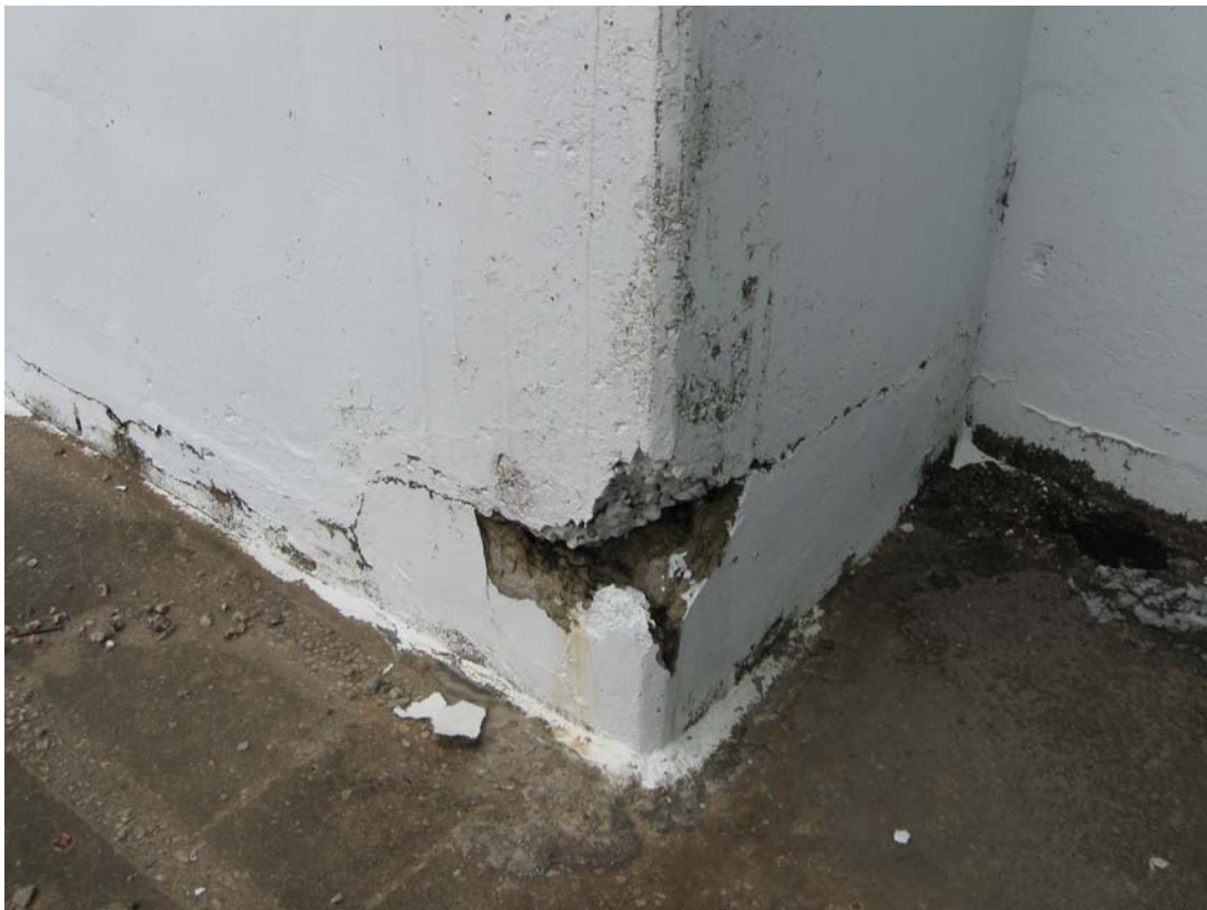
PIQ 4/2010. PL-14. Concrete damage on outside corner of Room 125: 100-foot level.
