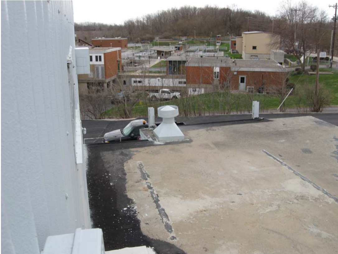
PIQ 4/2011. PL-9. Repair made to corner of roof above Room 125. Water no longer ponding on area of roof.
