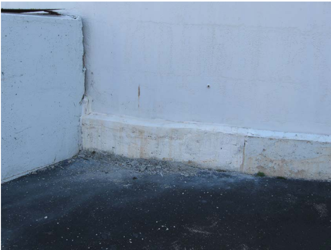
PIQ 4/2011. PL-10. Repair made to concrete at base of containment dome.
