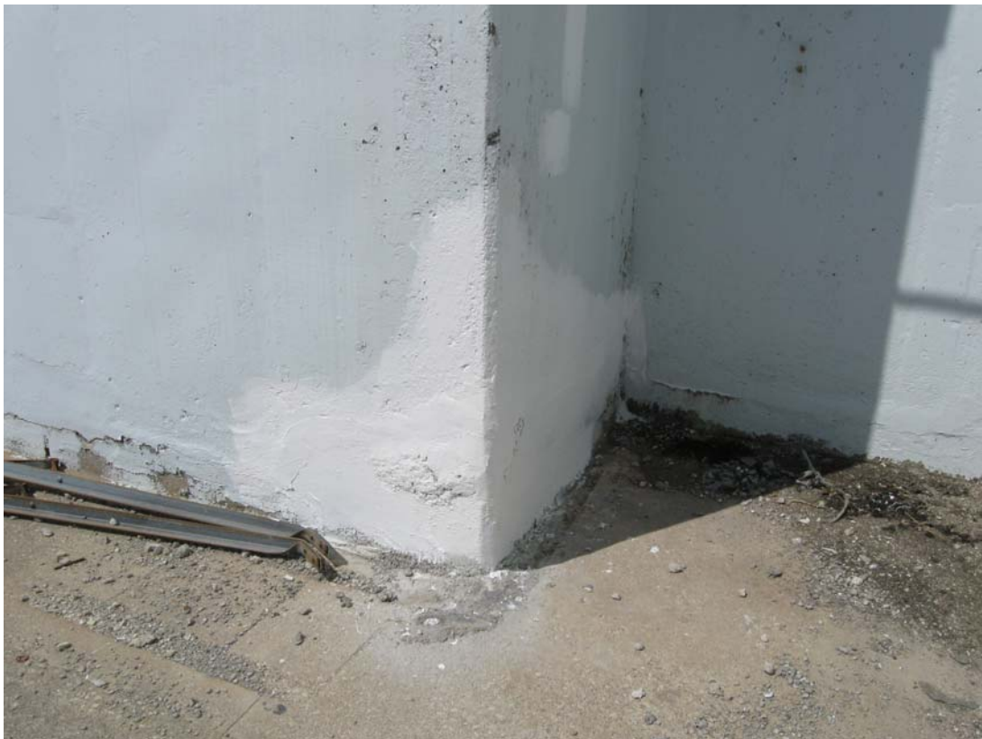
PIQ 4/2011. PL-8. Repairs made to corner of Room 125.
