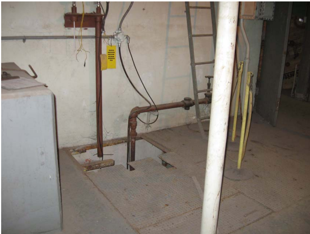
PIQ 4/2011. PL-12. Sump in basement of containment structure.
