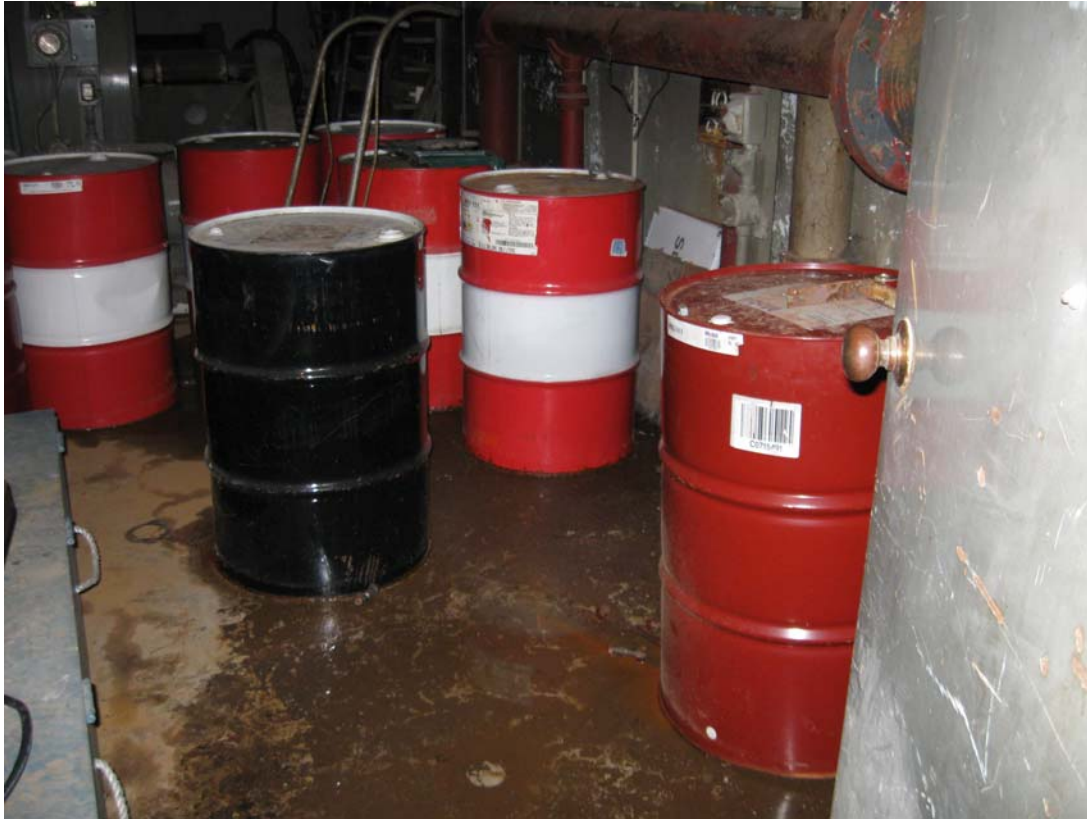
PIQ 4/2011. PL-3. Water on floor of Room B-3.
