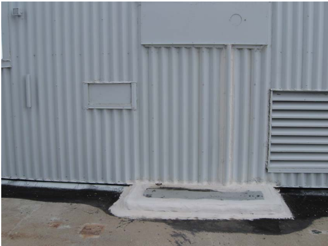
PIQ 4/2011. PL-6. Repair to roof. Above fresh water stains on wall of Room B-5.
