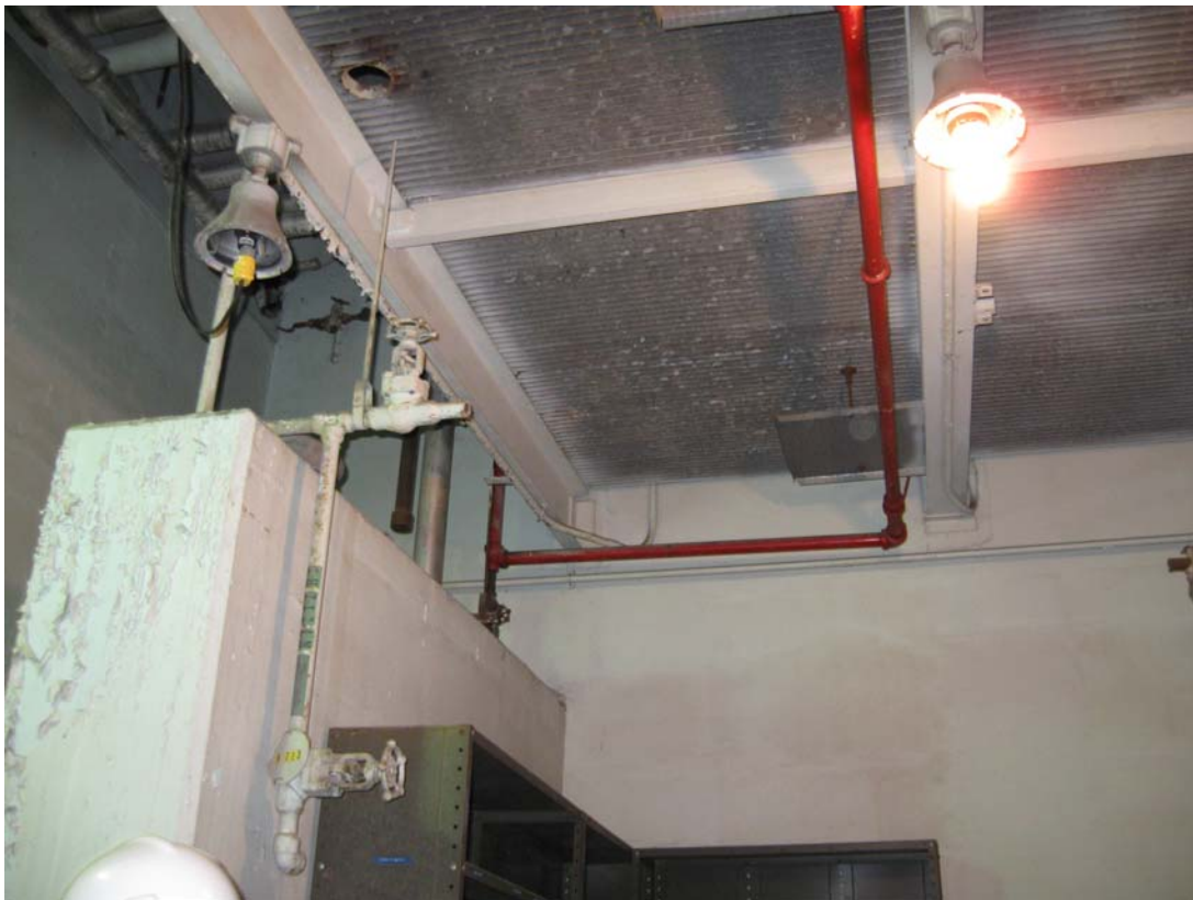
PIQ 4/2011. PL-4. Old pipes from sprinkler system removed.
