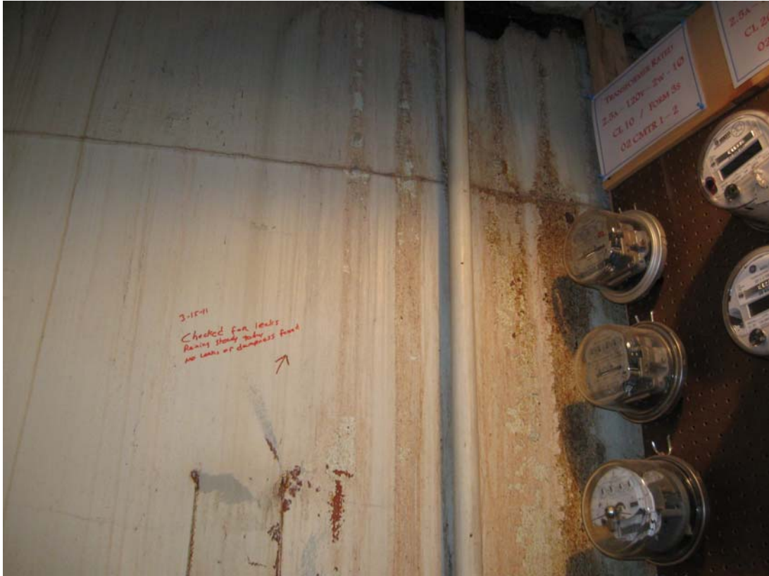
PIQ 4/2011. PL-5. Fresh water stains on wall of Room B-5.
