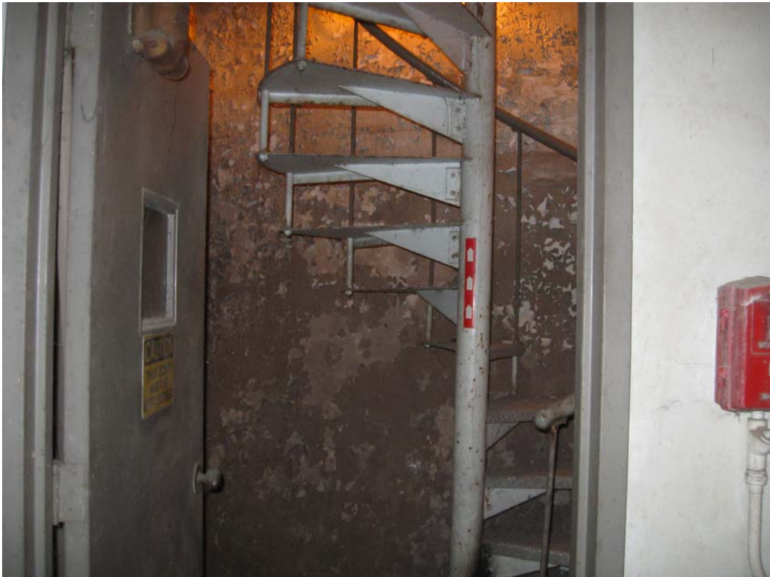
PIQ 4/2011. PL-2. Base of spiral staircase.
