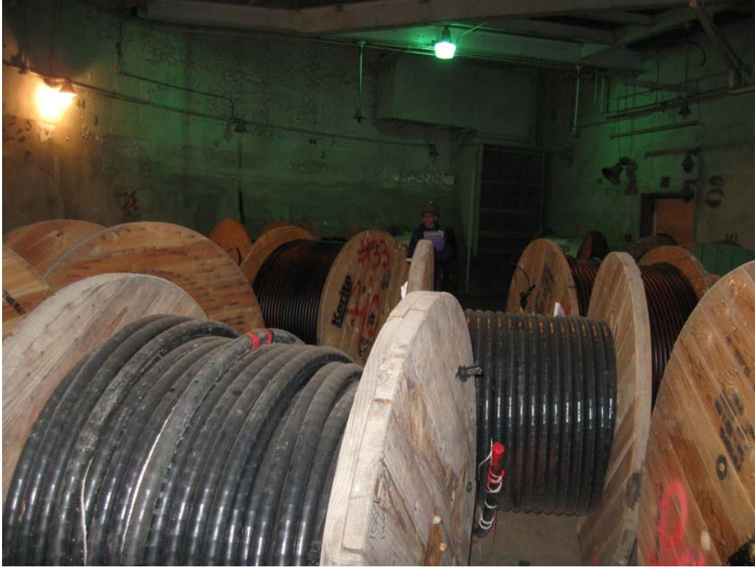
PIQ 4/2011. PL-1. Cable spools stored on 56-foot level of containment structure.
