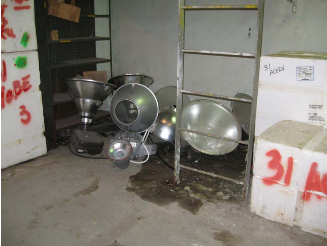
PIQ 4/2011. PL-7. Water of floor of Room B-5.
