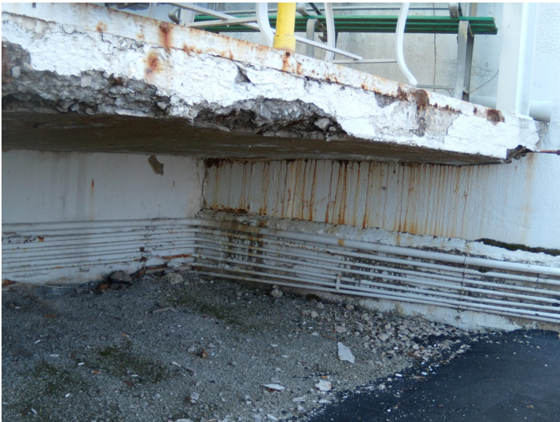
PIQ 4/2014. PL- 8. Break platform on northwest side of Auxiliary Building.
