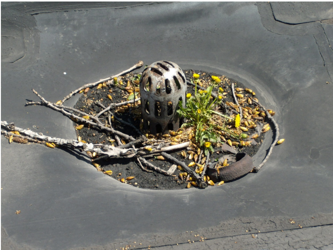
PIQ 4/2014. PL- 10. Weeds growing around roof drains.
