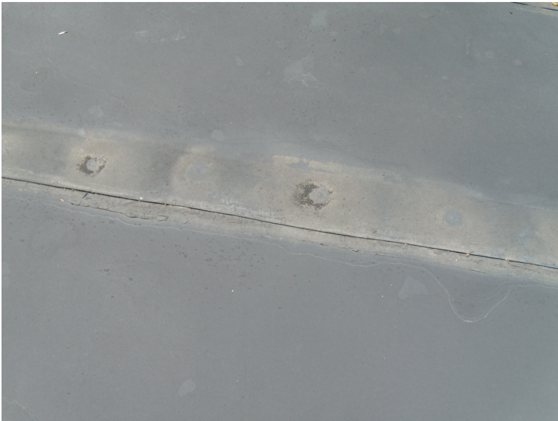
PIQ 4/2014. PL- 9. Seams in roof material separating.
