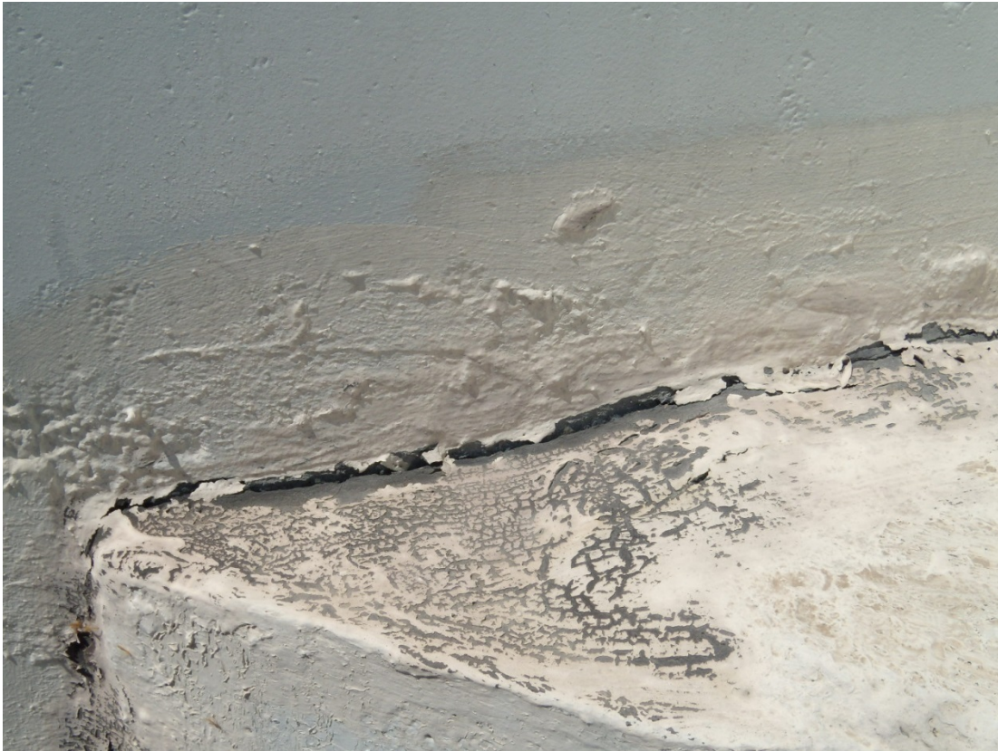
PIQ 4/2014. PL- 5. Crack around base of containment dome.
