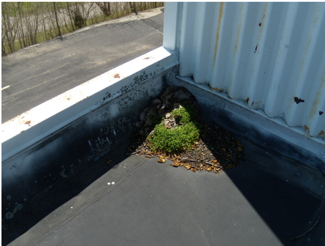
PIQ 4/2014. PL- 11. Weeds growing around roof drains.
