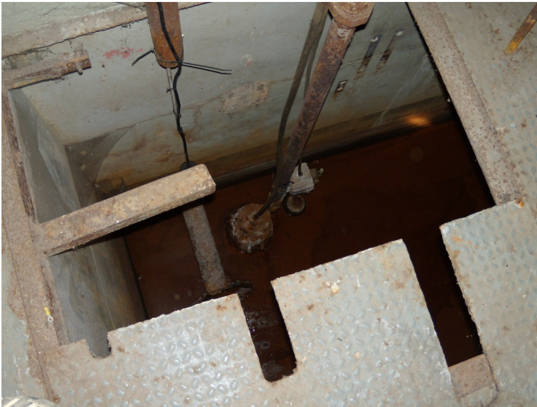
PIQ 4/2014. PL- 13. Water in base of sump.
