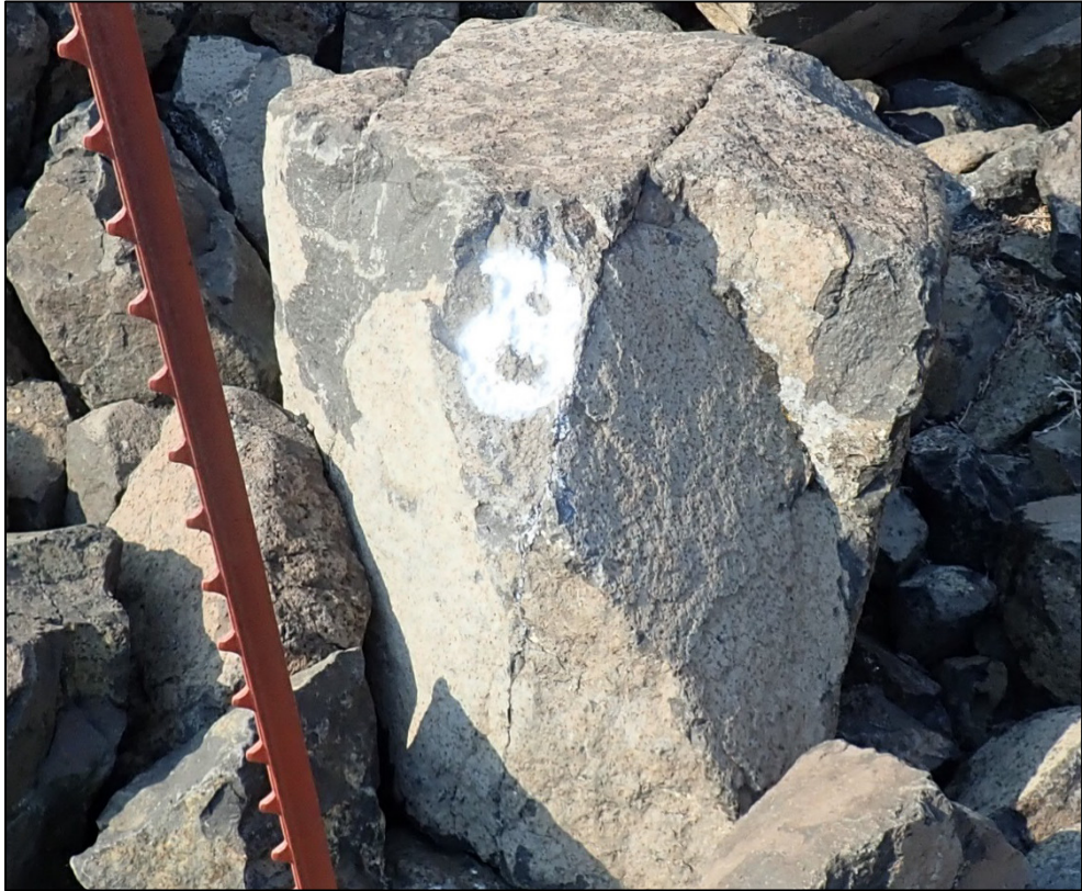
PL-11. Riprap Monitoring Location No. 8 in the Energy Dissipation Area
