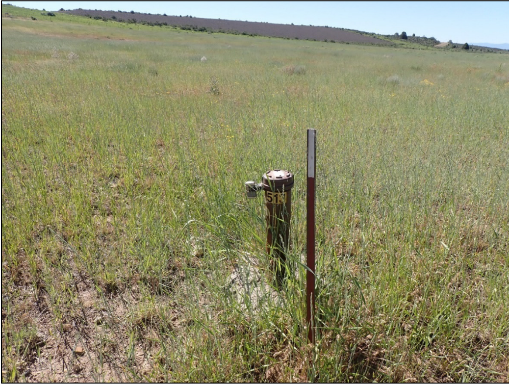
PL-5. Monitoring Well 0513
