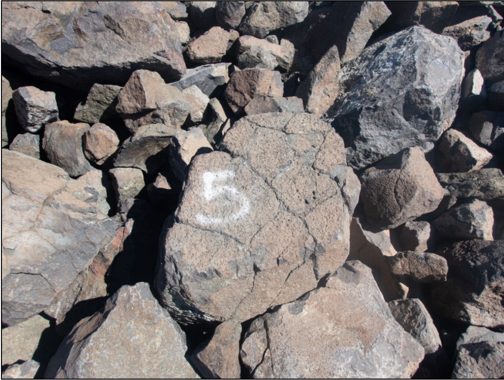
PL-9a. Riprap Monitoring Location No.5 in EDA
