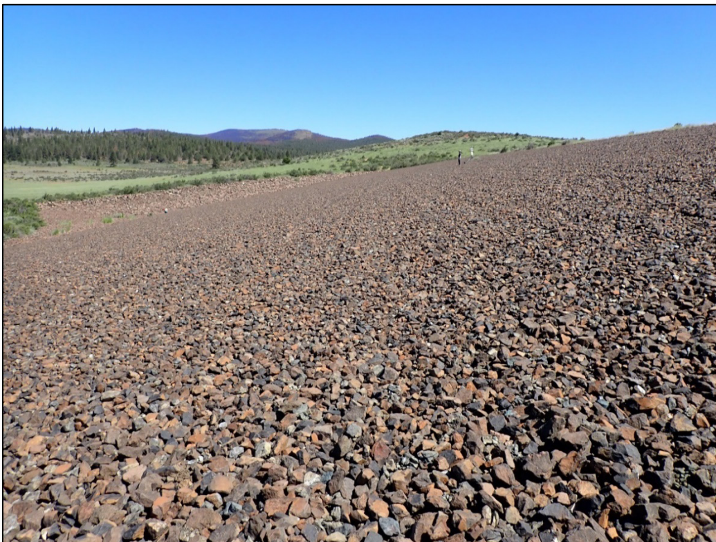
PL-8. West Side Slope of Disposal Cell
