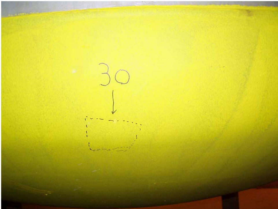
Figure 6. Basement Level – Survey Location 30 on Retention Tank 1
