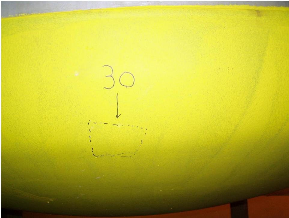
Figure 6. Basement Level – Survey Location 30 on Retention Tank 1
