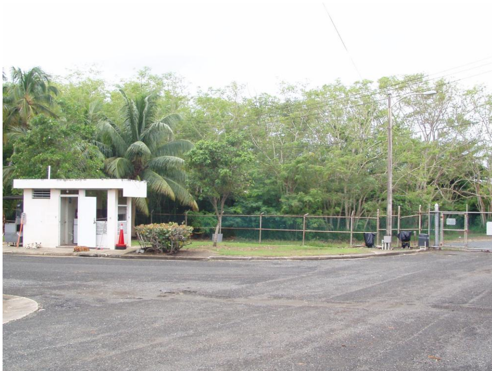
Figure 20. Site Security – Gate Security Building and Main Gate (Motor is Not Operational)
