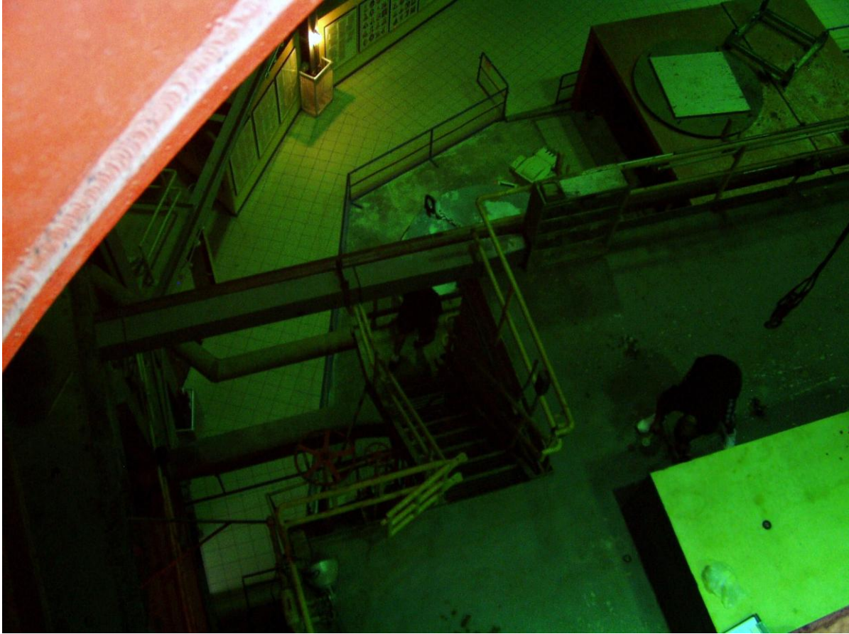
Figure 17. View from Catwalk – West/Northwest Side, Main Level (Survey Technician on Entombment Top Below)
