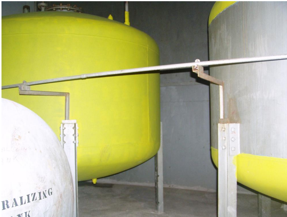
Figure 6. Basement Level – Retention Tanks 2 and 3
