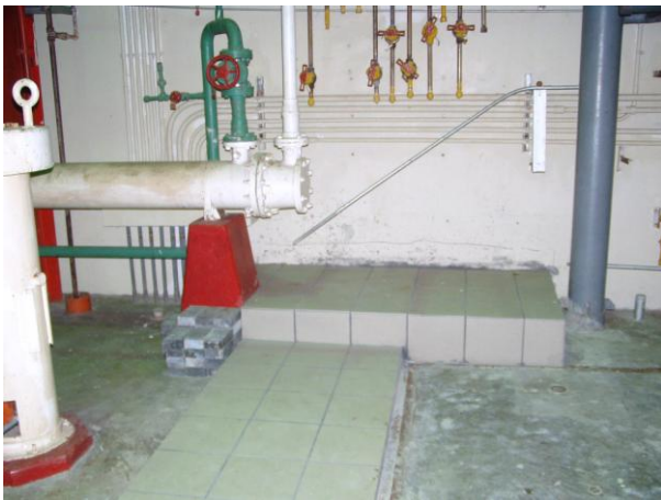
Figures 18a and 18b. Main Level – Tile, Concrete, and Lead Bricks Covering “Hot Spot” on North Side (Adjacent to Sample Locations 27 and 28)
