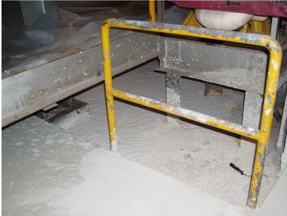
Figure 25. Basement Level – Lowest Point in Basement Shows No Recent Signs of Flooding (Dry, Cracked Silt/Mud is Visible)
