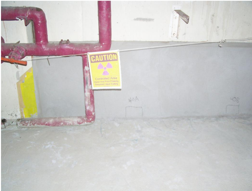
Figure 9. Basement Level – Survey Locations 40A and 40B
