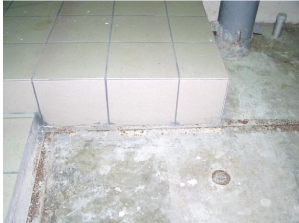
Figures 18a and 18b. Main Level – Tile, Concrete, and Lead Bricks Covering “Hot Spot” on North Side (Adjacent to Sample Locations 27 and 28)
