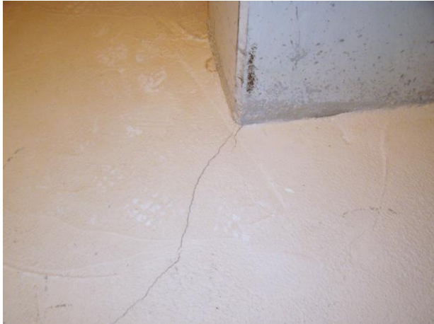
Figure 8a and 8b. Basement Level – Surface Cracks in Concrete Cover (Typical)
