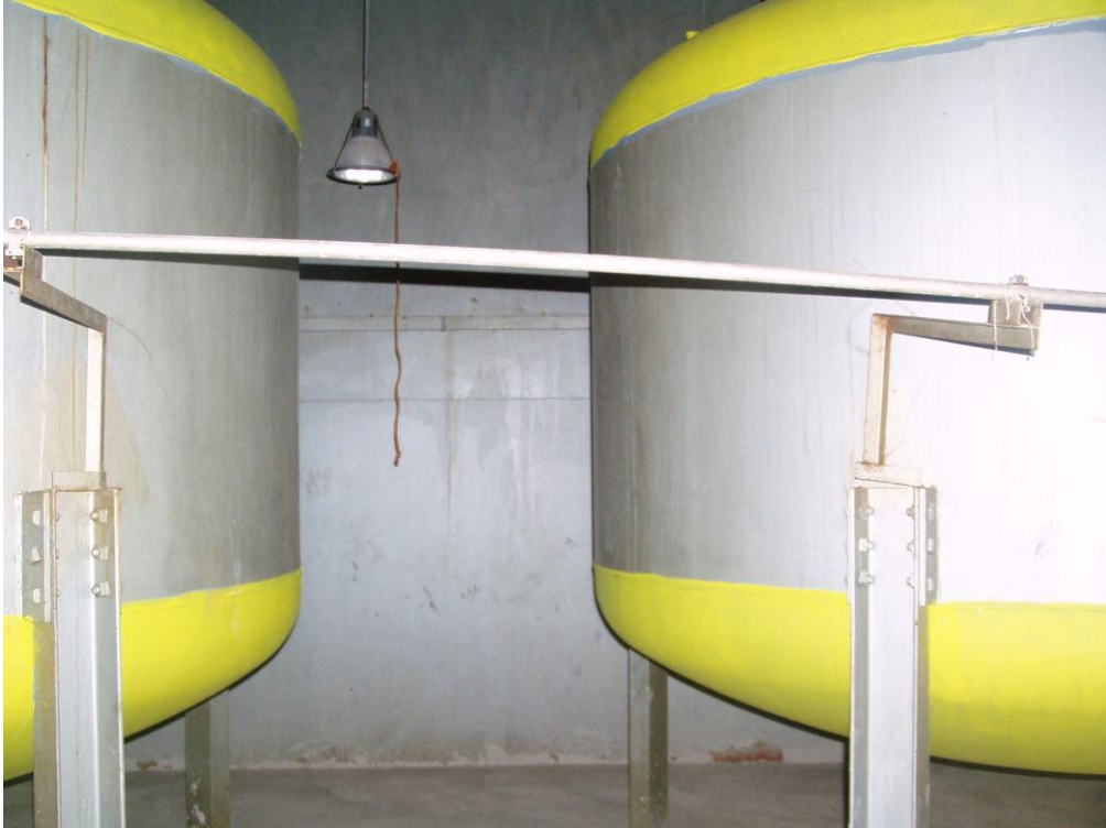
Figure 5. Basement Level – Retention Tanks 1 and 2
