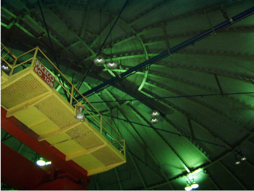
Figure 13. Interior View of Dome “Shell” and Crane Catwalk
