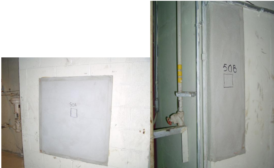
Figures 11a and 11b. Basement Level – Survey Locations 50A and 50B
