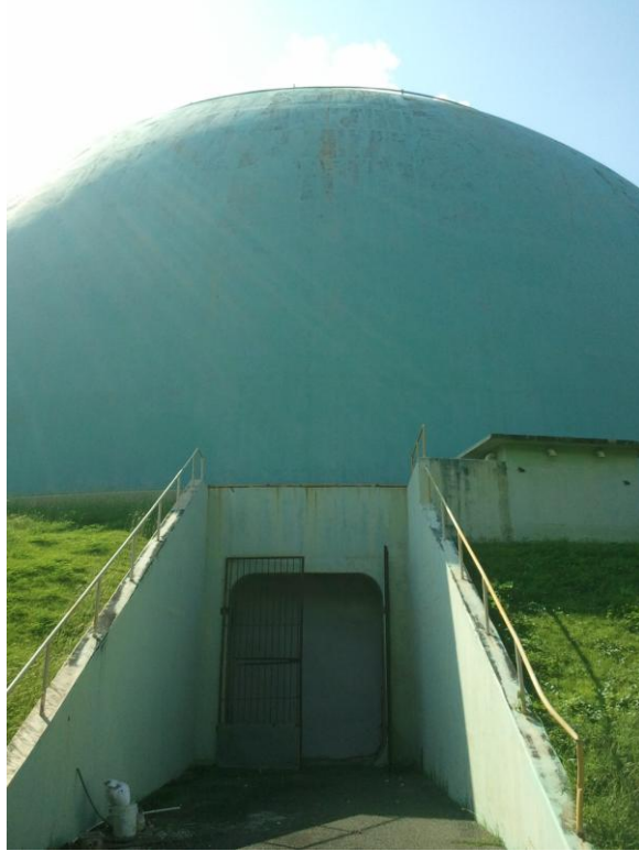
Figure 32. Exterior Structure – Basement Loading Access Door
