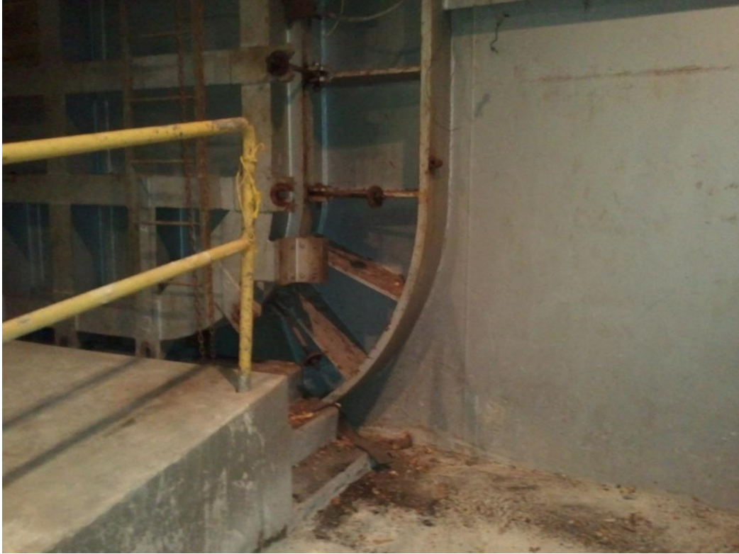
Figure 22. Basement Level – Loading Access Door (No Signs of Leak through Door)
