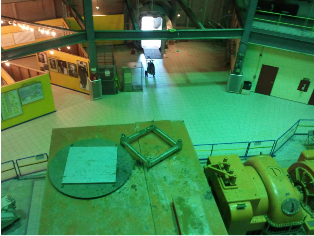
Figure 7. Main Level (North Side) – Overhead View
