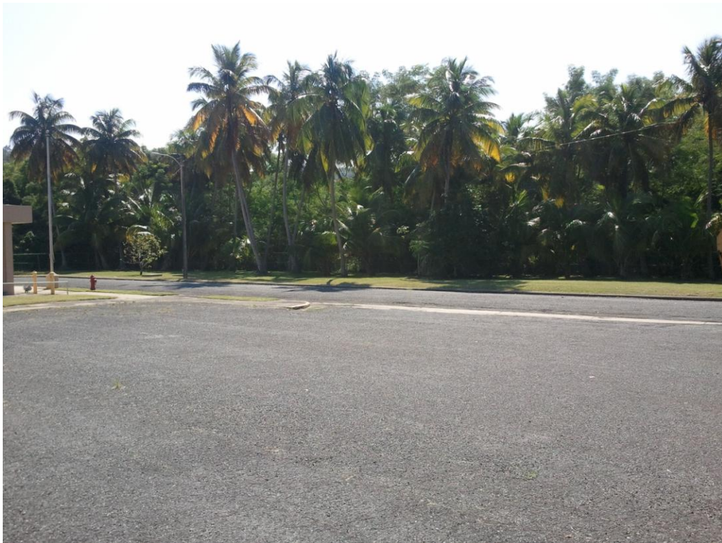
Figure 37. Fence – South Side
