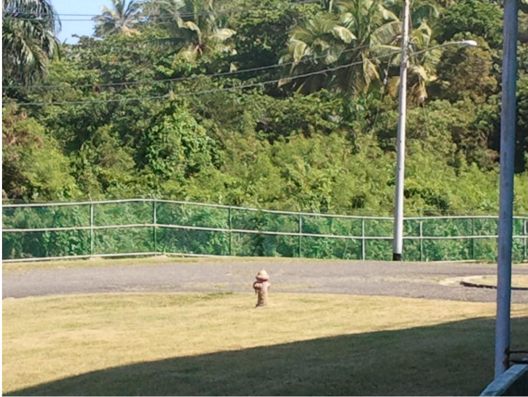
Figure 36. Fence – North Side
