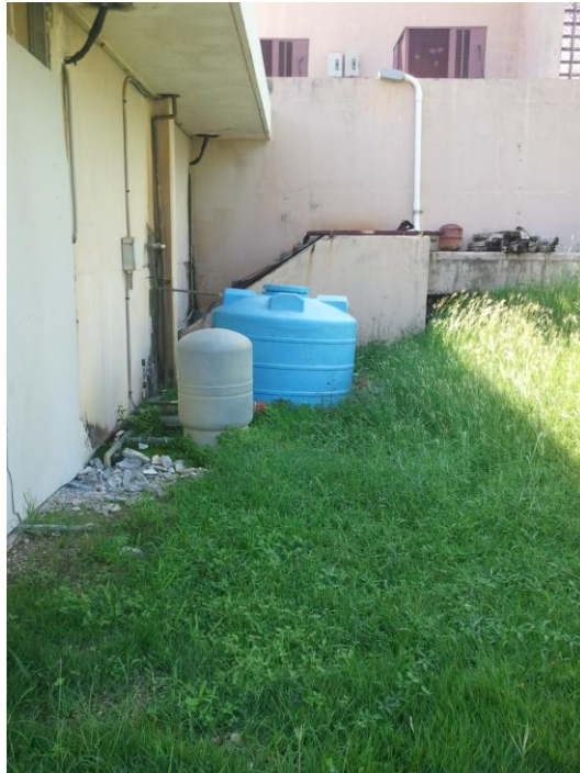
Figure 39. Ancillary Building – Previous Water Tank Overflow has been Shut-Off (No Standing Water)
