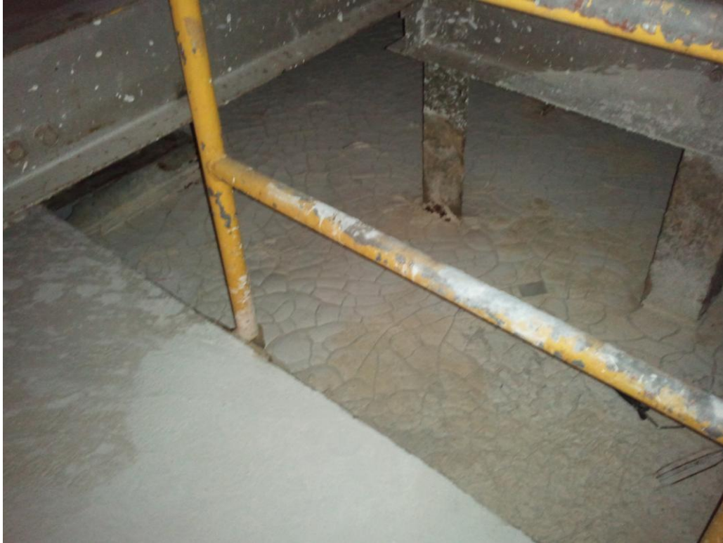
Figure 20. Basement Level – Lowest Point in Basement with No Standing Water
