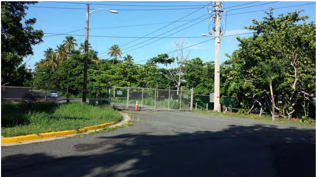
Figure 31. Security – Main Gate in Good Working Condition (Manual Open/Close)
