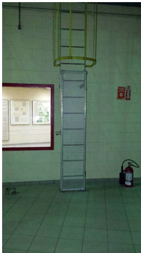
Figure 12. Main Level – Locked and Controlled Access to South Mezzanine
