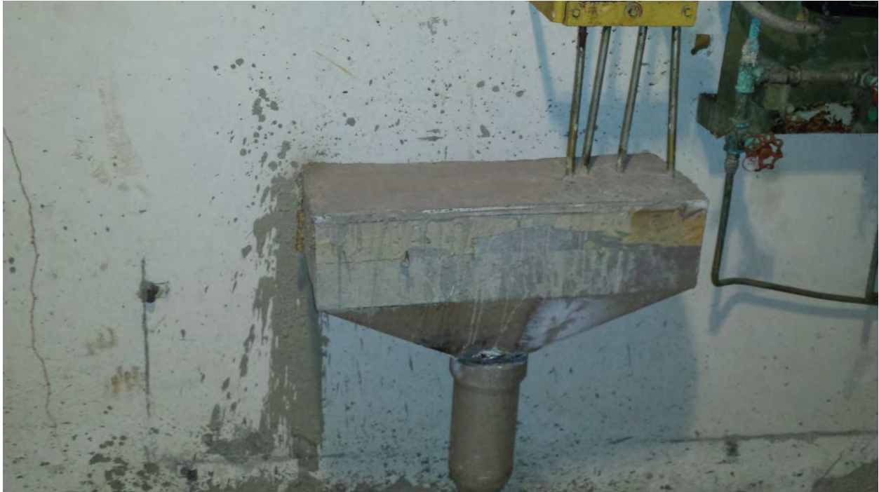
Figure 17. Basement Level – Concrete Filled Sink
