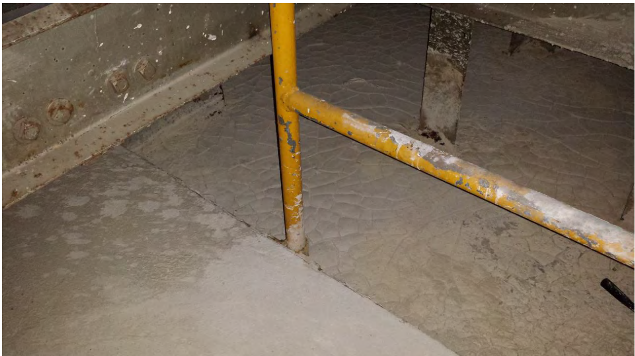
Figure 18. Basement Level – Lowest Point in Basement with No Standing Water
