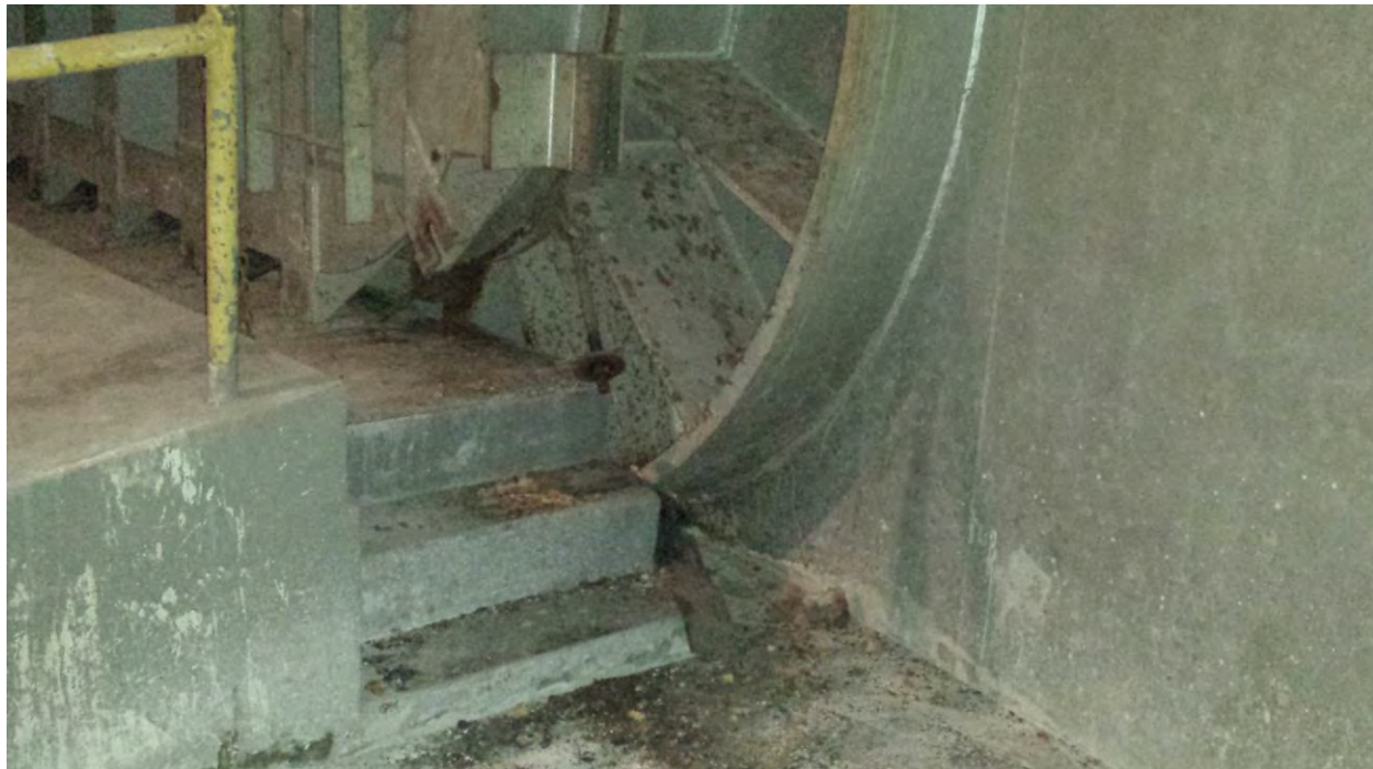
Figure 14. Basement Level – Bay Door (No Signs of Rain Water Infiltration)
