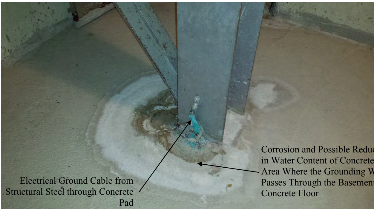
Figure 22. Basement Level – Corrosion Issues on Concrete Floor near Sample Locations 50A and 50B
