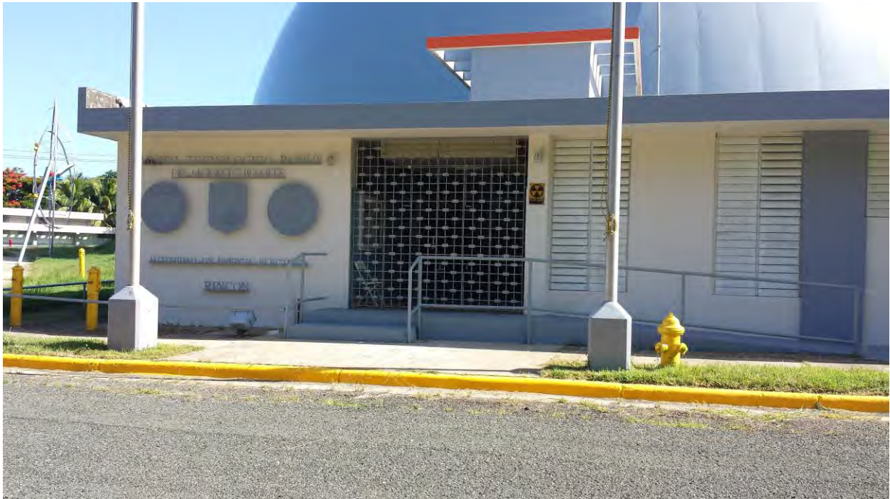
Figure 23. Dome Structure – Exterior With New Protective Coating and Paint
