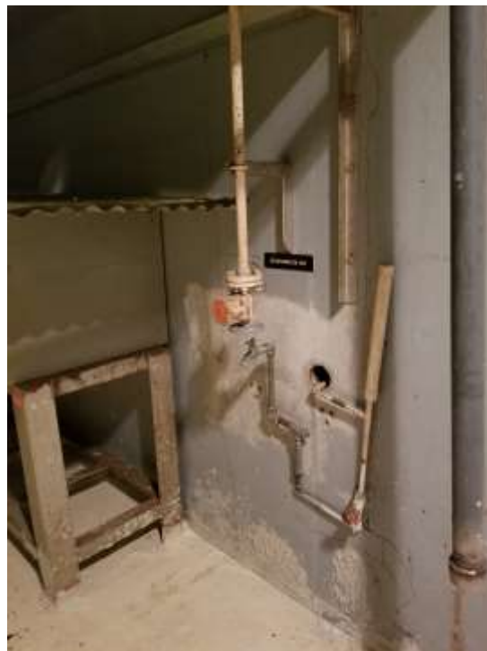
Figure 29. Basement Level – Painted Flange (Engineering Controls) at Former Decontamination Sink Location
