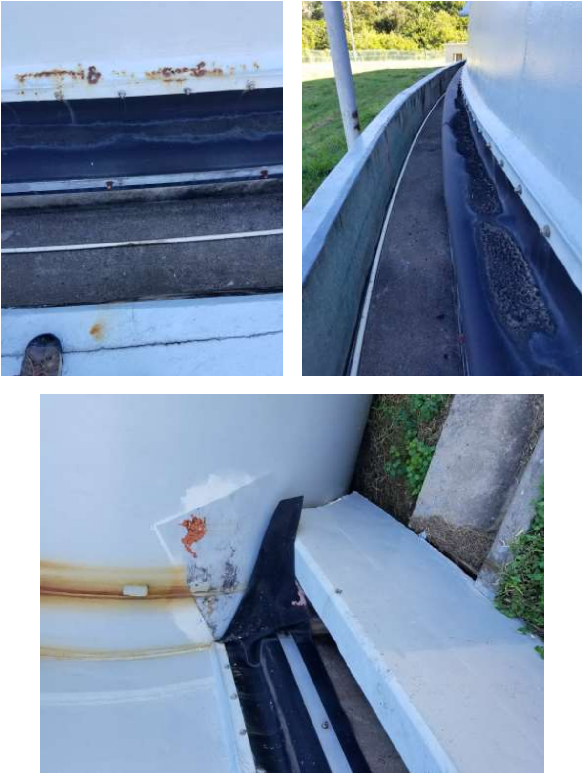
Figure 37. Dome Structure – Flexible Gasket/Seal – Dome Perimeter
