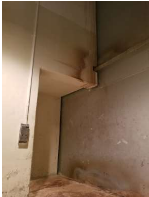
Figure 25. Basement Level – Beneath North Entrance Air Lock (No Signs of Recent Water Infiltration – Older Stains Persist)
