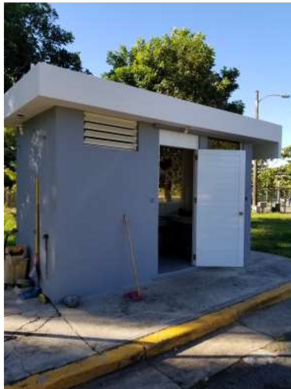
Figure 40. Ancillary Buildings and Structures – Guard Shack
