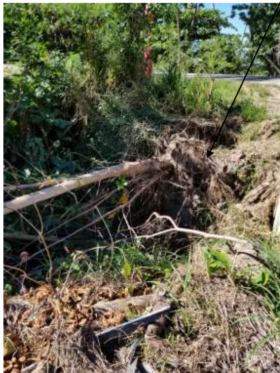
Figure 35. Dome Structure – Drainage Outfall Points and Ditches (Under Main Access Road –East side of road – right pipe filled with sand and debris)
