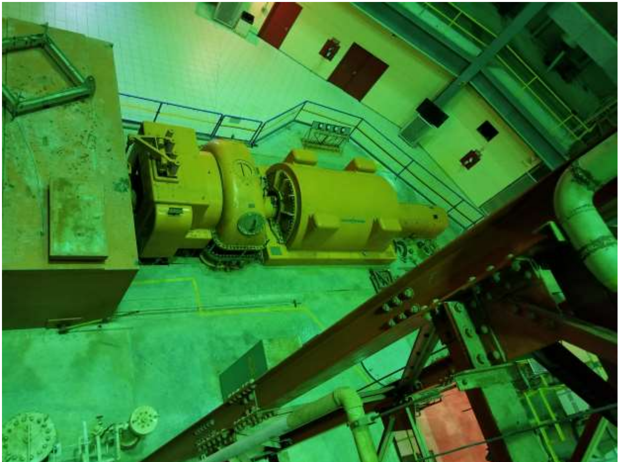
Figure 8. Main Level (North/Northeast Side) – Overhead View
