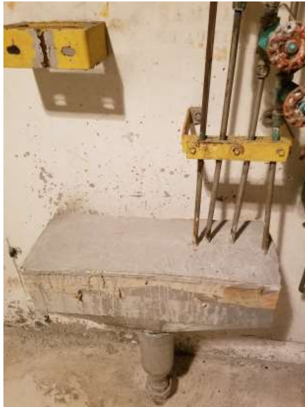
Figure 26. Basement Level – Concrete Filled Sink
