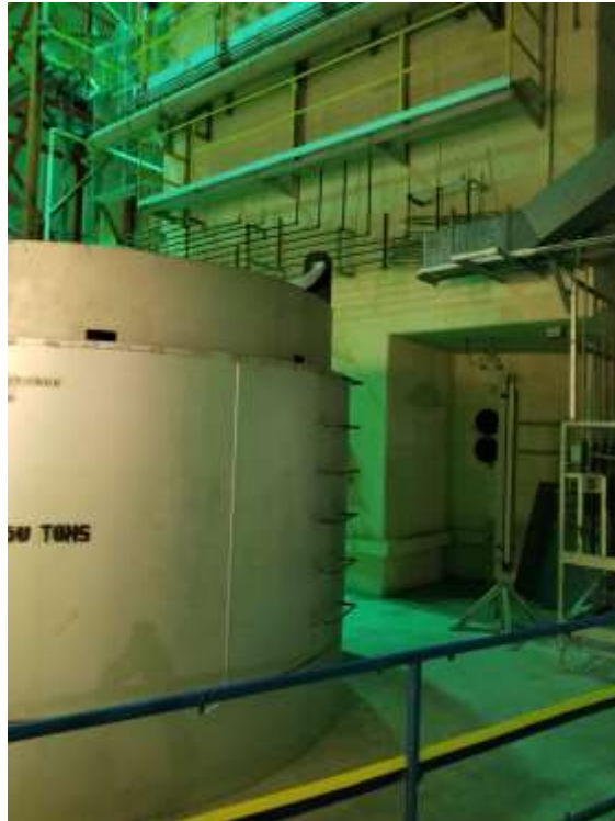
Figure 20. Main Level (Controlled Area) – Northwest Side
