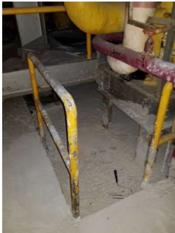
Figure 27. Basement Level – Lowest Point in Basement with No Standing Water
