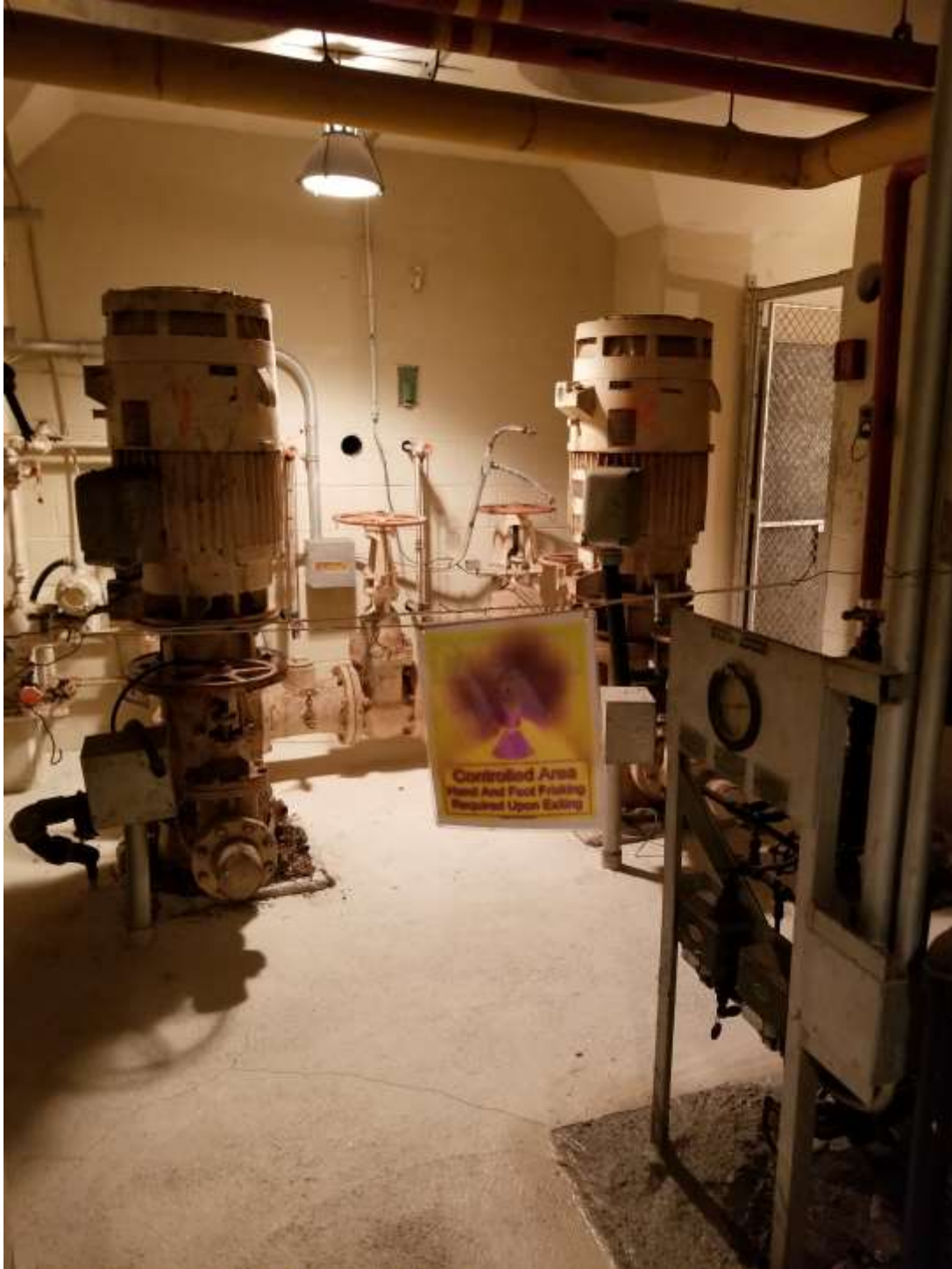
Figure 42. Basement Level – Temporary Posting
