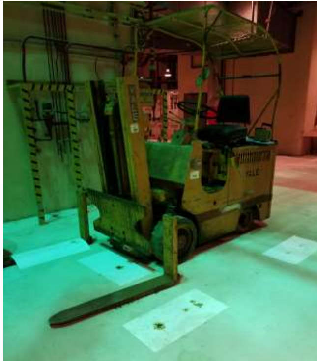
Figure 24. Basement Level – Oil/Lubricant Spots on Basement Floor from Overhead Equipment
