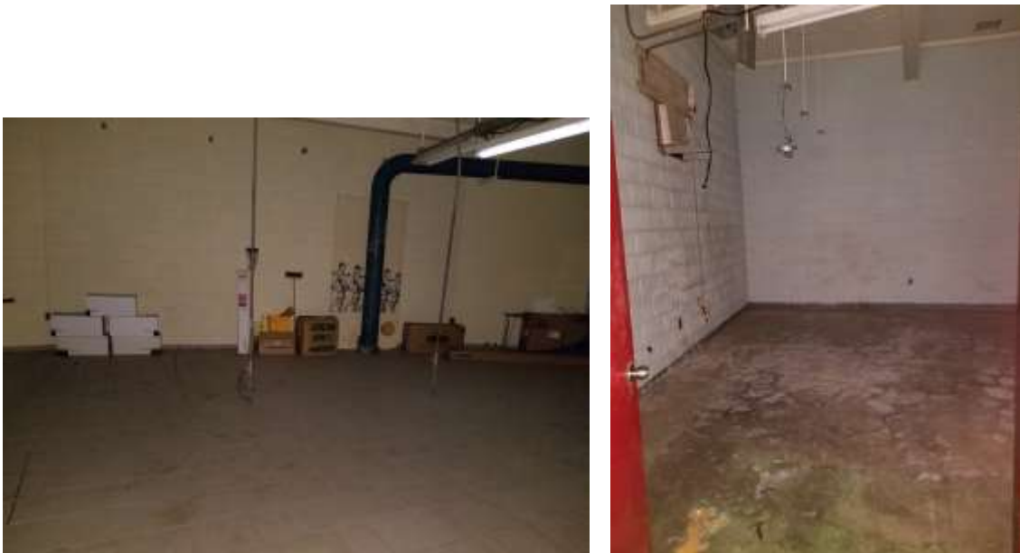
Figure 14. Main Level (Museum Area) – Locked and Controlled Access to Machine Shop (Left) and Electrical Shop (Right) Former File Storage
