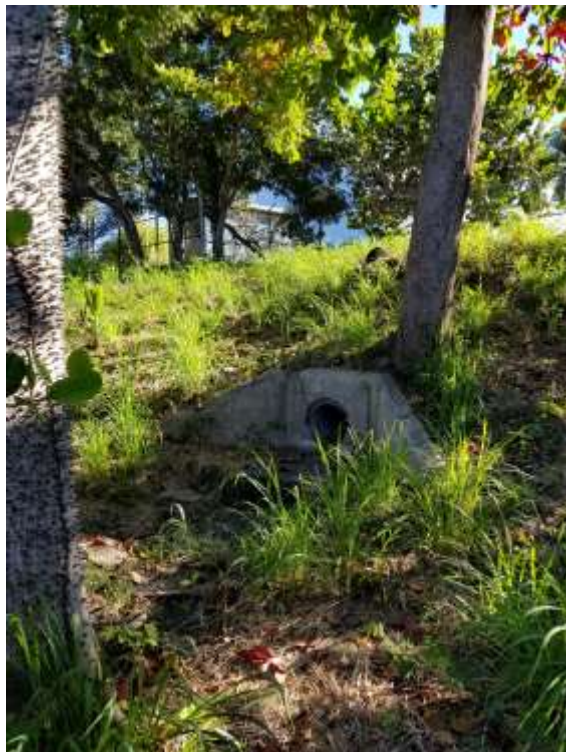
Figure 34. Dome Structure – Drainage Outfall Points and Ditches (Southern Outfall)
