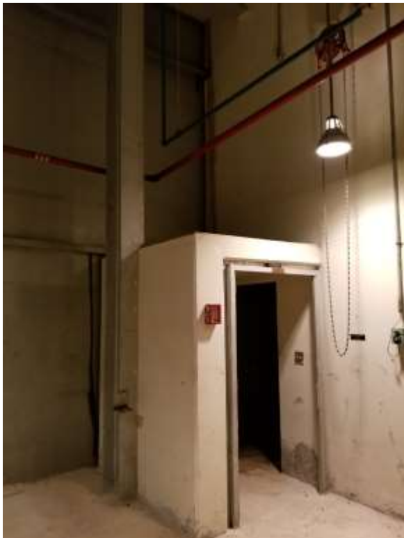
Figure 25. Basement Level – Beneath North Entrance Air Lock (No Signs of Recent Water Infiltration – Older Stains Persist)
