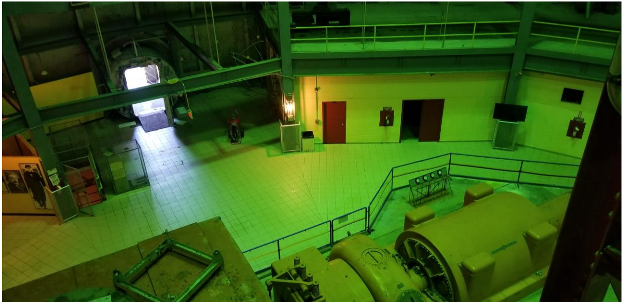
Figure 8. Main Level (North/Northeast Side) – Overhead View
