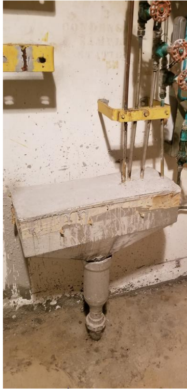
Figure 26. Basement Level – Concrete Filled Sink
