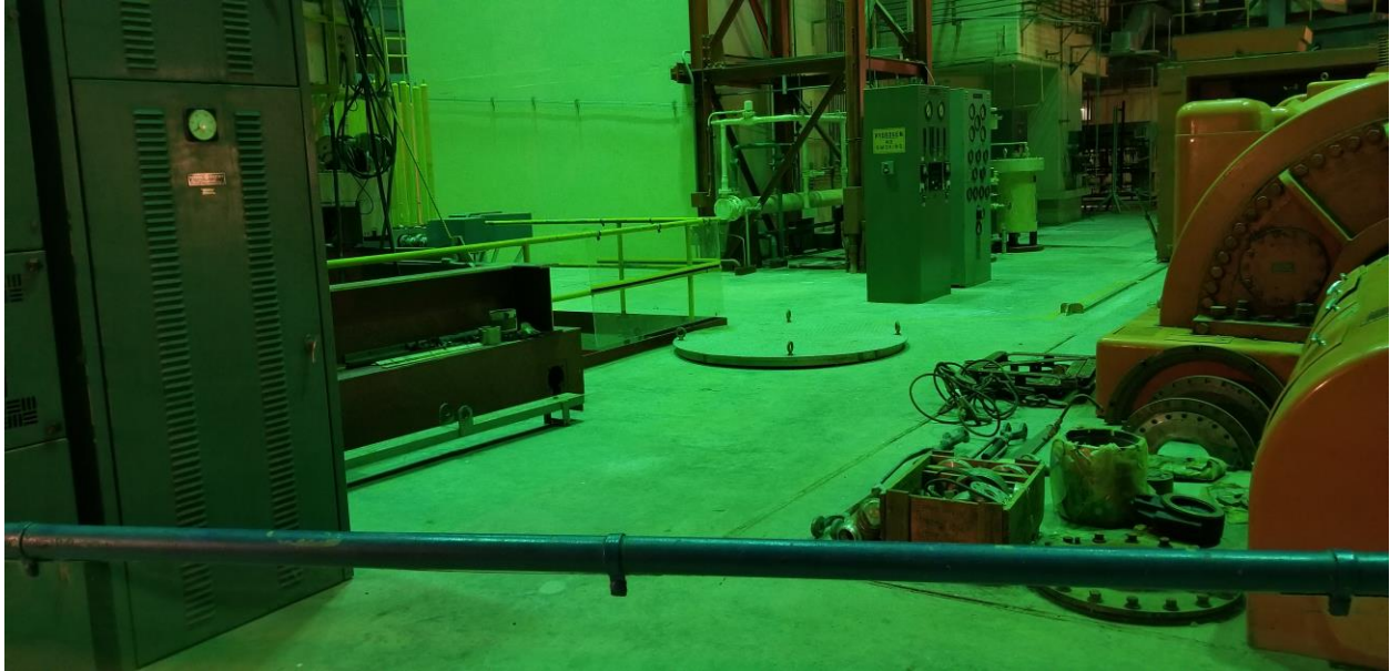
Figure 17. Main Level (Controlled Area) – East Side
