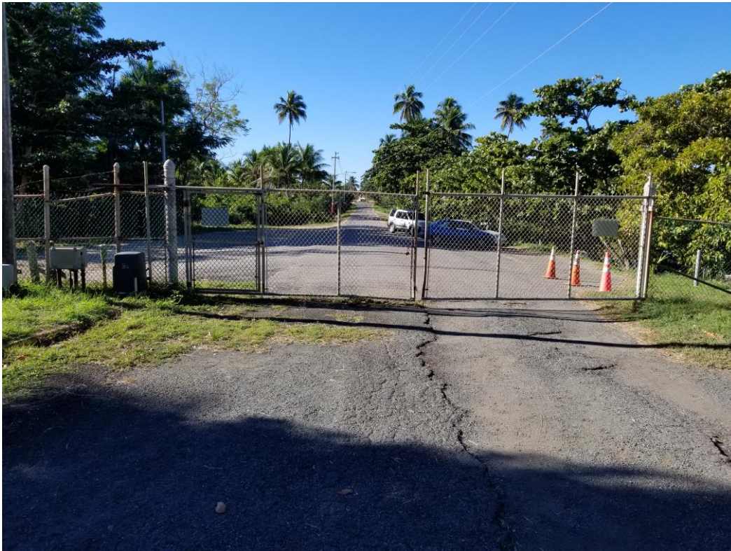
Figure 39. Security – Main Gate in Good Working Condition (Manual Open/Close)
