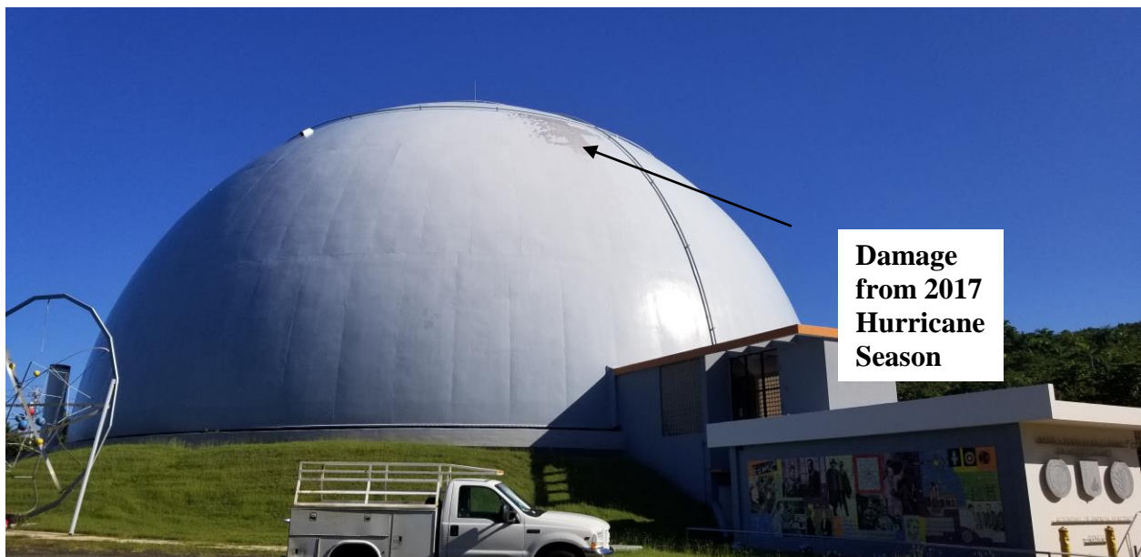
Figure 32. Dome Structure – Exterior with Protective Coating and Paint
