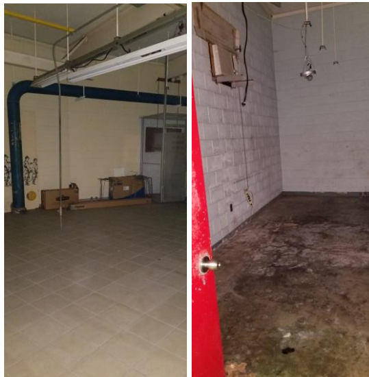
Figure 14. Main Level (Museum Area) – Locked and Controlled Access to Machine Shop (Left) and Electrical Shop (Right) Former File Storage
