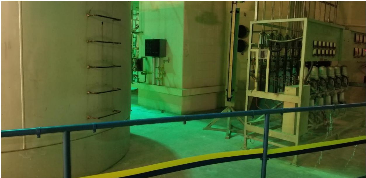
Figure 20. Main Level (Controlled Area) – Northwest Side
