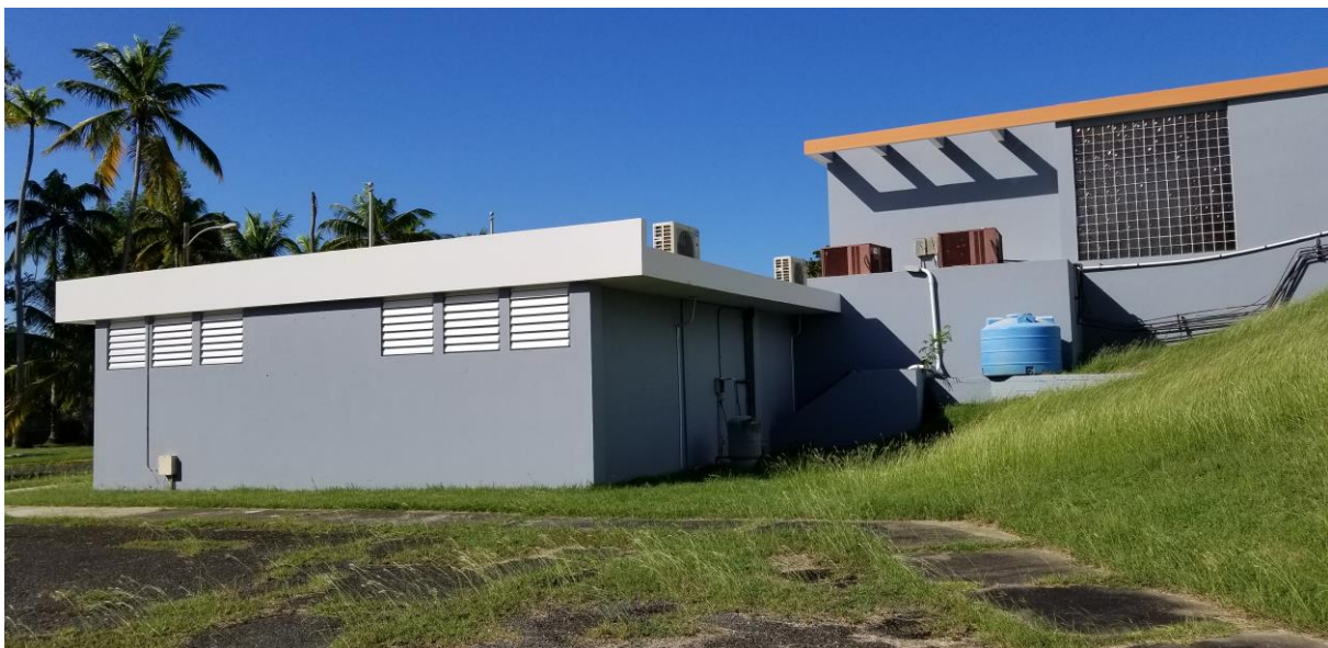
Figure 40. Ancillary Buildings and Structures – Bathroom and Museum Area at South Entrance
