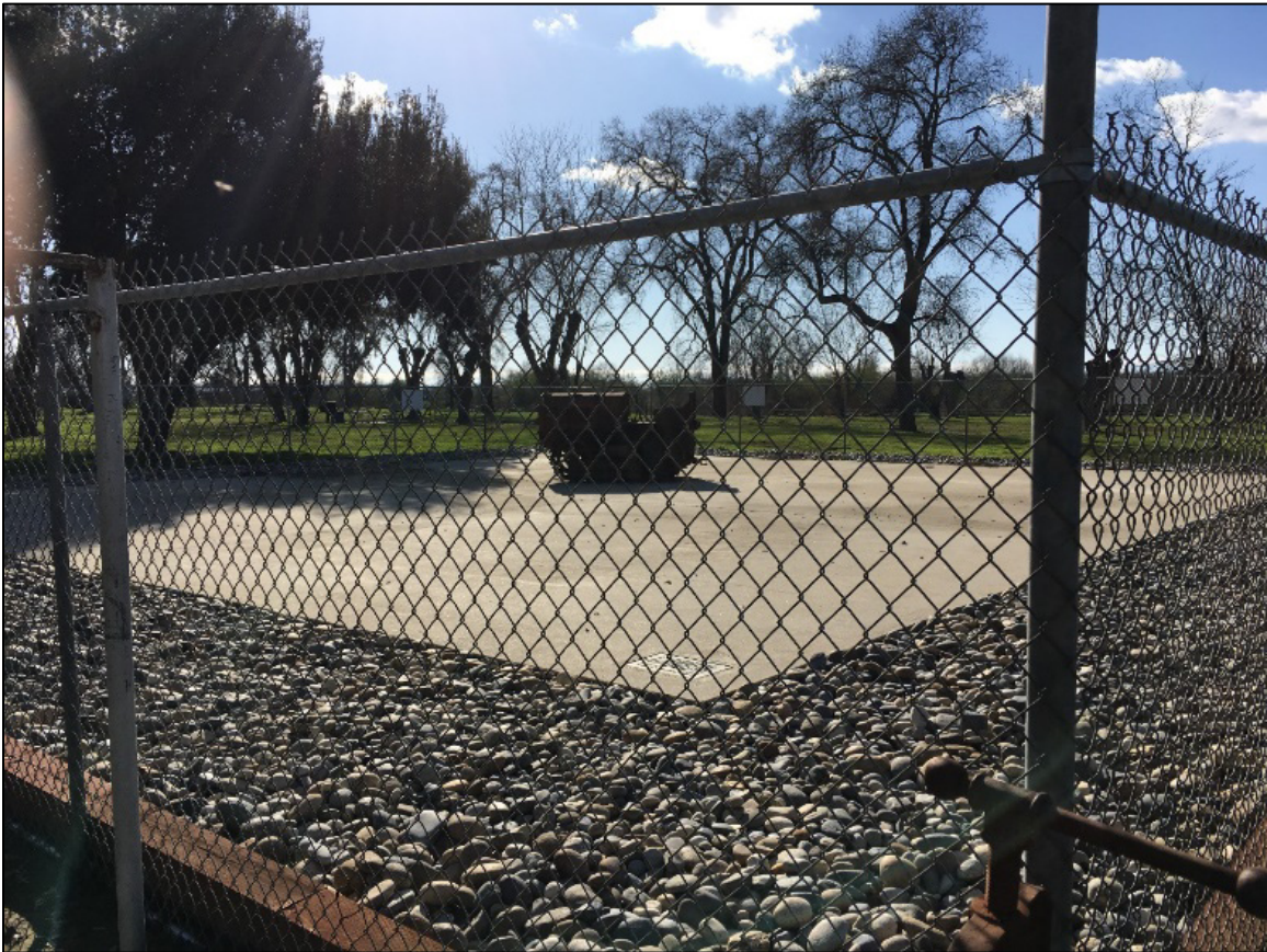
Figure 4. Burris Park Site After 2018 Maintenance Activities, Looking West, February 2019
