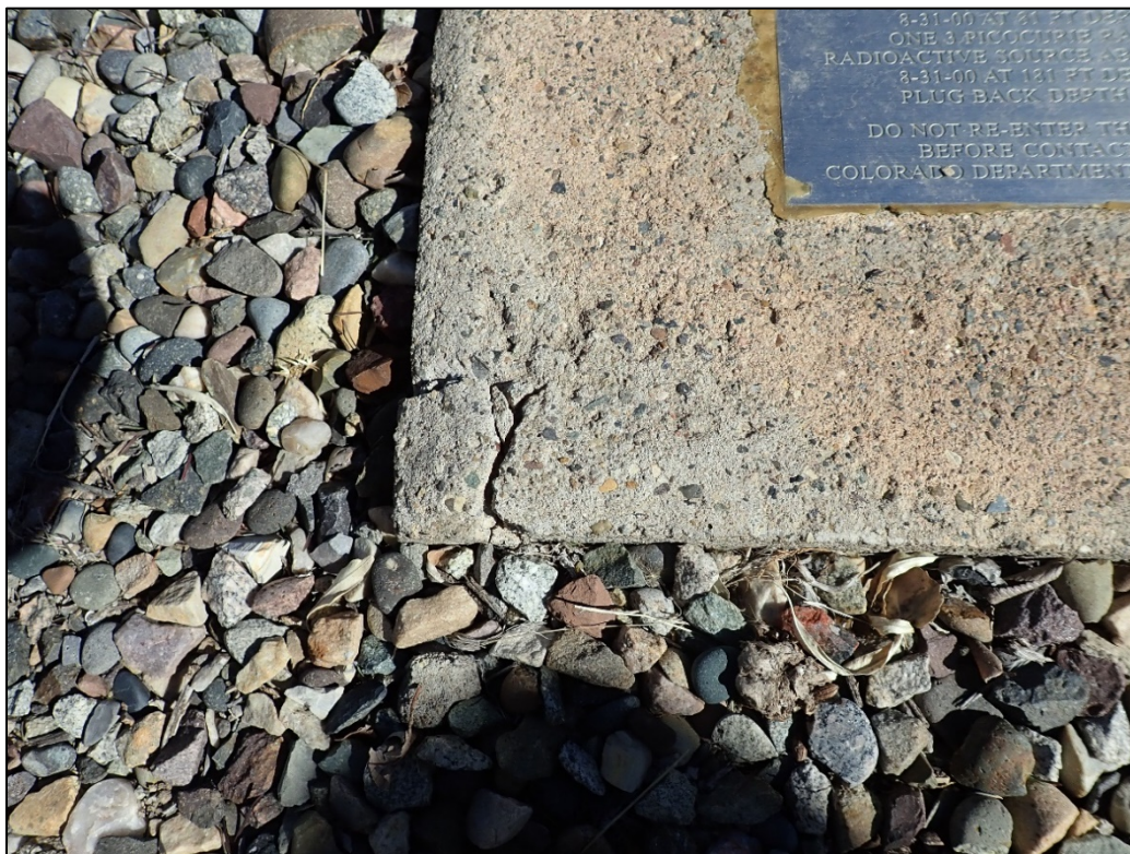
PL-6. Broken Concrete Pad Around Decommissioned Borehole Containing Radium Foil
