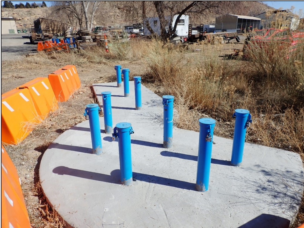
PL-4. AS&T Monitoring Well Gallery
