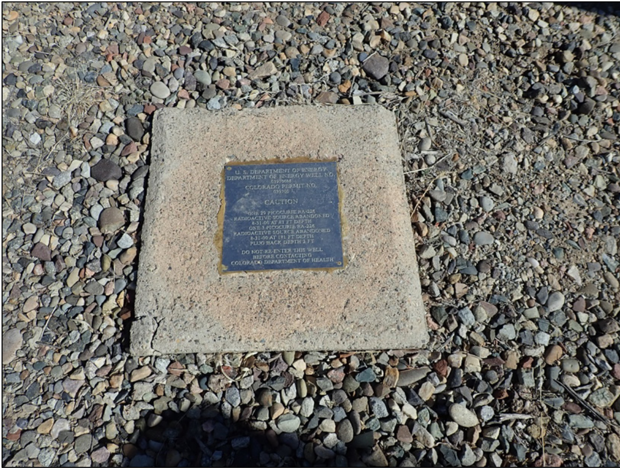
PL-7. Decommissioned Borehole Containing Radium Foil
