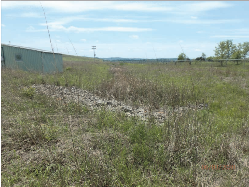
P6030001 West Outer Drainage Cell 1 (looking south)
