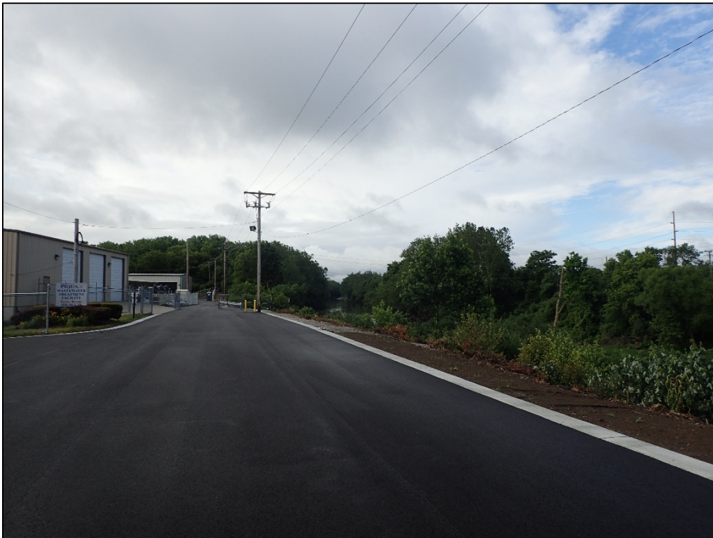
PL-2. New Paving to Water Treatment Plant
