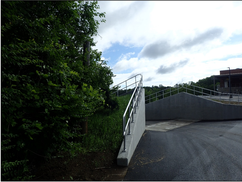
PL-3. New Retaining Wall
