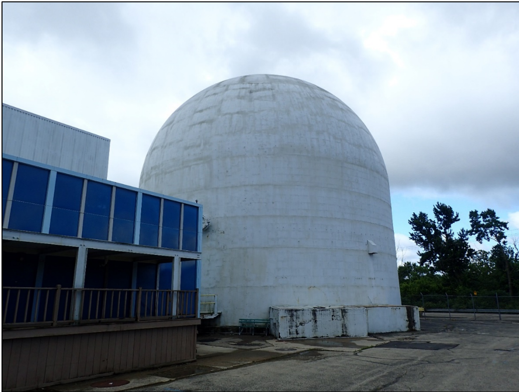
PL-1. Containment Building
