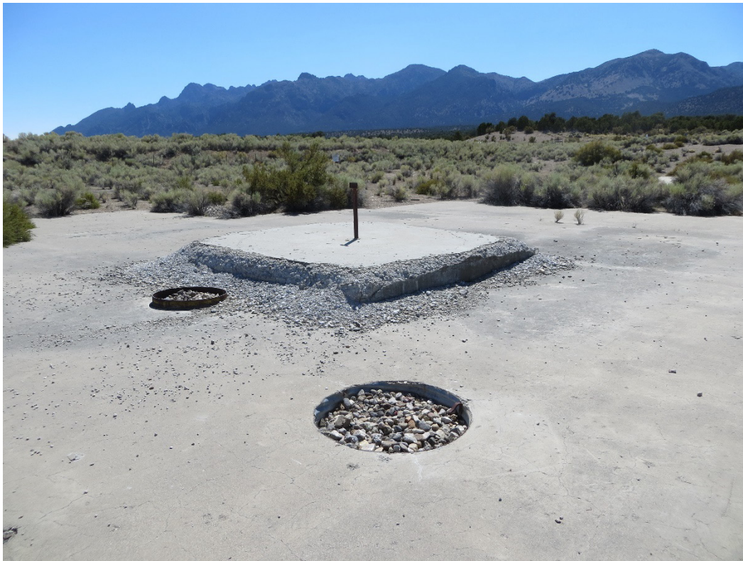
Figure A-3. Concrete Cap That Covers the UC-4 Borehole (August 2020)
