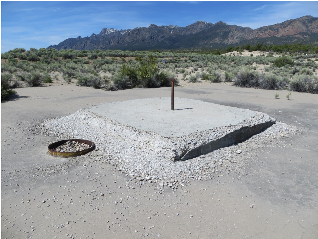
Figure A-2. Concrete Cap That Covers the UC-4 Borehole (June 2019)
