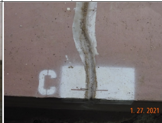
Figure 21. Sealed Crack at Edge of Red Concrete
