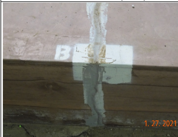
Figure 20. Sealed Crack at Edge of Red Concrete
