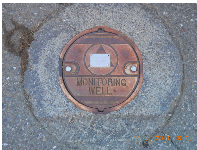
Well UCD1-054 – New bolts Installed in Vault Lid (Photo No. 4539)
