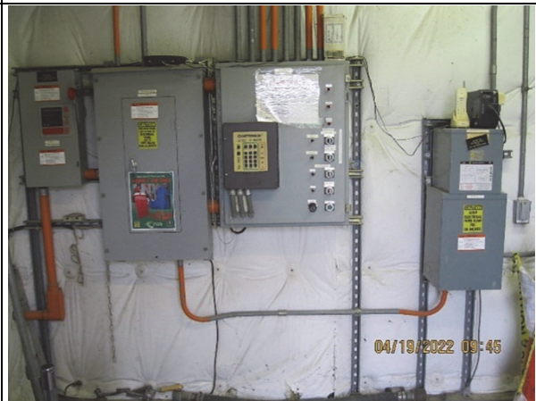
Figure 38. Controls for the Pump and Treatment System in Building 300
