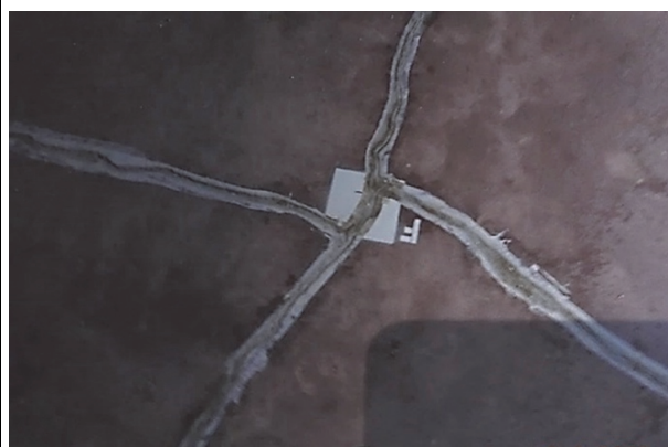
Figure 16. Close up of Sealed Crack in the Red Concrete (1C-10)
