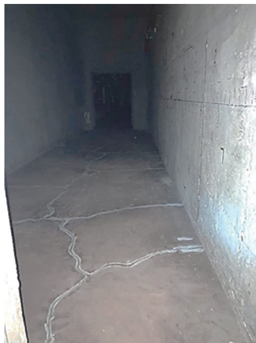
Figure 20. Sealed Crack in Room 59 (1C-21)
