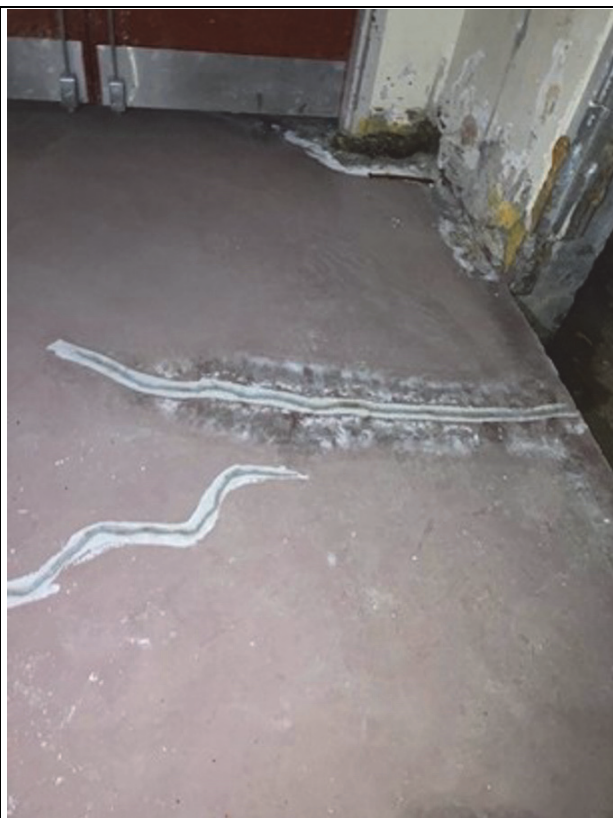
Figure 18. Sealed Cracks in Red Concrete Floor at 1C-10 Outside of T-57 (1C-11)
