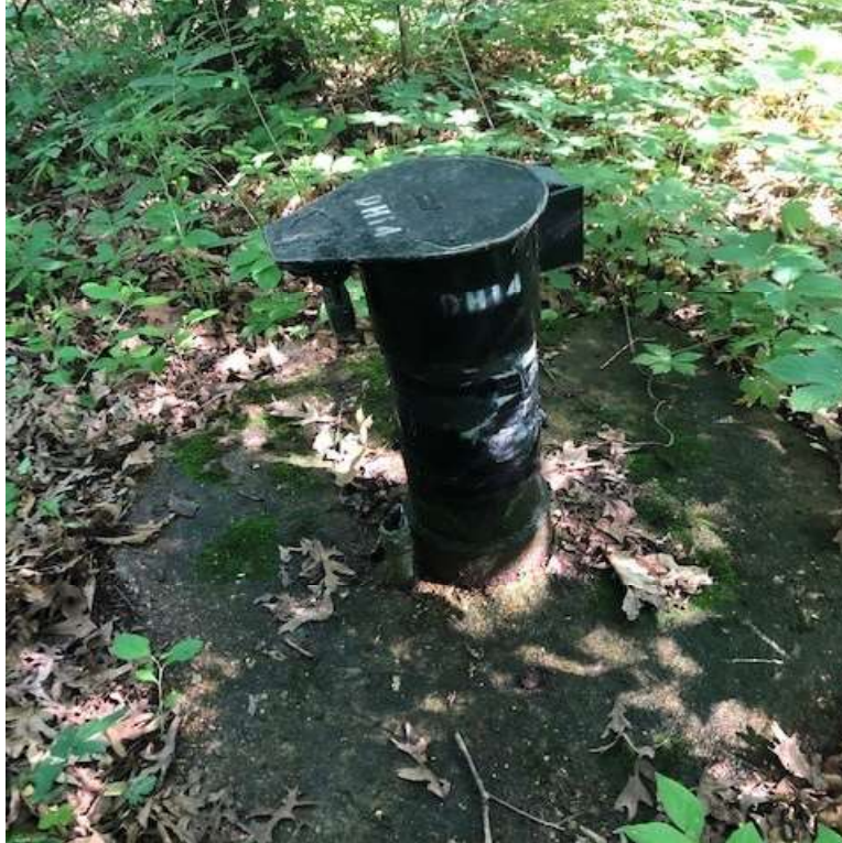
P13 - Monitoring Well DH14 at Red Gate Woods
