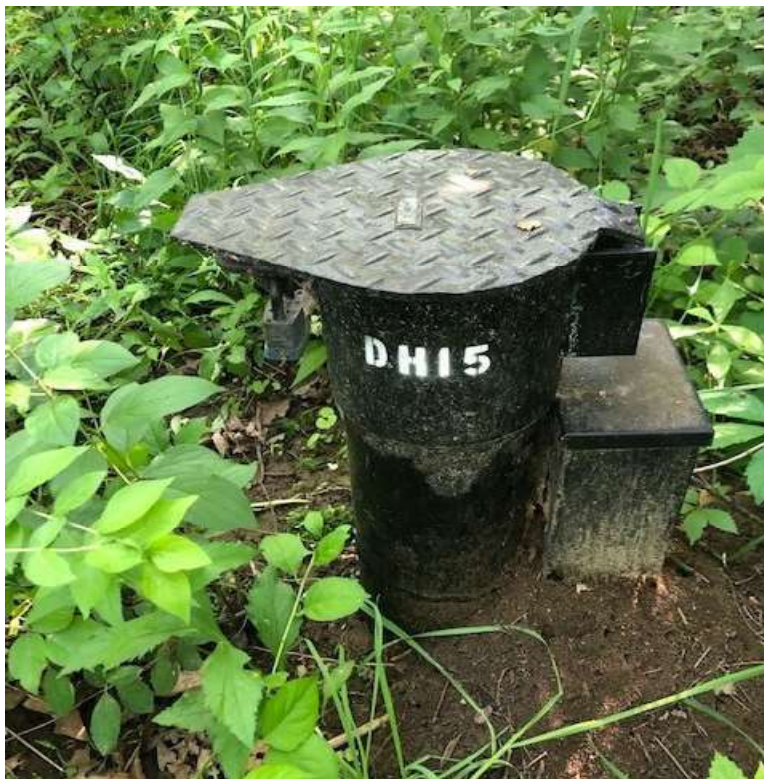
P14 – Monitoring Well DH15 at Red Gate Woods
