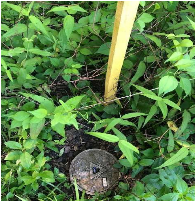
P02 – Monitoring Well BH06 at Plot M
