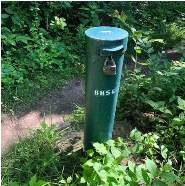
P09 – Monitoring Well BH56 at Site A
