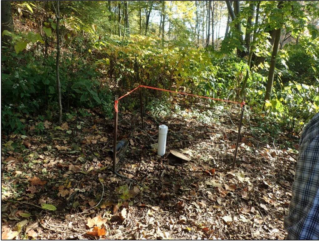
PL-3. New Pipe Installed at Boundary Monument BM1
