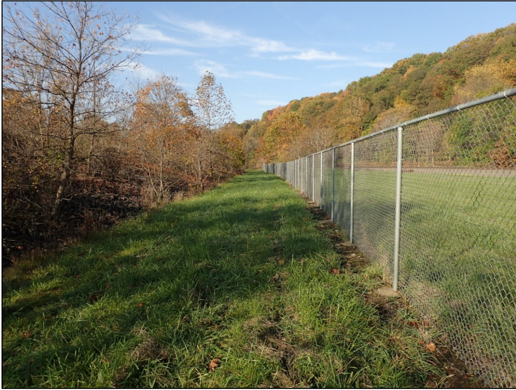
PL-1. Fence Line along Northwest Side of Disposal Cell
