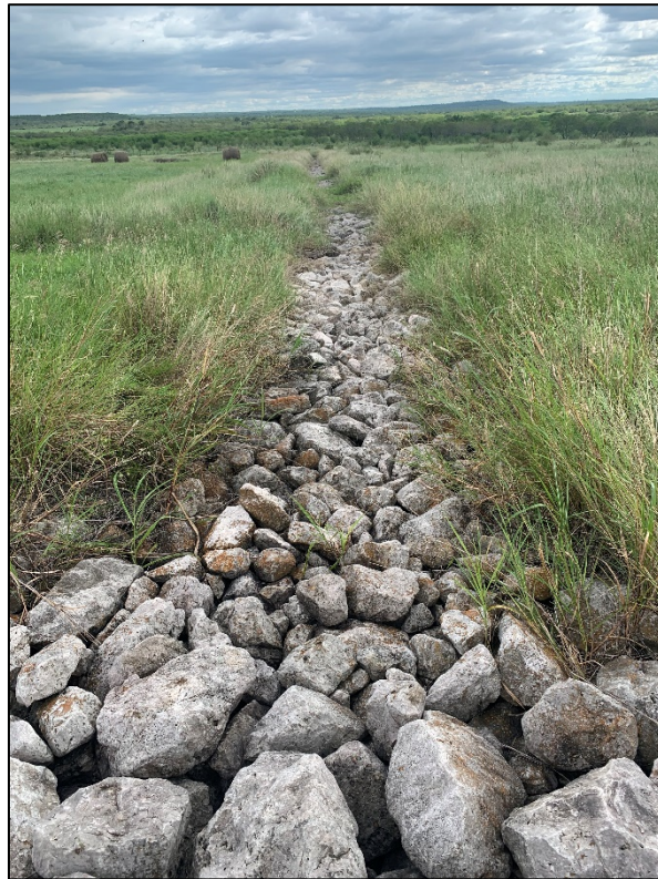
PL-4. Rock Drain on South Corner of Disposal Cell
