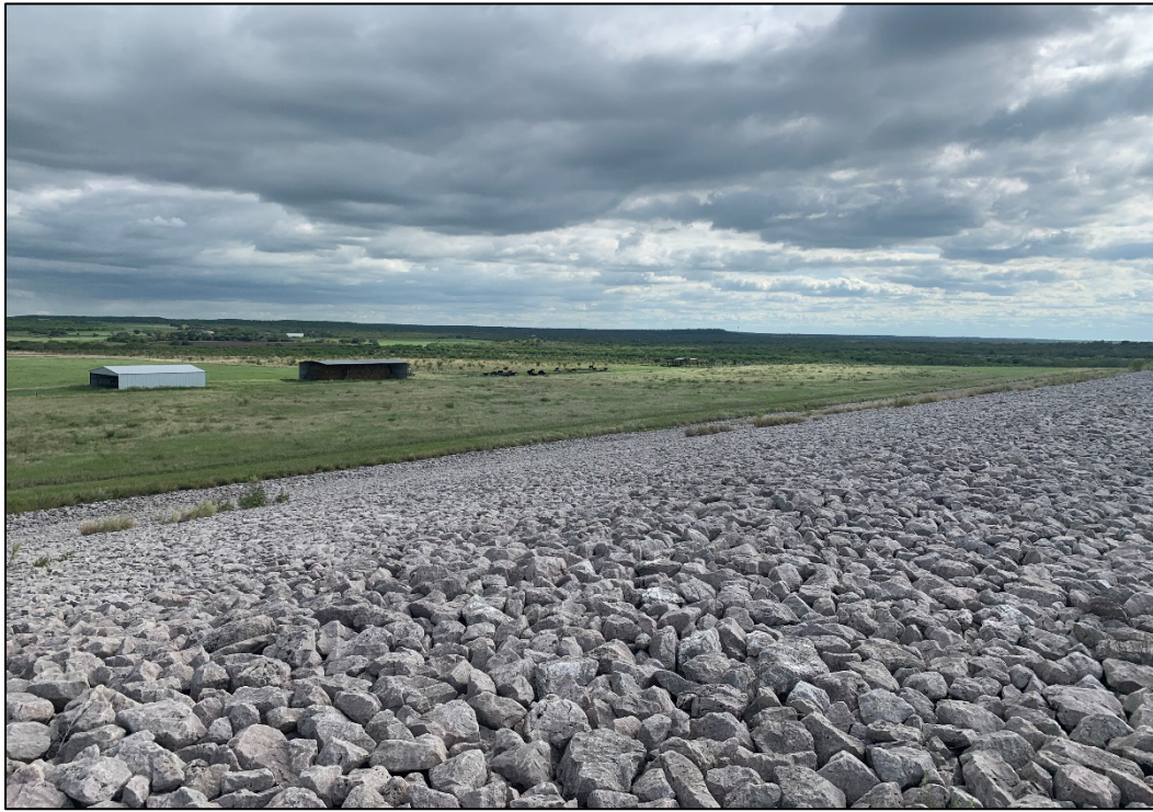
PL-3. South Side of Disposal Cell Side Slope
