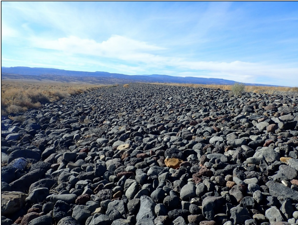
PL-8. South Slope of Disposal Cell
