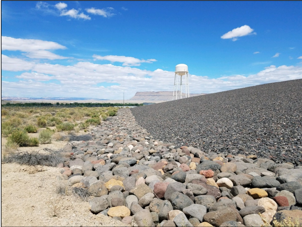
PL-7. Southwest Side Slope (and Apron) of Disposal Cell
