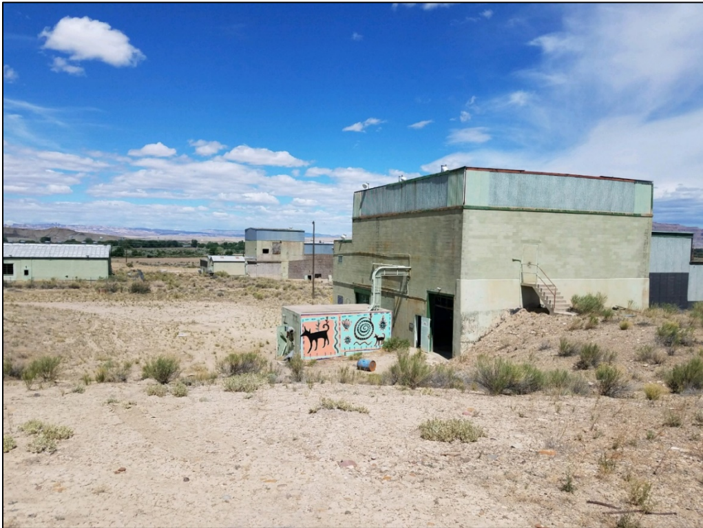
PL-10. Abandoned Mill Buildings
