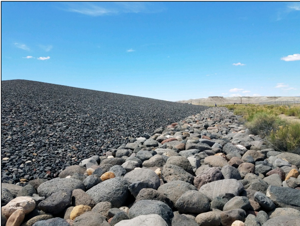
PL-8. Northwest Side Slope (and Apron) of Disposal Cell
