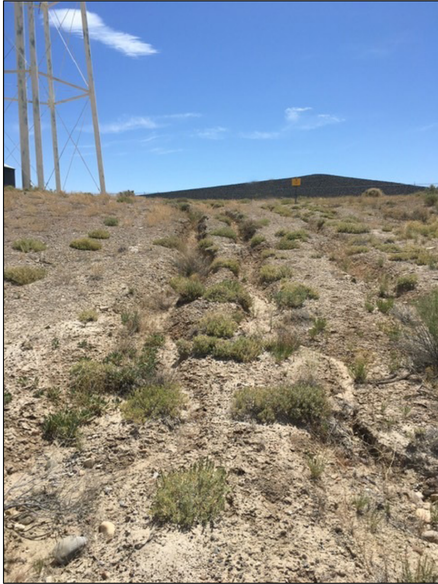
PL-11. Gullies Downslope of Water Tower (Offsite)
