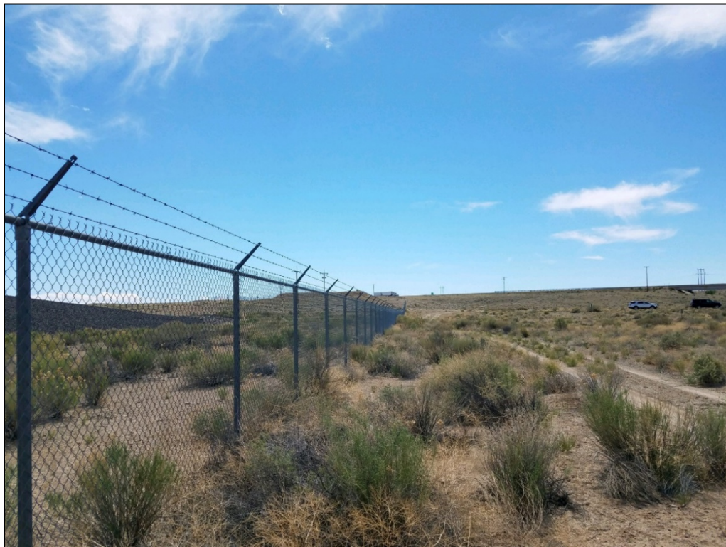
PL-2. Chainlink Security Fence
