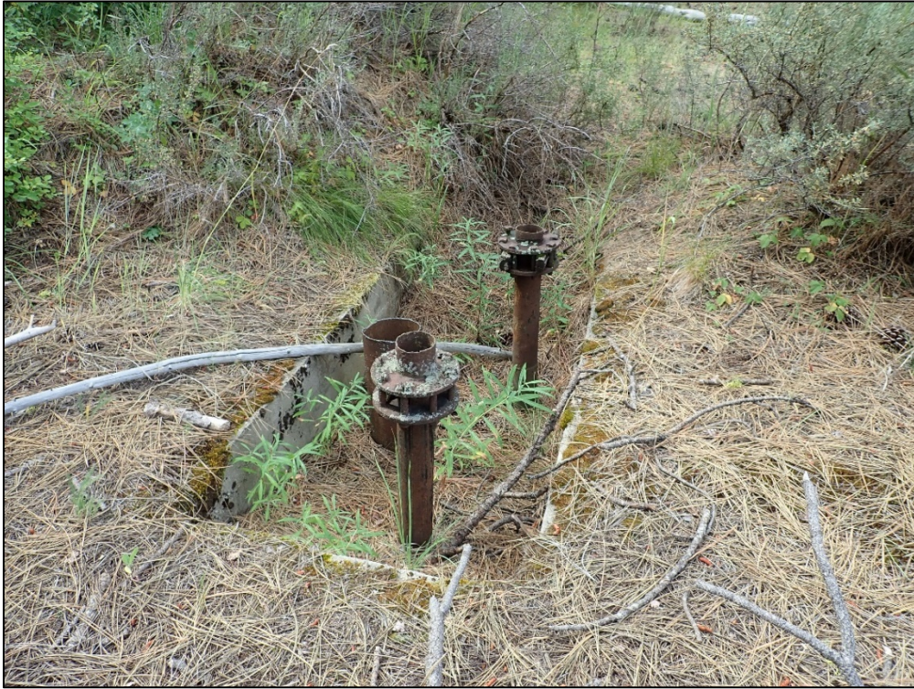
PL-6. Concrete Structure and Water Piping Remains
