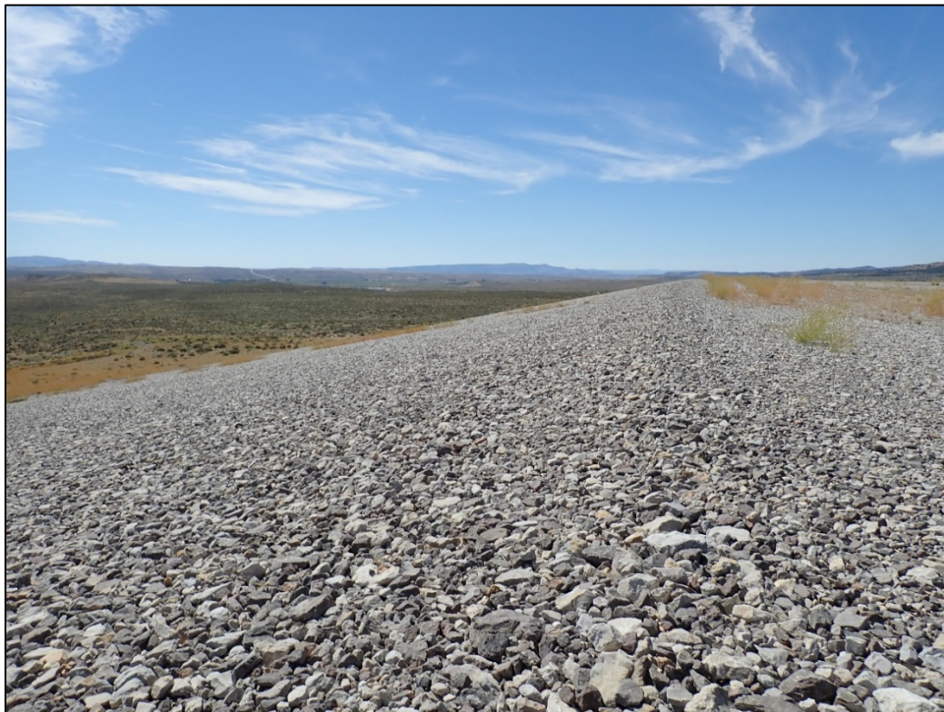
PL-12. Disposal Cell South Side Slope
