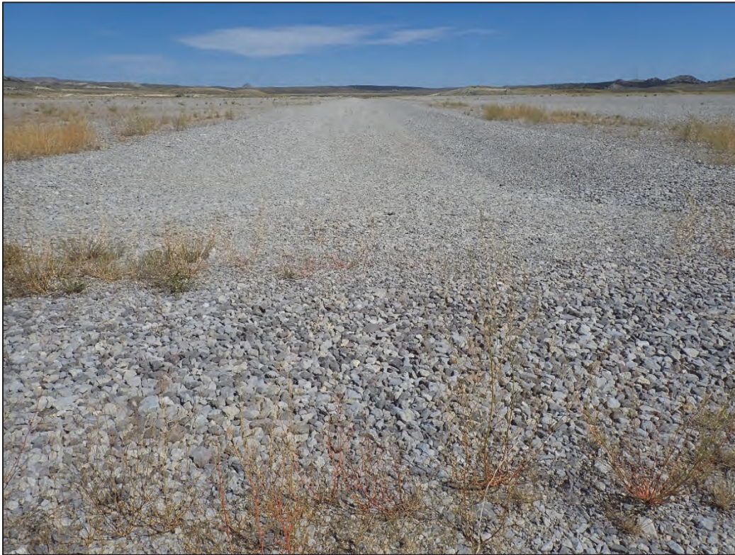
PL-17. Diversion Channel No. 1
