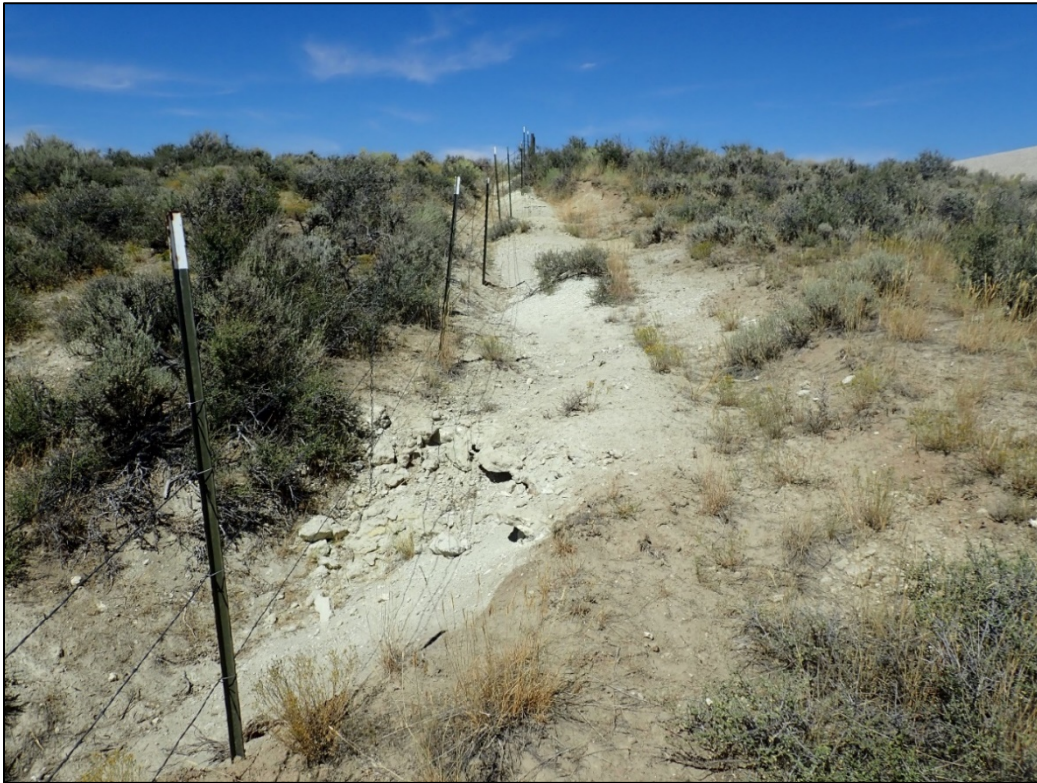
PL-1. Erosion Along Western Perimeter Fence South of Perimeter Sign P7
