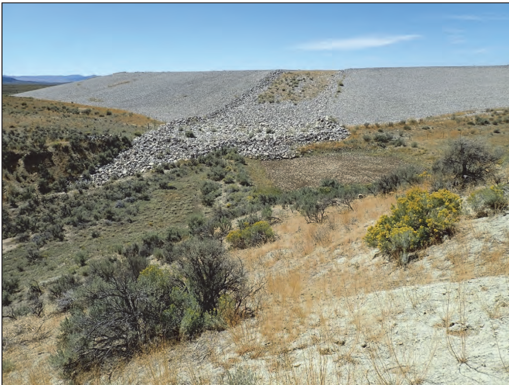
PL-18. Southwest View of Launch Rock Erosion Protection Basin
