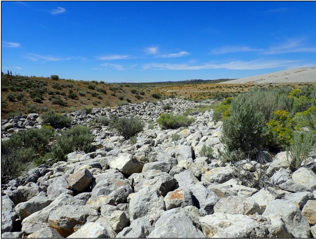
PL-19. Diversion Channel No. 2
