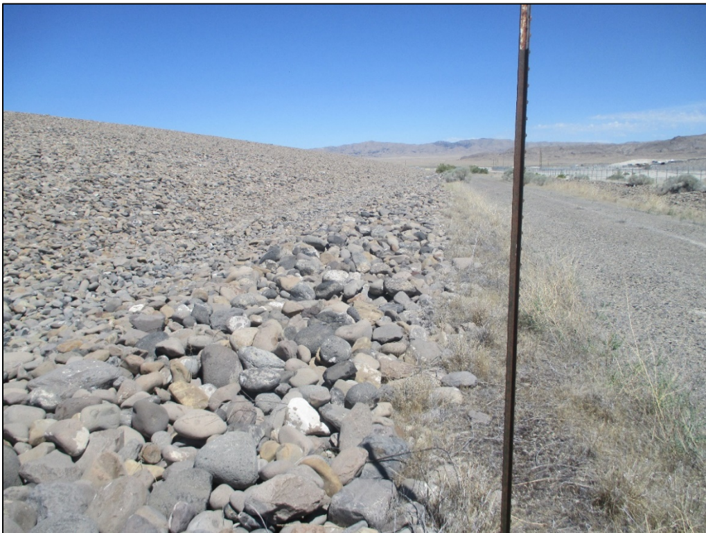
PL-4. Disposal Cell, South Side Toe Drainage
