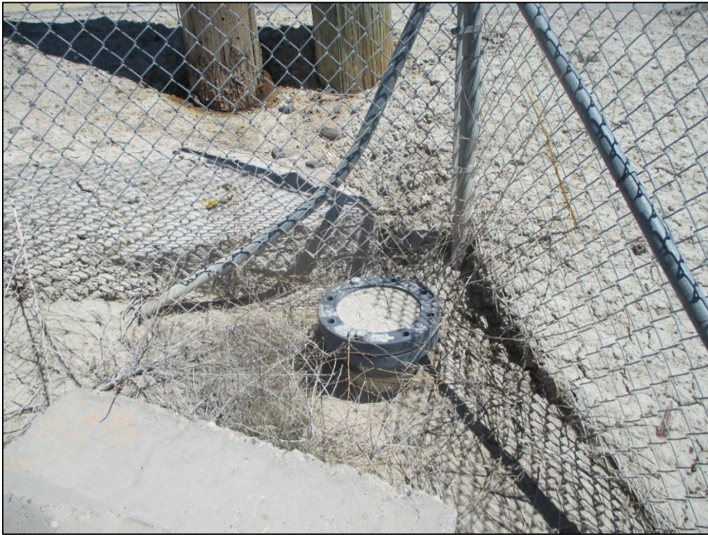
PL-3. Protective Casing on Boundary Monument BM-3
