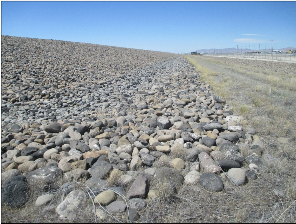
PL-5. Disposal Cell, East Side Toe Drainage
