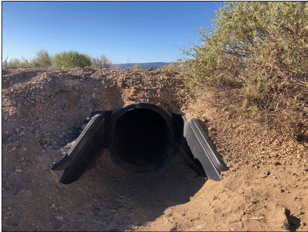
PL-8. Cleaned-Out Culvert
