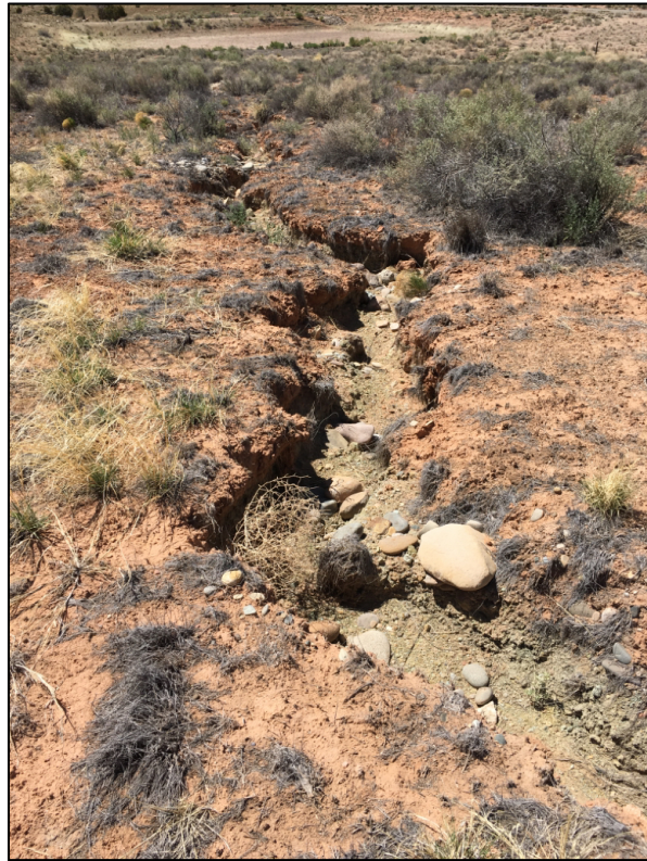
PL-7. Deep Erosional Gully
