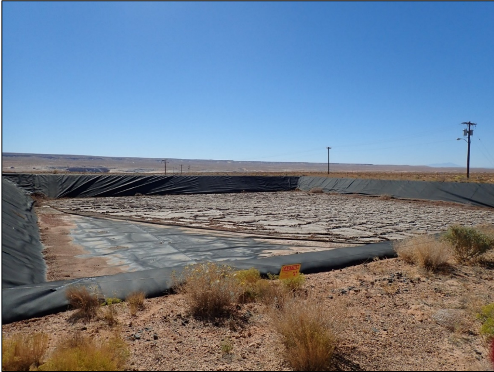
PL-9. Inactive, Lined Evaporation Pond
