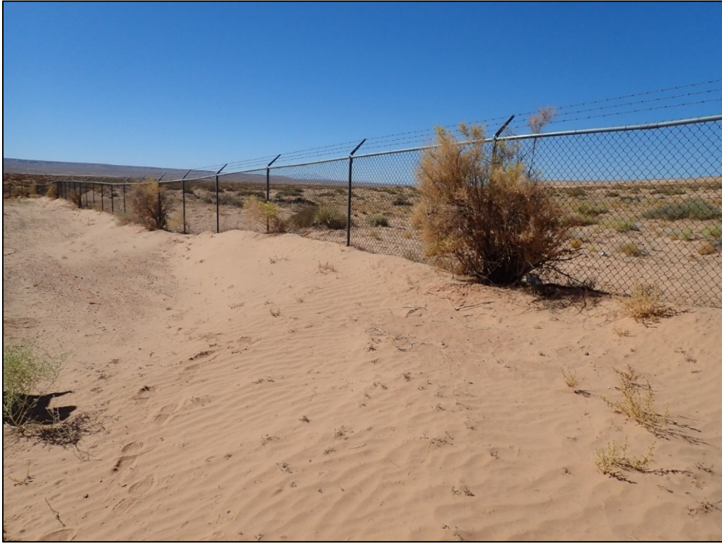
PL-1. Sand Accumulation and Treated Woody Vegetation Along West Fence
