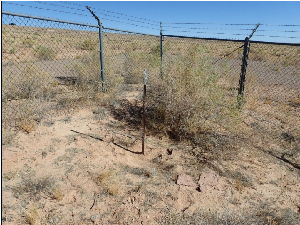
PL-6. Survey/Boundary Monument SM/BM-3 with Sand Accumulation
