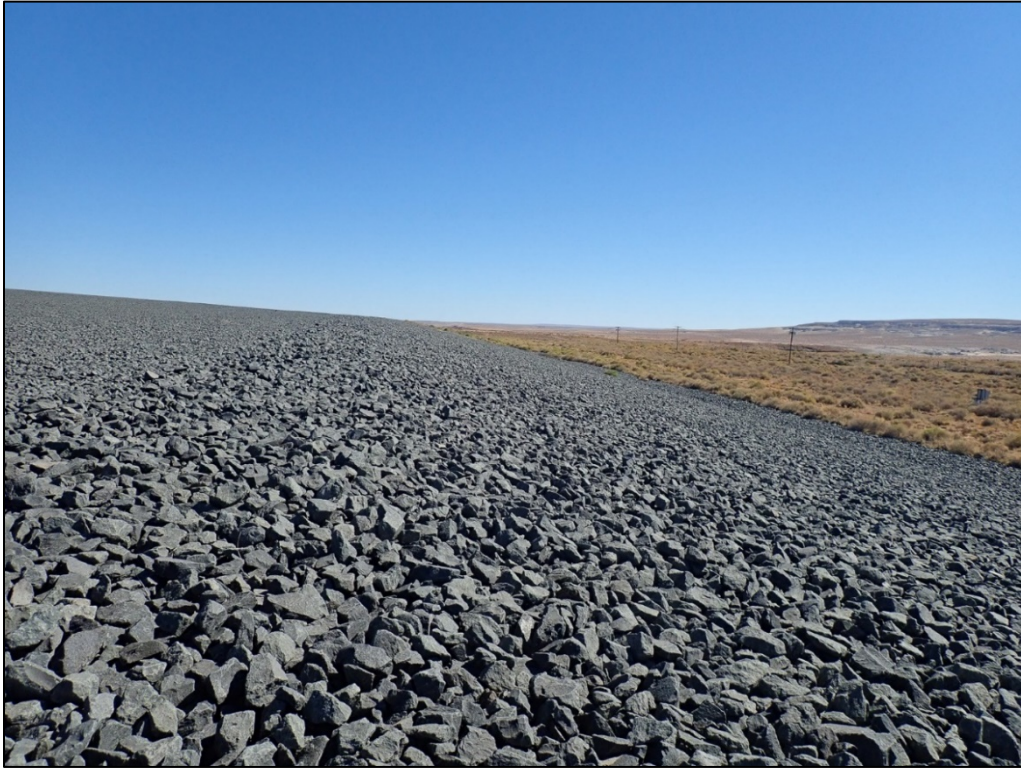
PL-7. Disposal Cell Top and Side Slope
