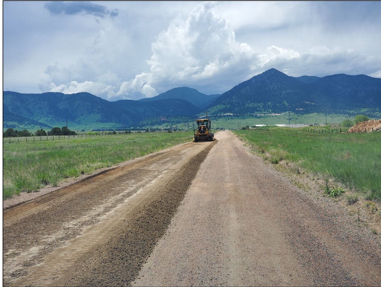
2023 Roads Maintenance Project
