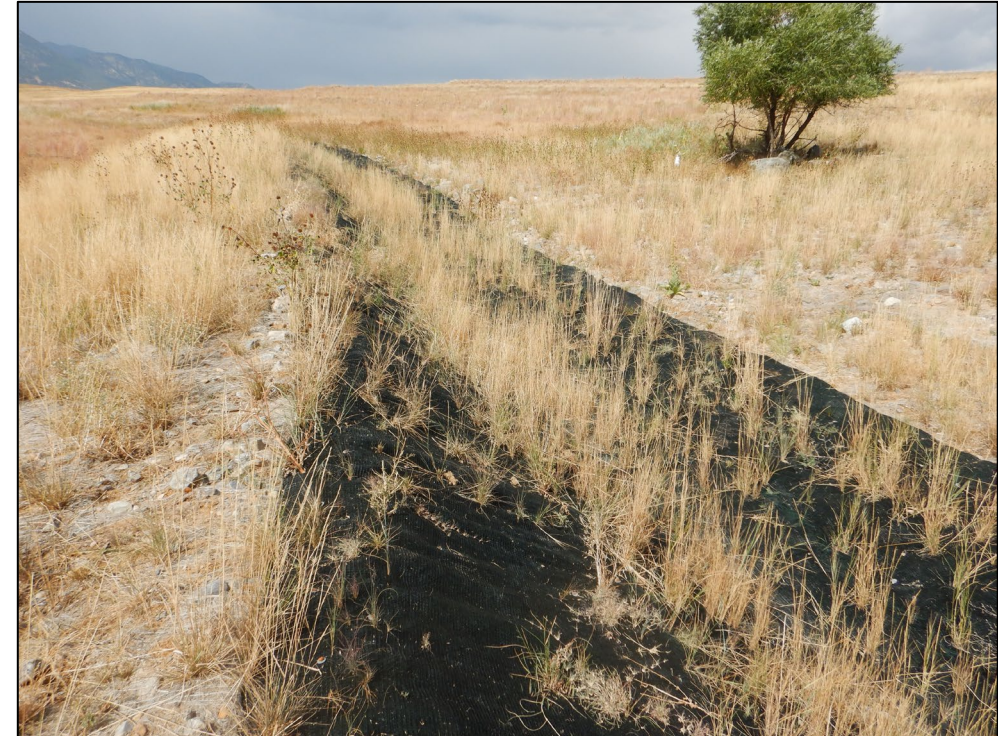
OLF Berm Seven with turf reinforcement material
