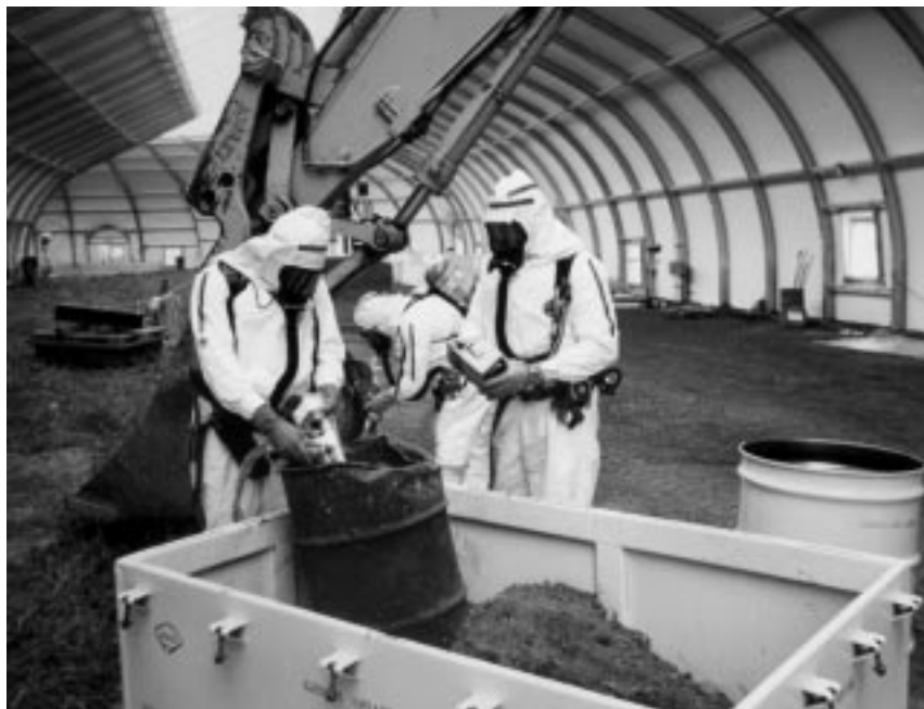
Figure 1.4: Remediation Activities at One of Rocky Flats' Contaminated Environmental Sites
