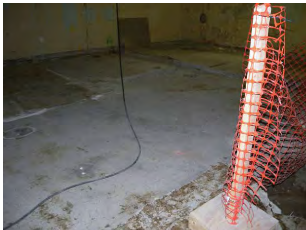
Figure C-29. T Bldg. Room 63 View J
