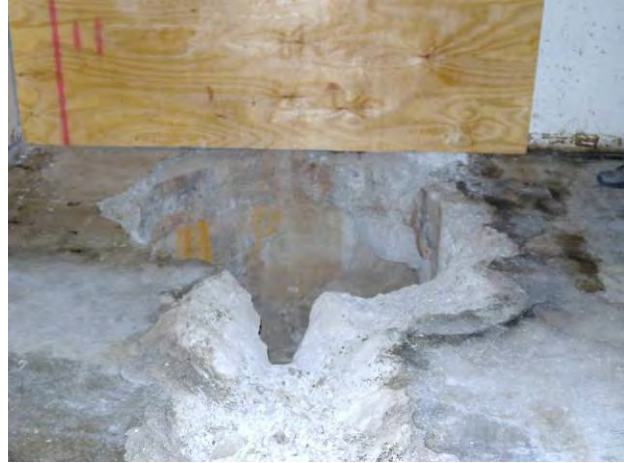
Figure C-5. T Bldg. Room 16 View D
