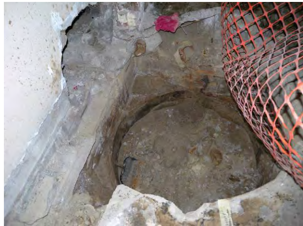
Figure C-27. T Bldg. Room 63 View H
