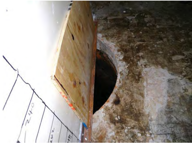
Figure C-19. T Bldg. Room 61 View H
