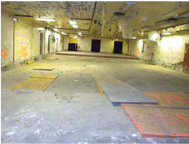
Figure C-44. T Bldg. Rooms 39-44, 48-50 View G
