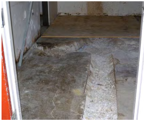
Figure C-2. T Bldg. Room 16 View A
