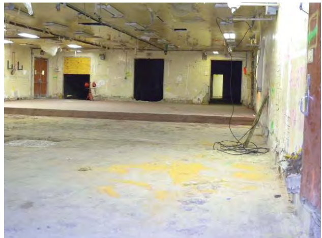
Figure C-47. T Bldg. Rooms 39-44, 48-50 View L
