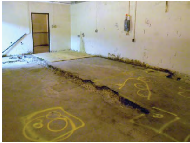
Figure C-11. T Bldg. Room 16 View J
