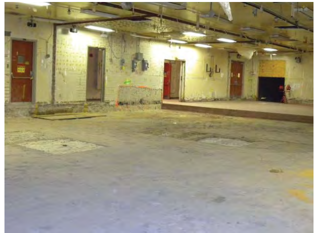
Figure C-45. T Bldg. Rooms 39-44, 48-50 View H
