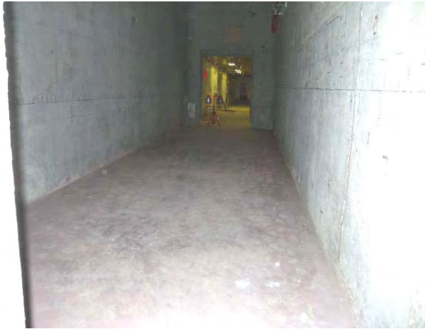
Figure C-36. T Bldg. Room 59 View E
