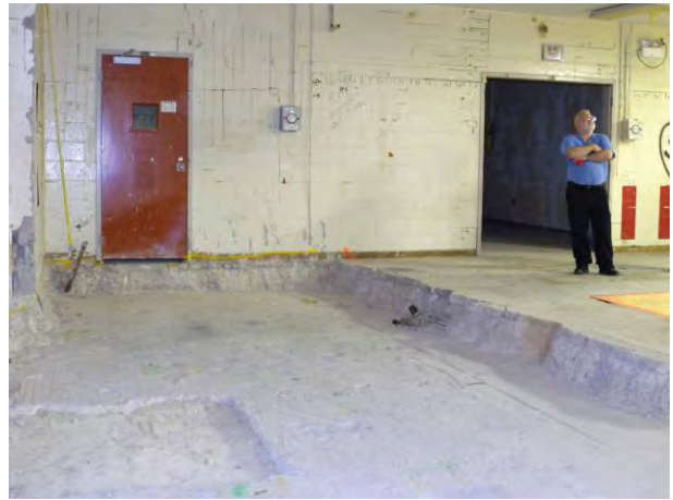
Figure C-43. T Bldg. Rooms 39-44, 48-50 View F
