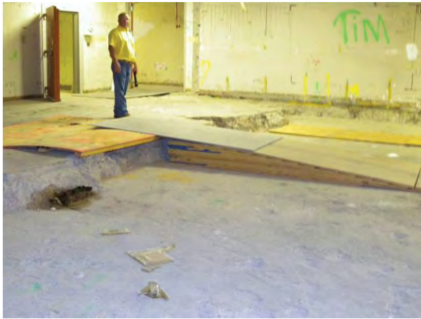
Figure C-42. T Bldg. Rooms 39-44, 48-50 View E
