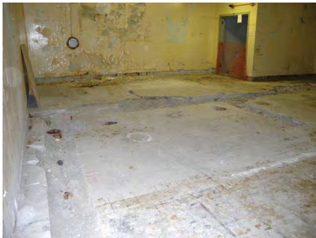
Figure C-22. T Bldg. Room 63 View C
