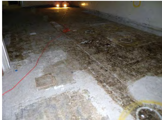
Figure C-15. T Bldg. Room 61 View D
