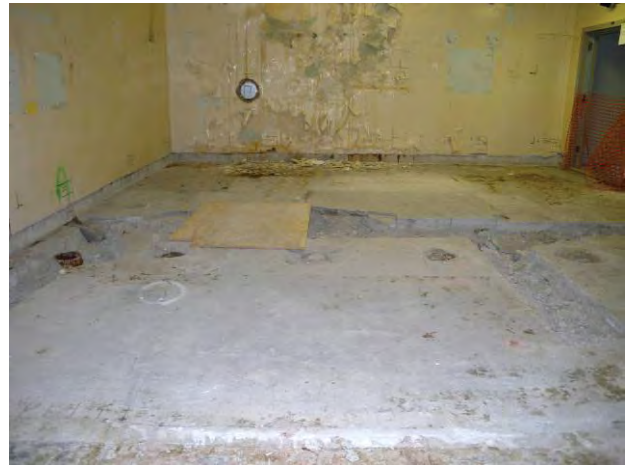
Figure C-21. T Bldg. Room 63 View B
