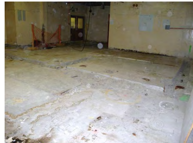
Figure C-23. T Bldg. Room 63 View D
