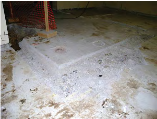
Figure C-26. T Bldg. Room 63 View G
