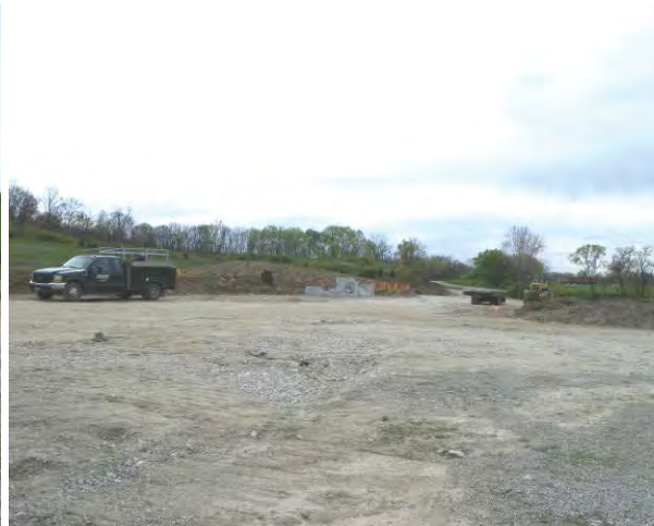
Figure 19. Work on Spine Road, Looking Southeast from Trailer 1 in OU-1 Area
