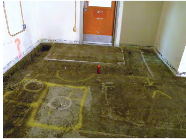
Figure C-17. T Bldg. Room 61 View F
