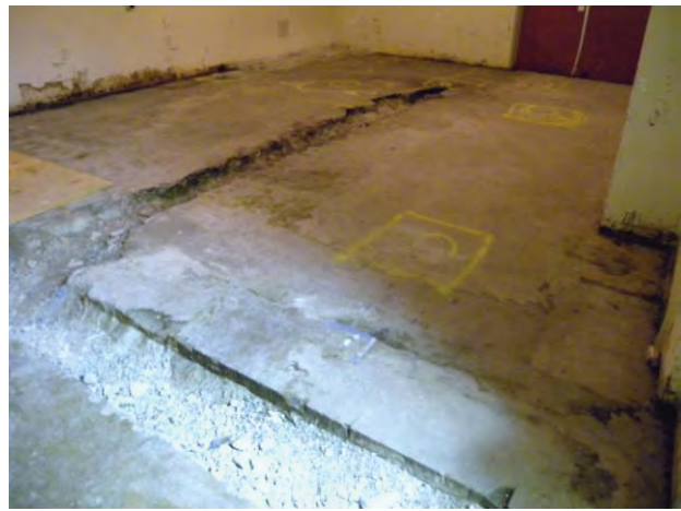
Figure C-3. T Bldg. Room 16 View B
