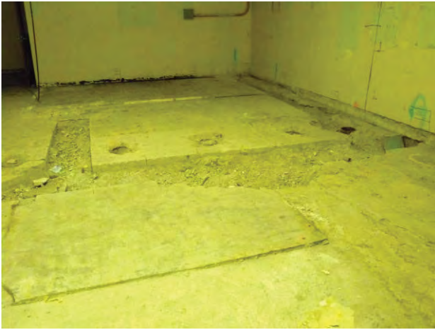
Figure C-24. T Bldg. Room 63 View E
