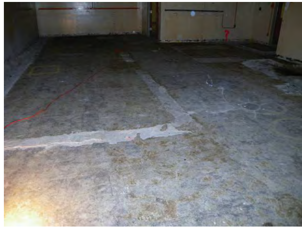
Figure C-13. T Bldg. Room 61 View B
