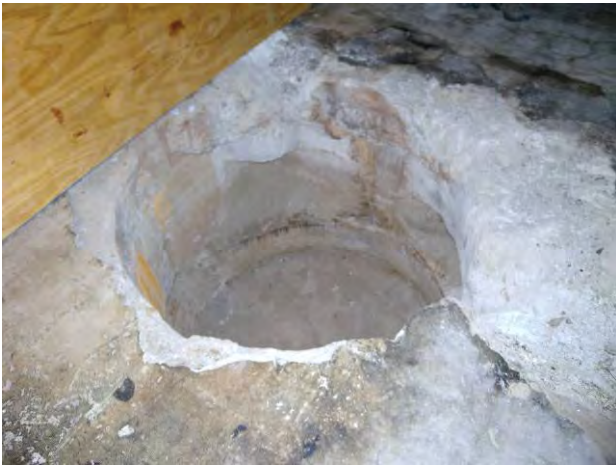
Figure C-6. T Bldg. Room 16 View E
