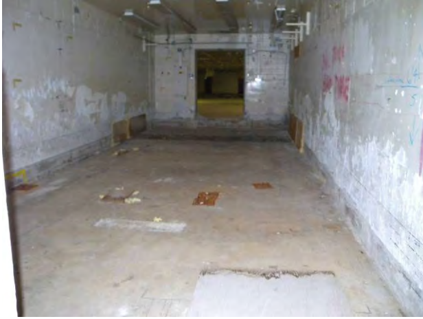
Figure C-34. T Bldg. Room 58 View C
