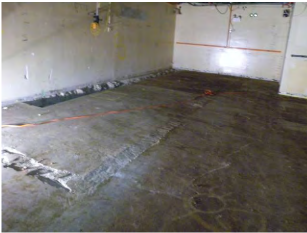
Figure C-12. T Bldg. Room 61 View A
