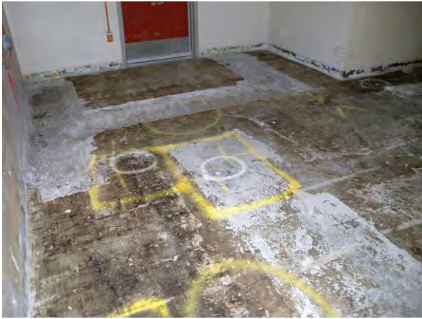
Figure C-16. T Bldg. Room 61 View E
