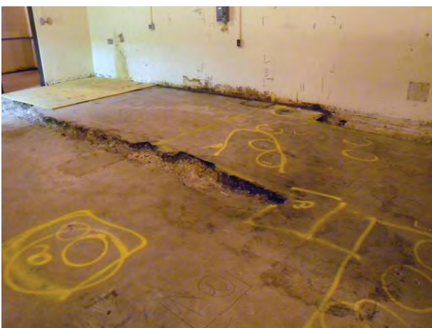
Figure C-10. T Bldg. Room 16 View I
