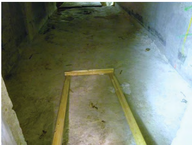
Figure C-32. T Bldg. Room 57 View A
