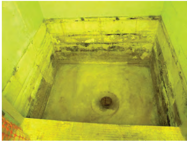
Figure C-31. T Bldg. Room 62 View M
