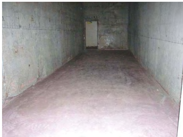
Figure C-37. T Bldg. Room 59 View F
