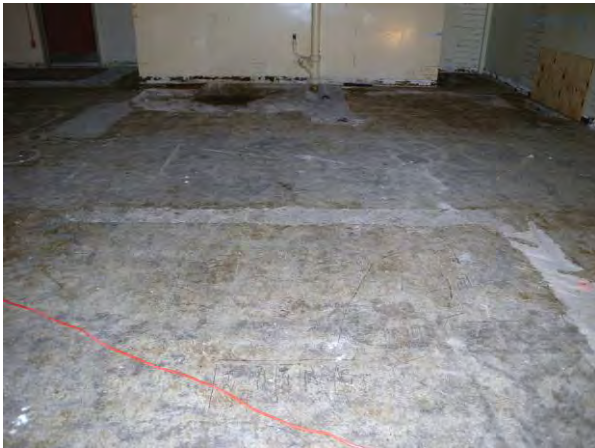
Figure C-14. T Bldg. Room 61 View C
