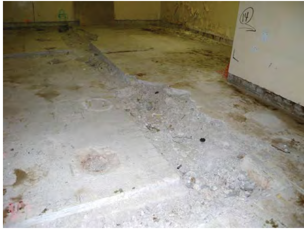
Figure C-25. T Bldg. Room 63 View F
