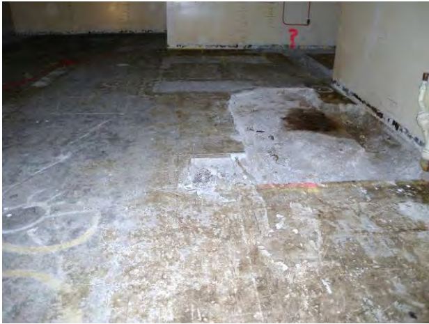
Figure C-18. T Bldg. Room 61 View G
