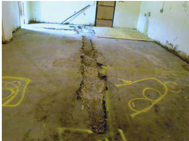
Figure C-9. Room 16 View H
