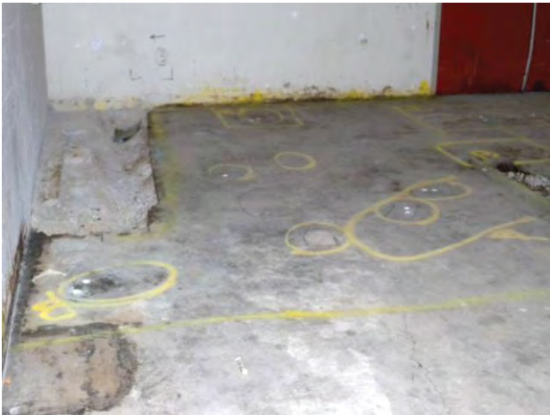
Figure C-8. T Bldg. Room 16 View G
