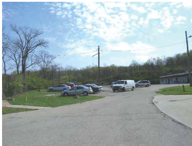
Figure 8. Parking Area That Replaced Buildings 2, 63, and 63W
