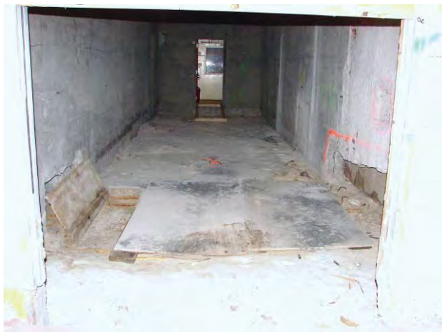
Figure C-33. T Bldg. Room 57 View B
