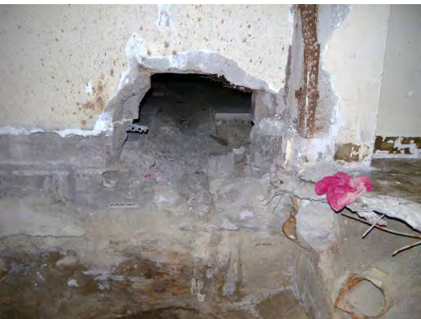
Figure C-28. T Bldg. Room 63 View I
