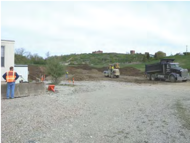
Figure 18. Work on Spine Road, Looking North Toward OU-1 Area
