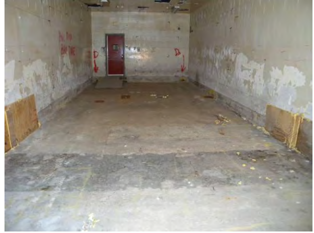
Figure C-35. T Bldg. Room 58 View D
