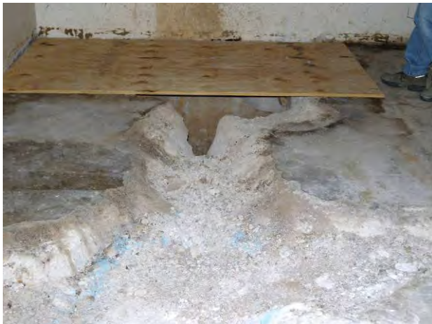
Figure C-4. T Bldg. Room 16 View C
