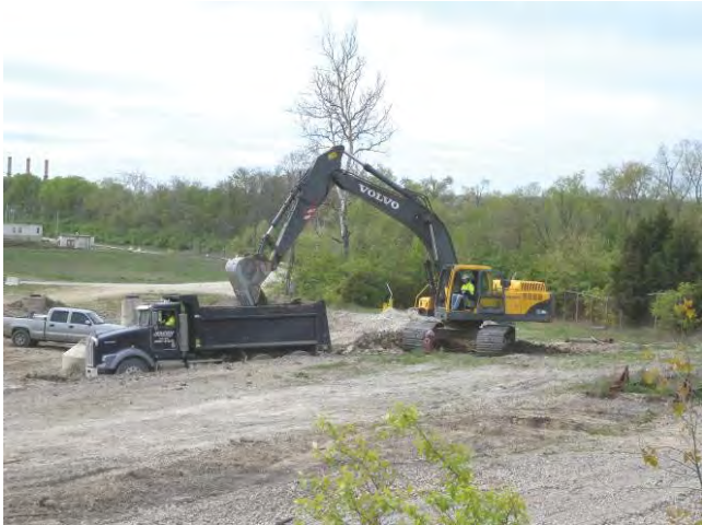
Figure 16. Work on Spine Road, Looking South Toward Wells 0315 and 0347
