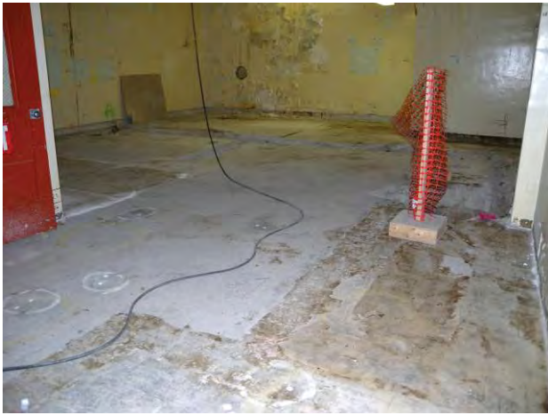
Figure C-20. T Bldg. Room 63 View A
