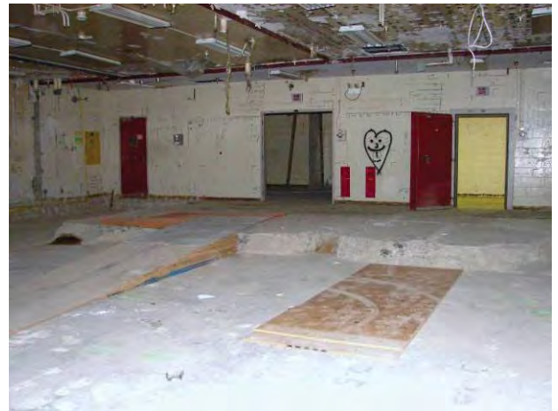
Figure C-41. T Bldg. Rooms 39-44, 48-50 View D
