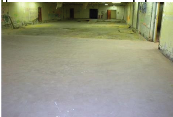
Figure C-38. T Bldg. Rooms 39-44, 48-50 View A
