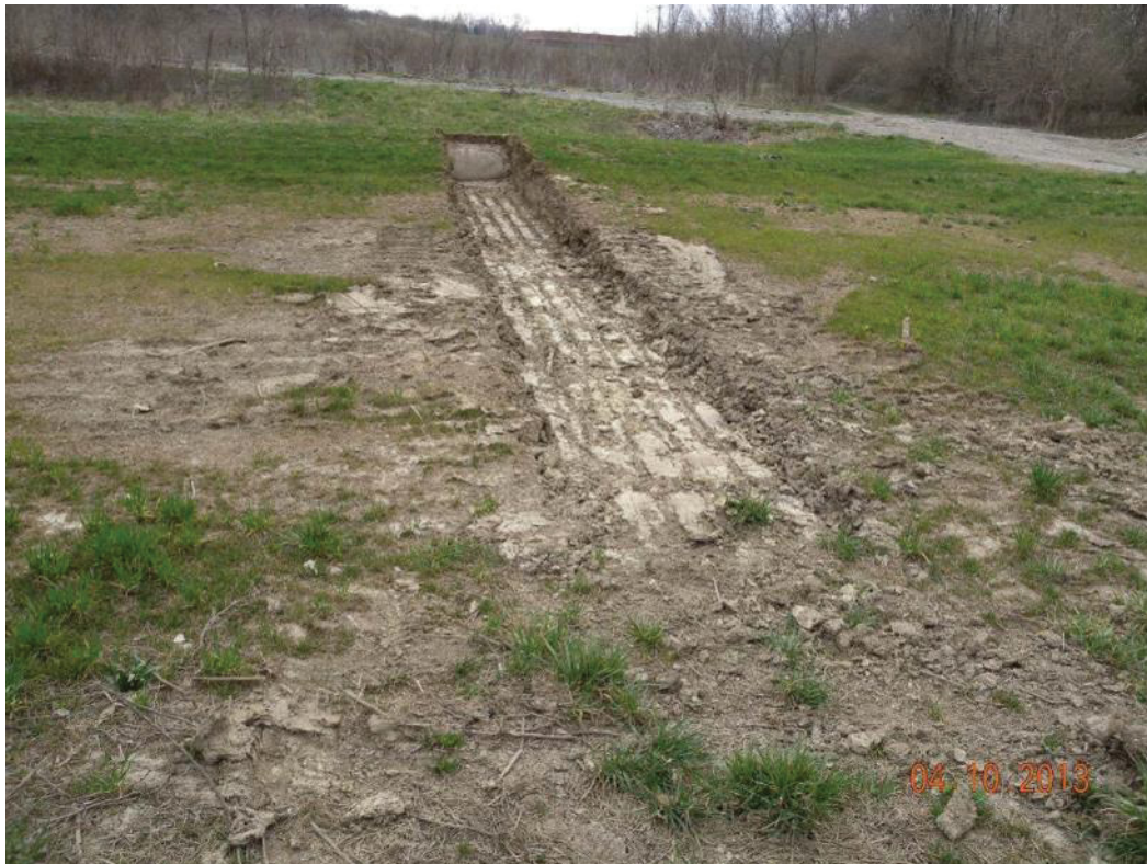
Figure 12. French Drain Installation Southward from Well P046 in OU-1 Area
