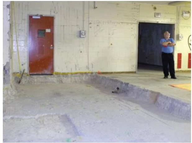
Figure C-43. T Bldg. Rooms 39-44, 48-50 View F
