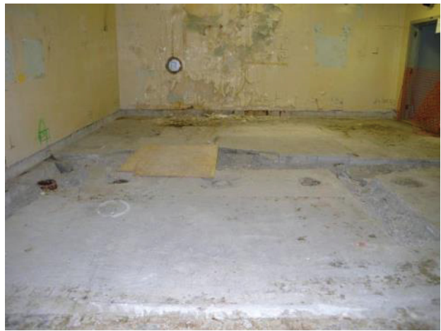
Figure C-21. T Bldg. Room 63 View B
