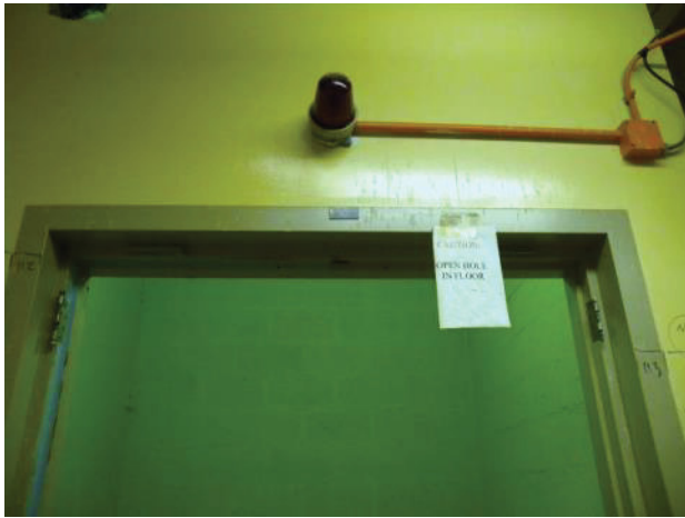
Figure C-30. T Bldg. Room 62 View K
