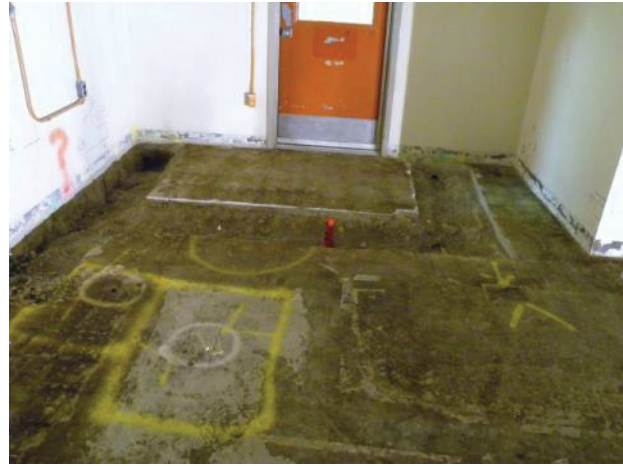
Figure C-17. T Bldg. Room 61 View F
