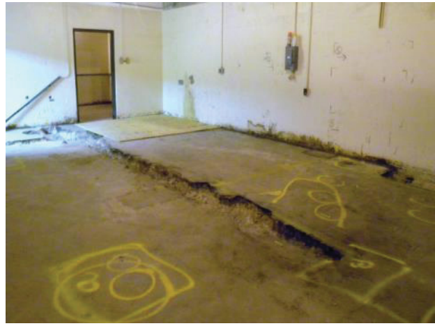
Figure C-11. T Bldg. Room 16 View J
