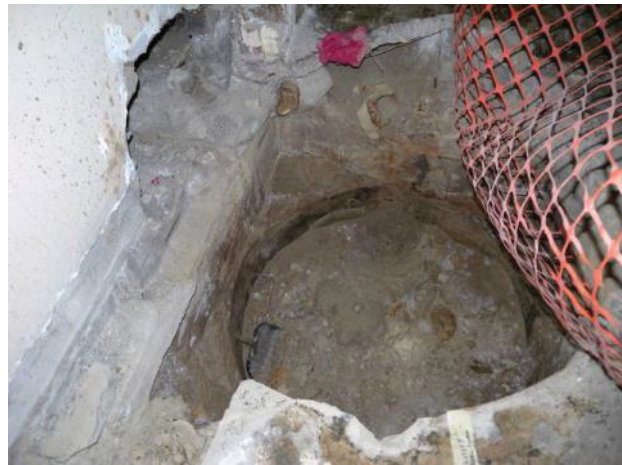
Figure C-27. T Bldg. Room 63 View H
