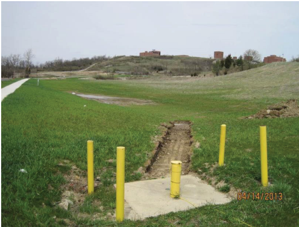
Figure 14. French Drain Being Installed in OU-1 Area to Correct Drainage Problem
