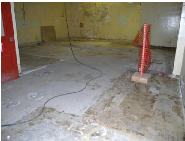
Figure C-20. T Bldg. Room 63 View A
