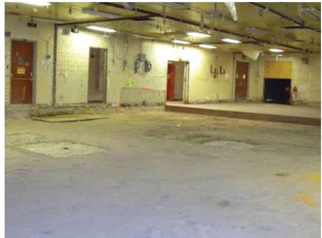
Figure C-45. T Bldg. Rooms 39-44, 48-50 View H
