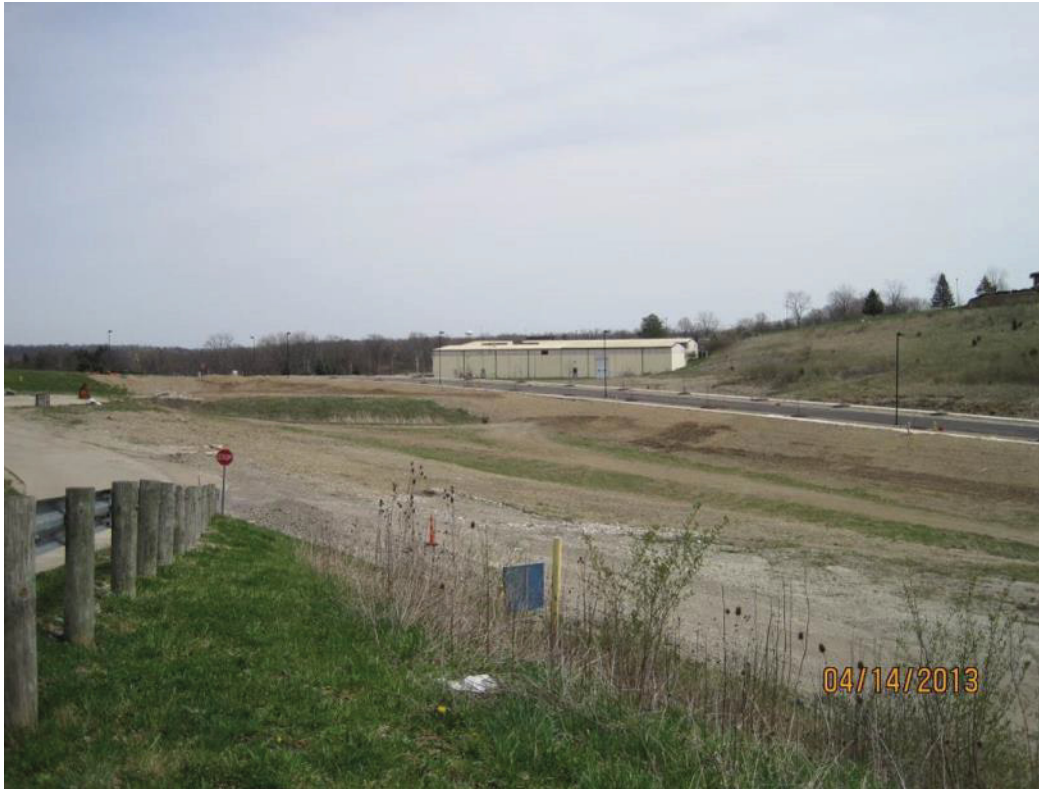
Figure 7. Vanguard Blvd. Looking Northeast Toward Building 61
