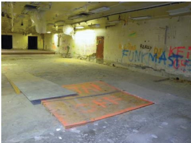
Figure C-46. T Bldg. Rooms 39-44, 48-50 View I
