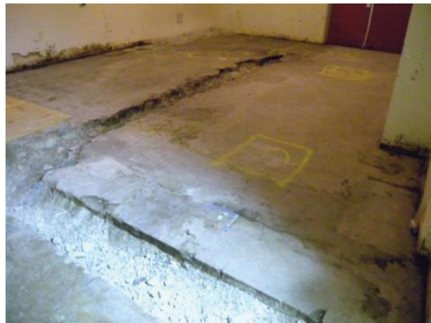
Figure C-3. T Bldg. Room 16 View B
