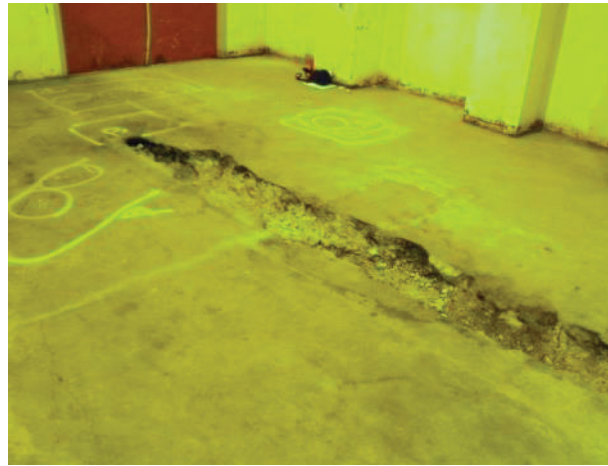
Figure C-7. T Bldg. Room 16 View F
