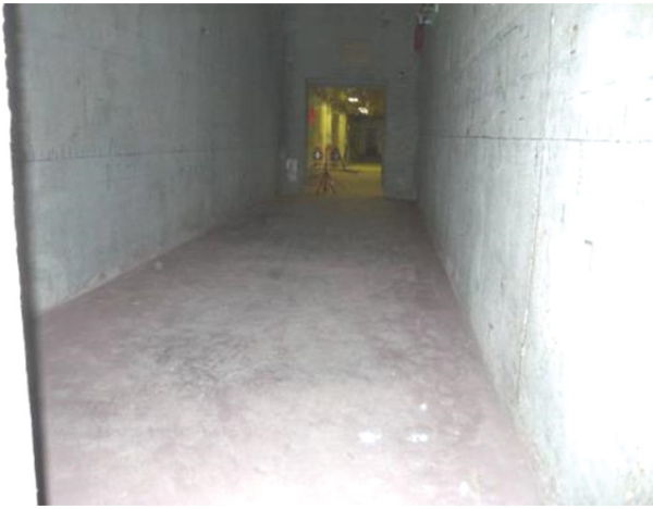
Figure C-36. T Bldg. Room 59 View E
