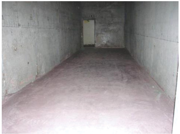
Figure C-37. T Bldg. Room 59 View F
