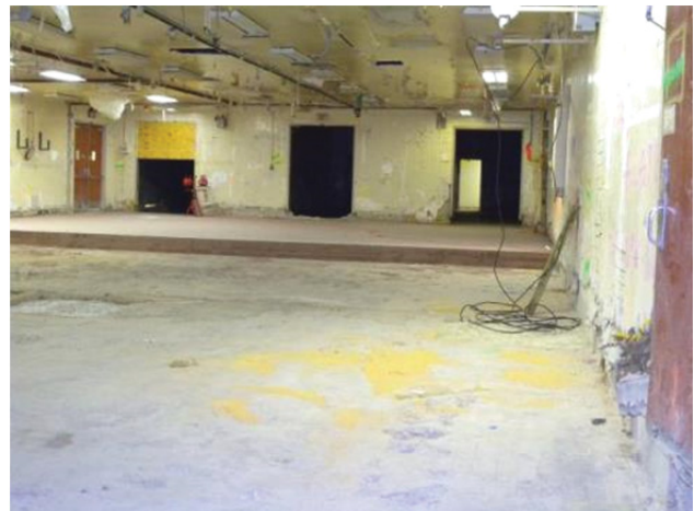
Figure C-47. T Bldg. Rooms 39-44, 48-50 View J
