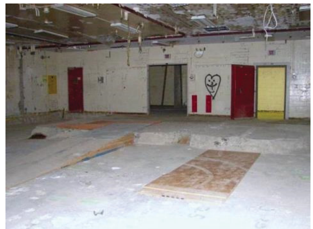
Figure C-41. T Bldg. Rooms 39-44, 48-50 View D
