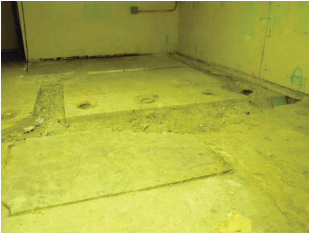
Figure C-24. T Bldg. Room 63 View E
