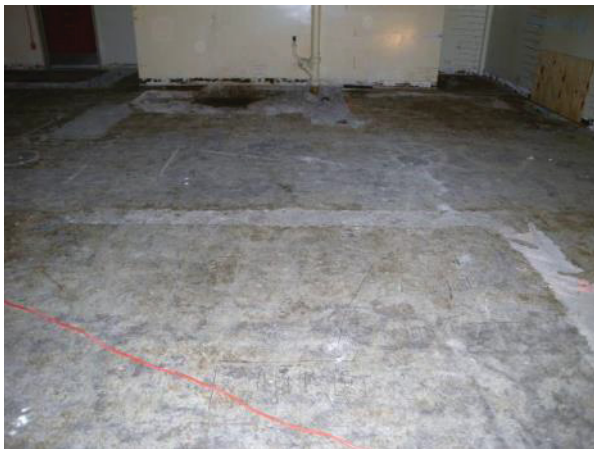
Figure C-14. T Bldg. Room 61 View C
