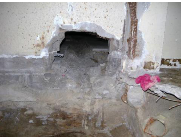
Figure C-28. T Bldg. Room 63 View I
