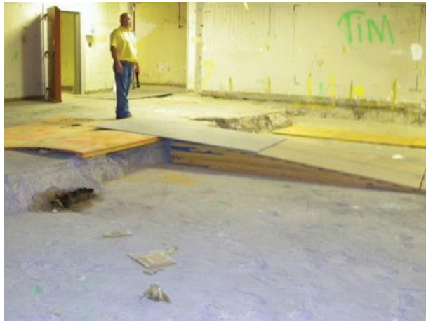
Figure C-42. T Bldg. Rooms 39-44, 48-50 View E
