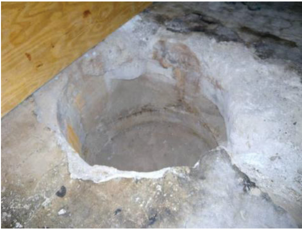
Figure C-6. T Bldg. Room 16 View E
