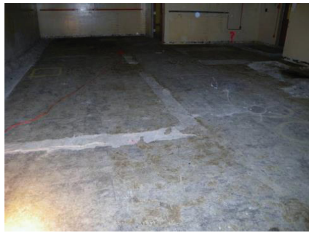
Figure C-13. T Bldg. Room 61 View B
