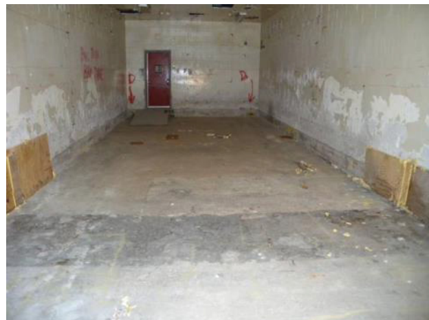
Figure C-35. T Bldg. Room 58 View D
