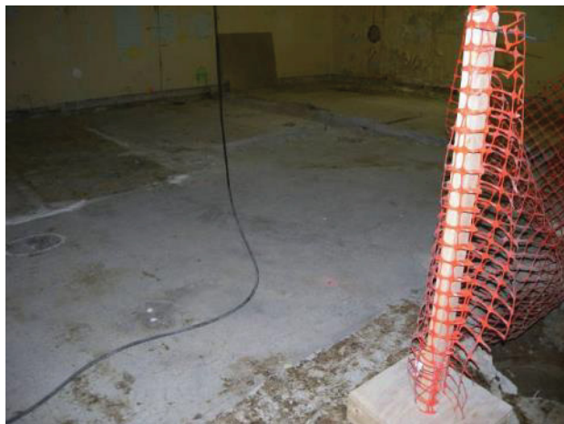
Figure C-29. T Bldg. Room 63 View J
