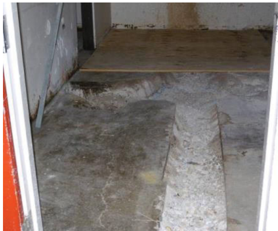
Figure C-2. T Bldg. Room 16 View A
