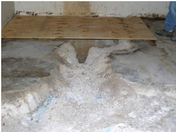
Figure C-4. T Bldg. Room 16 View C
