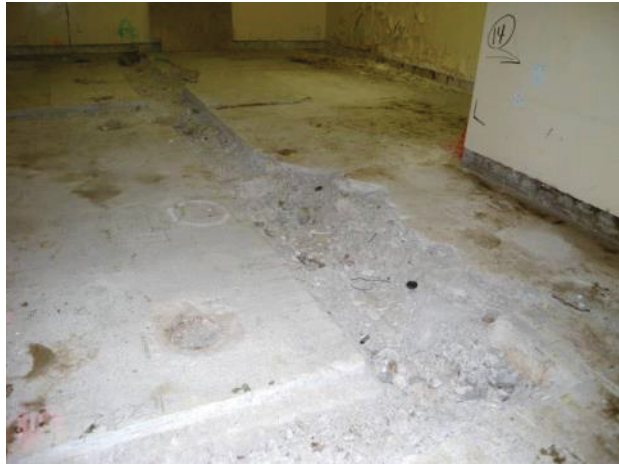
Figure C-25. T Bldg. Room 63 View F
