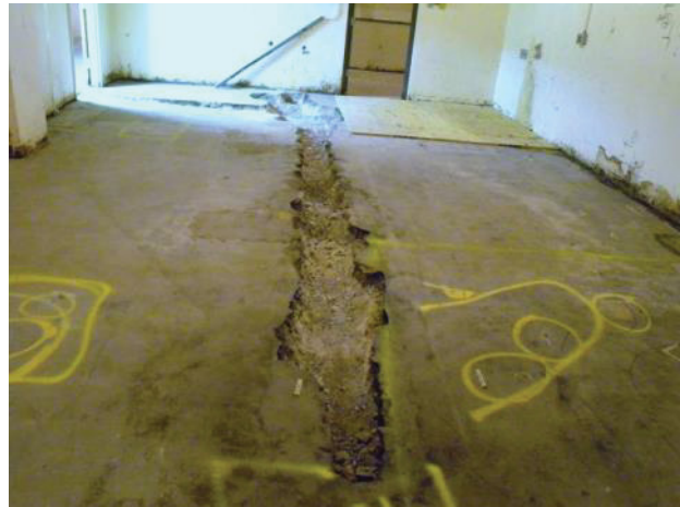
Figure C-9. Room 16 View H
