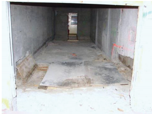
Figure C-33. T Bldg. Room 57 View B
