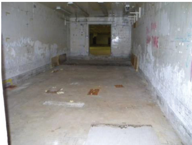
Figure C-34. T Bldg. Room 58 View C
