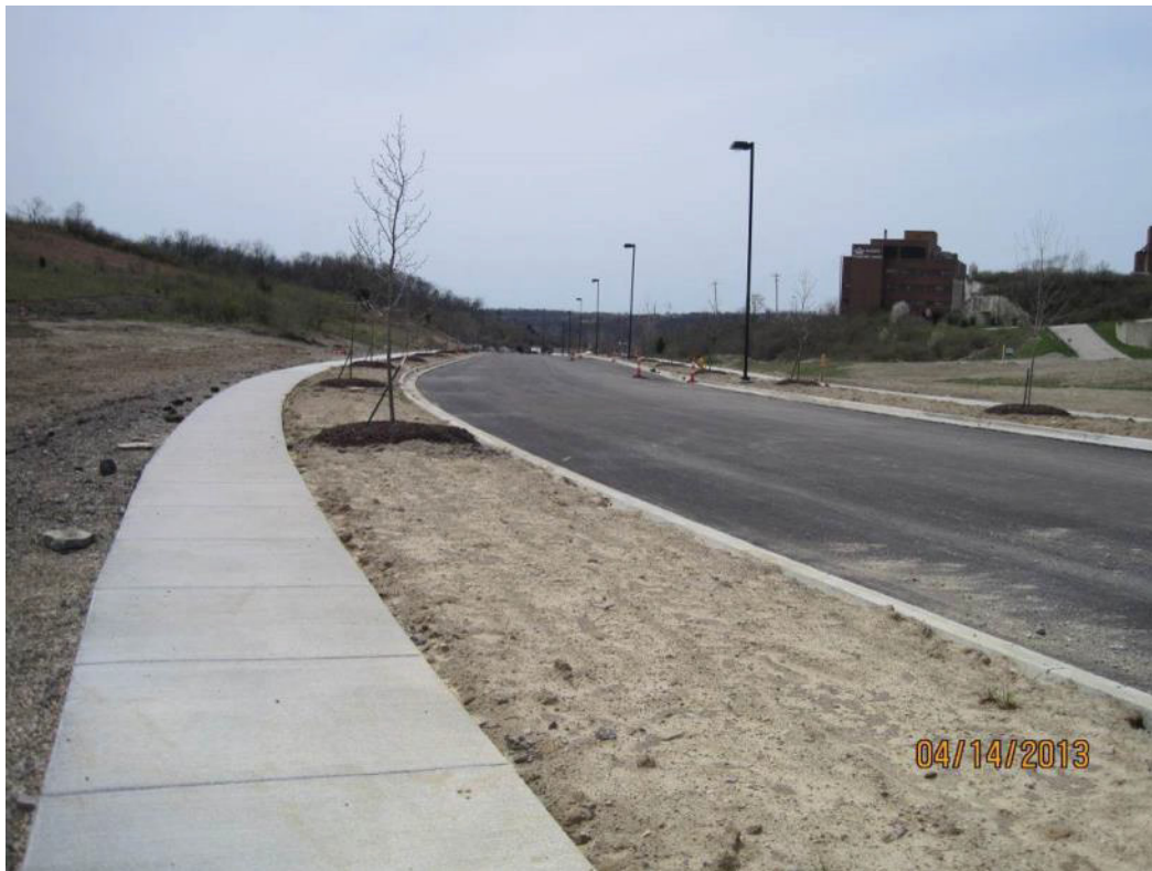
Figure 8. Vanguard Blvd. Looking Southwest Toward Central Office Space (COS) Building
