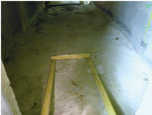
Figure C-32. T Bldg. Room 57 View A
