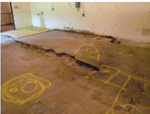
Figure C-10. T Bldg. Room 16 View I
