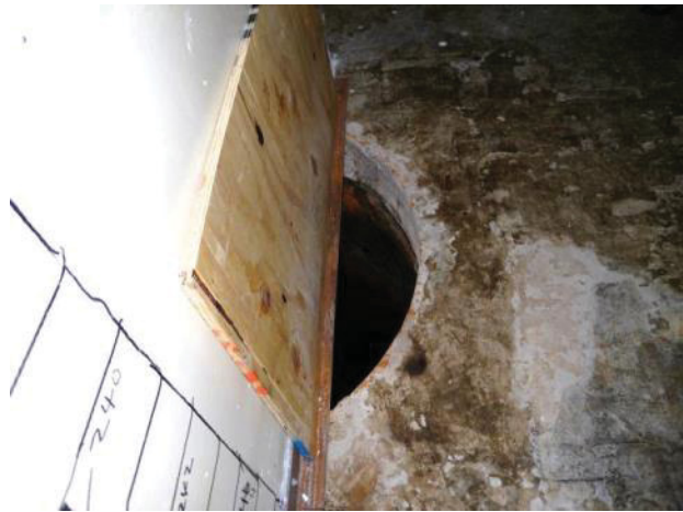
Figure C-19. T Bldg. Room 61 View H
